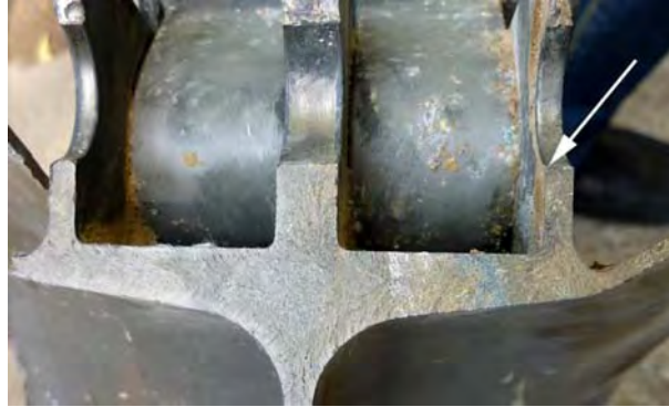
The arrow shows the place of a fatigue crack initiation on LP compressor 2 nd stage disk
