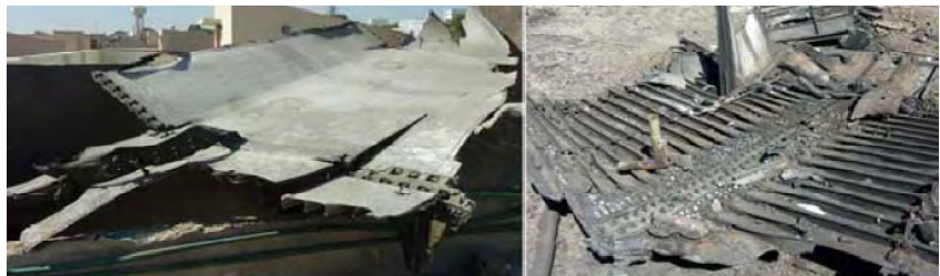
#20. Centre wing section upper and lower panels from the middle to the rear spar
