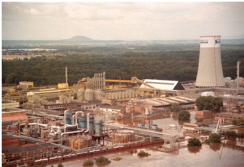
Figure 5.2: A flooded chemical factory. © Greenpeace/Vaclav Vasku
