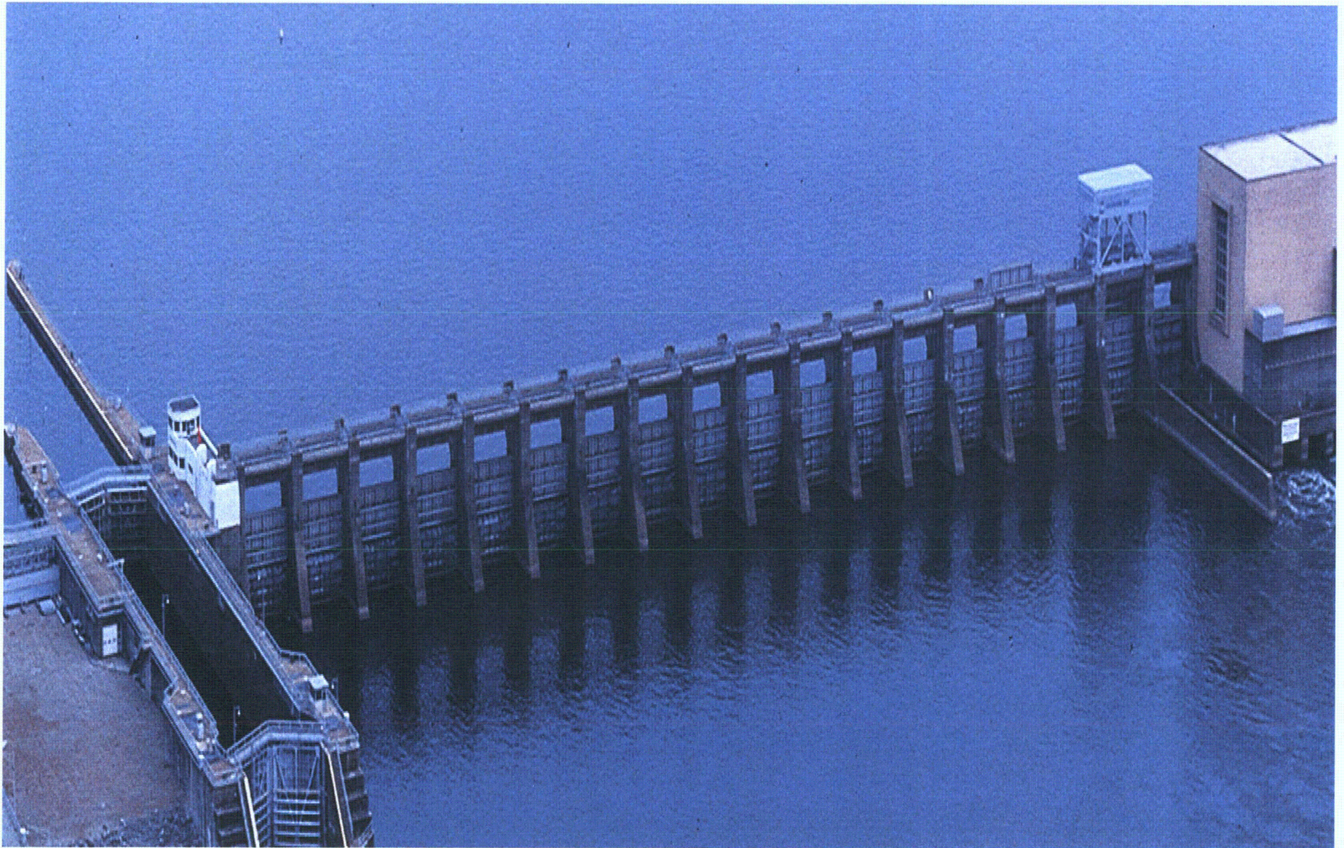
FIGURE 11 - View of Spillway Gates (looking upstream), September 1999
