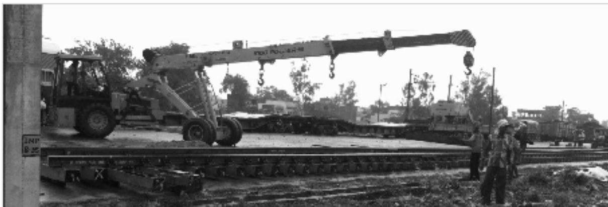
Using Hydra for collecting released PSC sleepers
