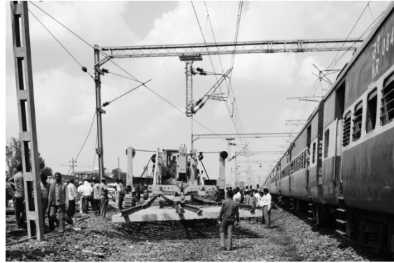
T-28 Machine laying 1:12 turnouts on PSC sleepers
