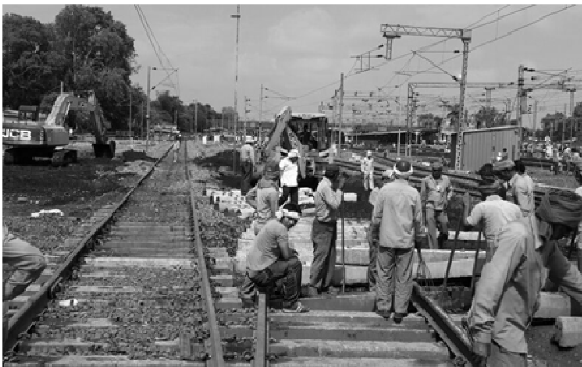
Manpower and Machines engaged in restoration going on war-footing
