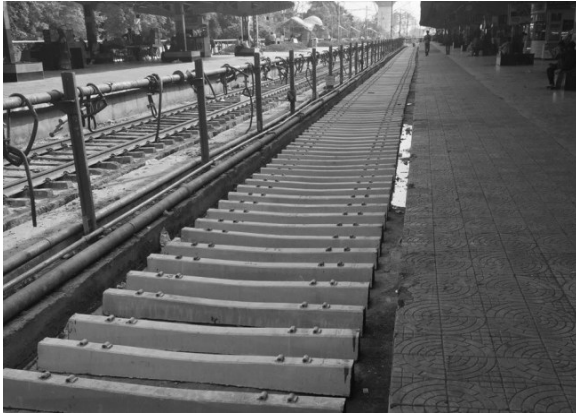
Sleepers spread out for concrete apron on Platform No. 5
