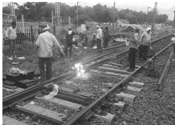
Alumino Thermic Welding of all track joints
