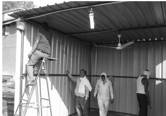
Goomties with unserviceable PSC sleeper flooring
