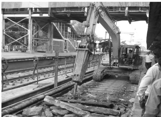
Dismantling of track on existing concrete apron
