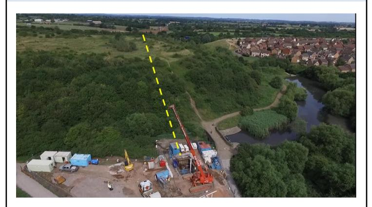
We have successfully tunnelled beneath the M4. Tunnelling has taken place from the Three Brooks Local Nature Reserve in Bradley Stoke, with great care being taken to protect wildlife and preserve natural habitats. The total length of the tunnel is approximately 400m and the DN is 1800.
