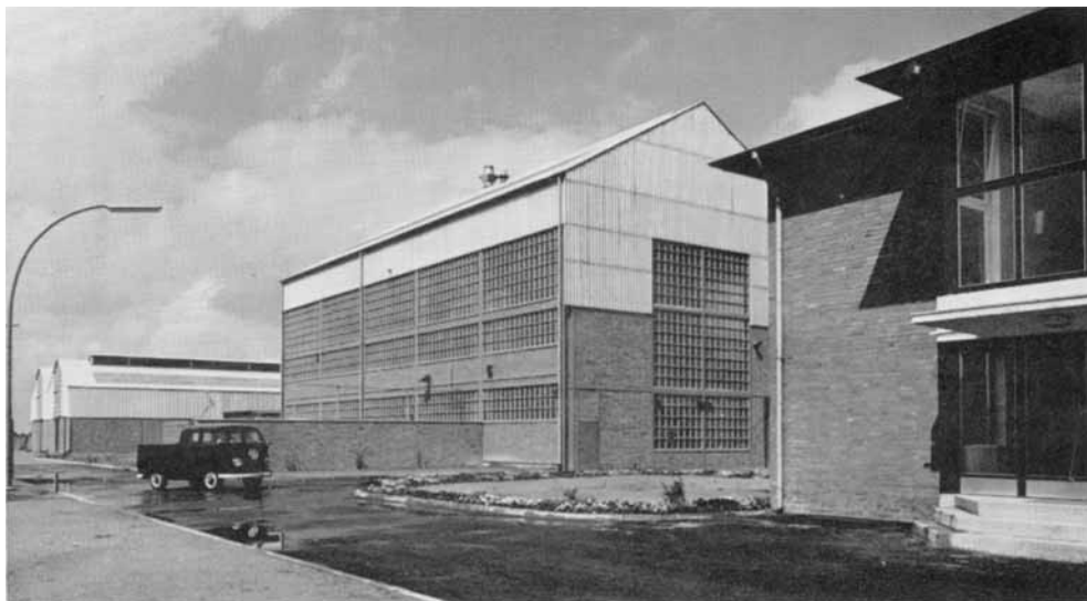
Production of platinum-on-alumina catalyst for European licensees of the Platforming process was begun in England in 1953 by Universal-Matthey Products Ltd. Local demand has been met by the construction of this new plant in Cologne, operated by Universal-Matthey Products (Deutschland) GmbH.
