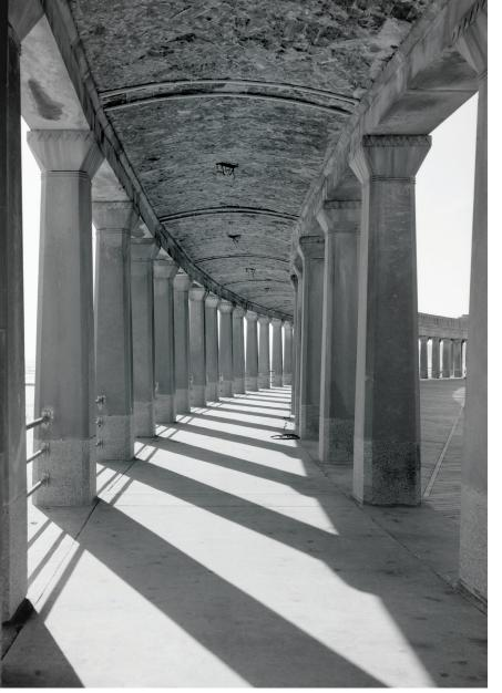
The side of the building that faces the ocean is fronted by a portico consisting of two rows, curved in plan, of concrete columns.
