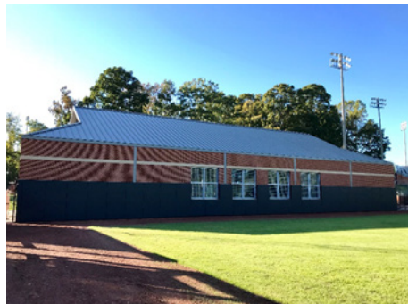
Baseball Indoor Training Facility (Side)
