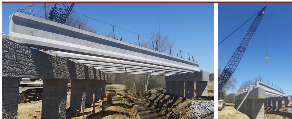
Phillips Road Realignment construction
