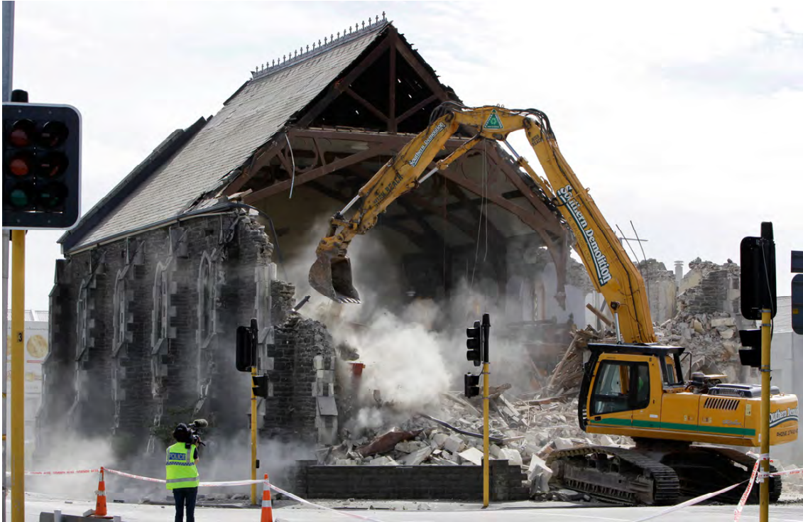
Canterbury Provincial Council Chamber under demolition 2011
