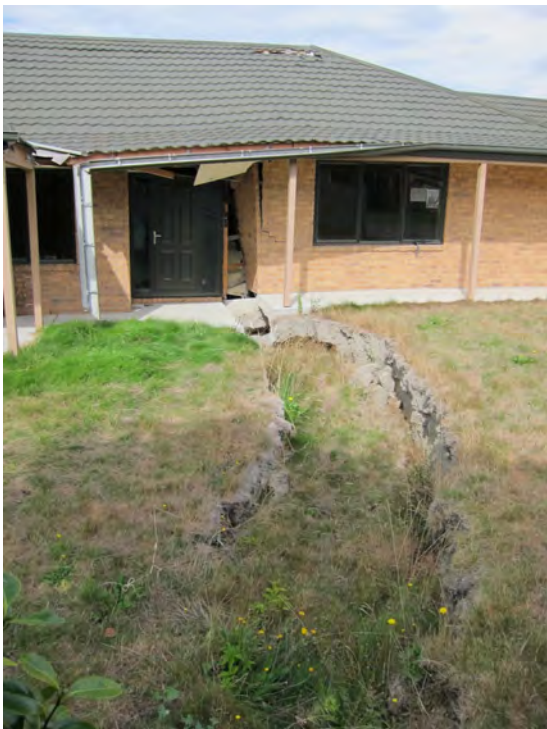
Liquefaction damage in Kaiapoi
