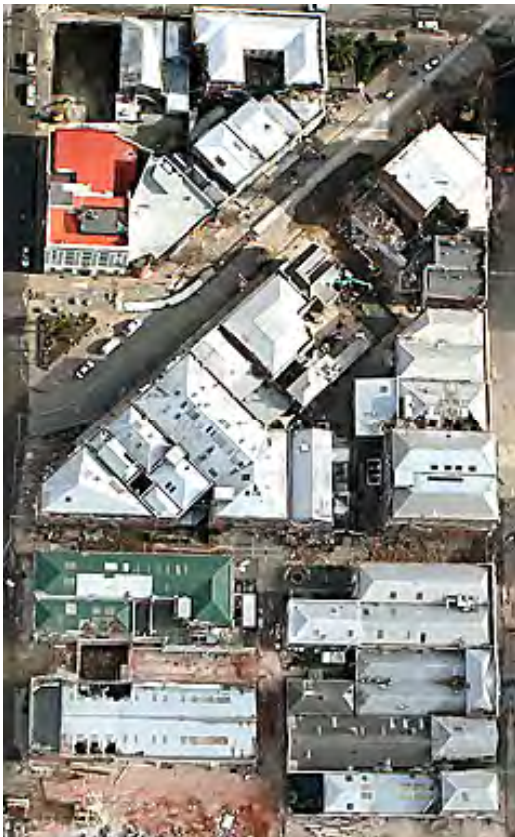
DAMAGED: Poplar Street from the air July 2011
