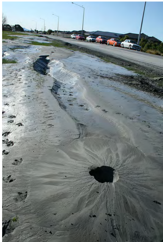
Sand boil where water welled up through sand
