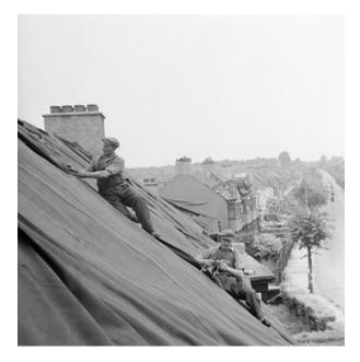
Roofers repairing bomb-damaged roofs with temporary tarpaulins. High explosive was capable of smashing windows and lifting roof tiles over a wide area, but most of the more than 2 million houses damaged in the Blitz were habitable again after a few weeks. (Courtesy of the Imperial War Museum)
