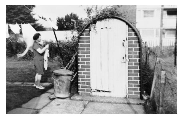
A garden shelter during the war. The Anderson shelter seen here, designed by the engineer David Anderson, was supposed to be installed below ground level, but in areas with the risk of flooding this was difficult to do. They were no defence against a direct or near direct hit. (Courtesy of the Imperial War Museum)
