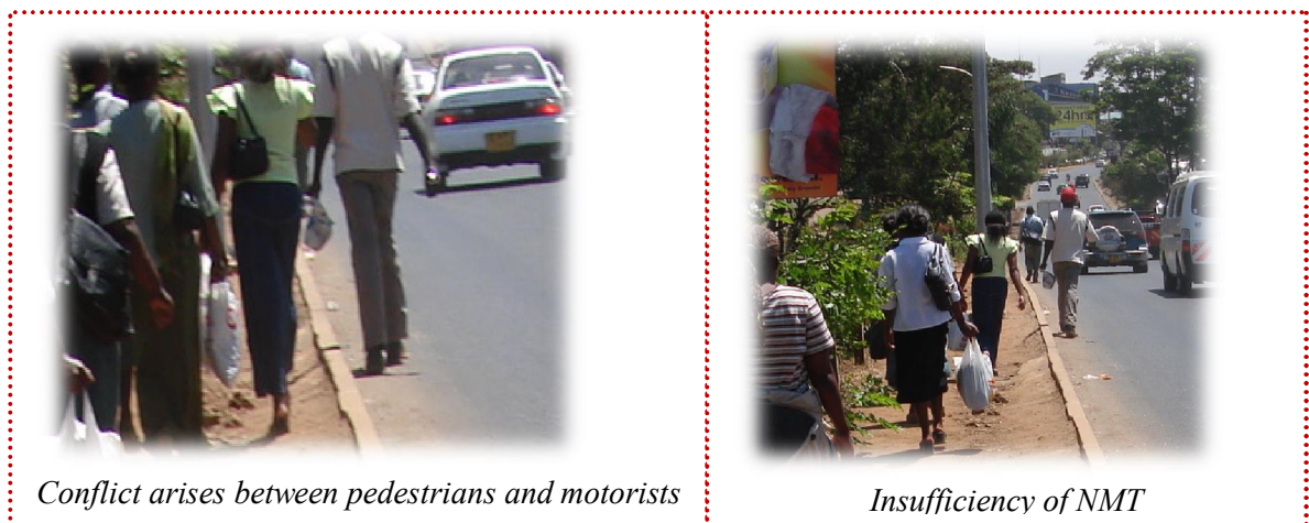
Plate 5.5: Inadequacy of sidewalks
