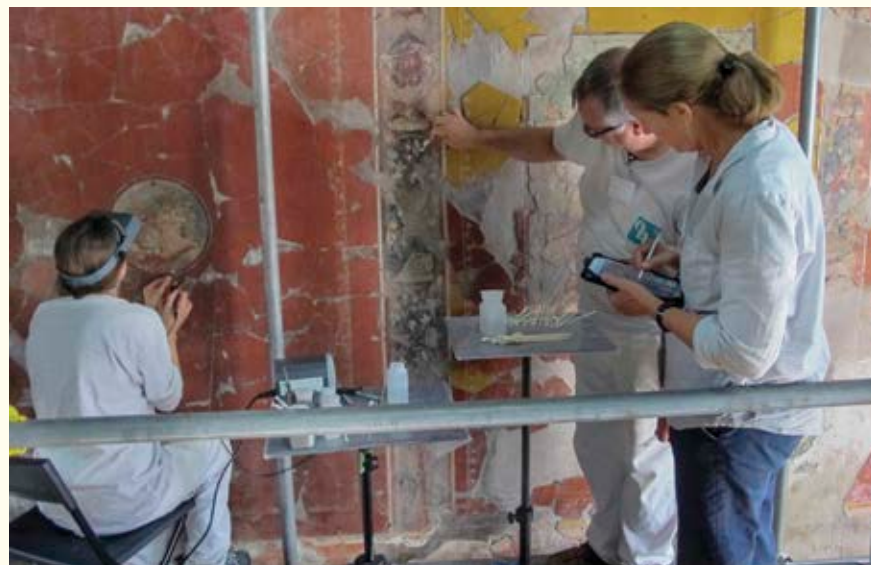
Members of the GCI project team carrying out monitoring and reattachment of flaking paint in the tablinum of the Casa del Bicentenario at Herculaneum. Photo: Franchesca Piqué
