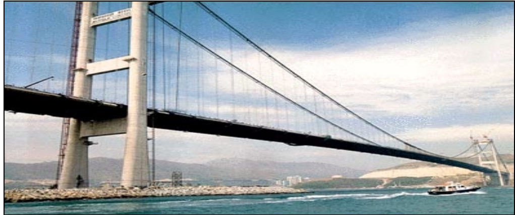
Figure 4.2. Tsing Ma Suspension Bridge
