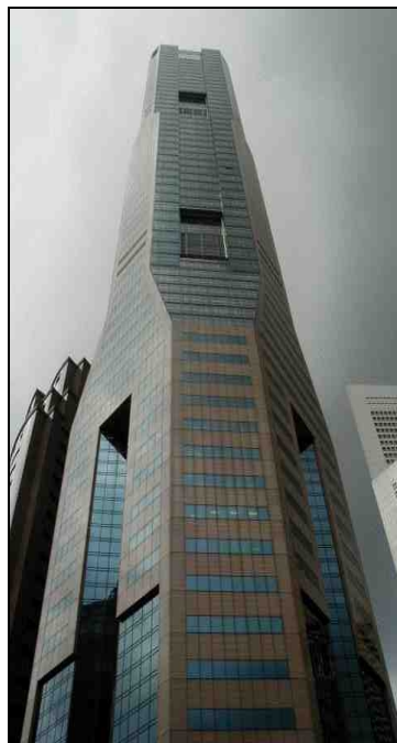
Figure 4.3. Republic Plaza Building (RPB)
