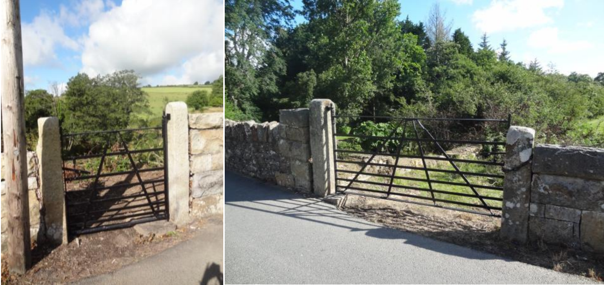
August 2013 - Our beautiful restored Antique Wrought Iron Gates.
