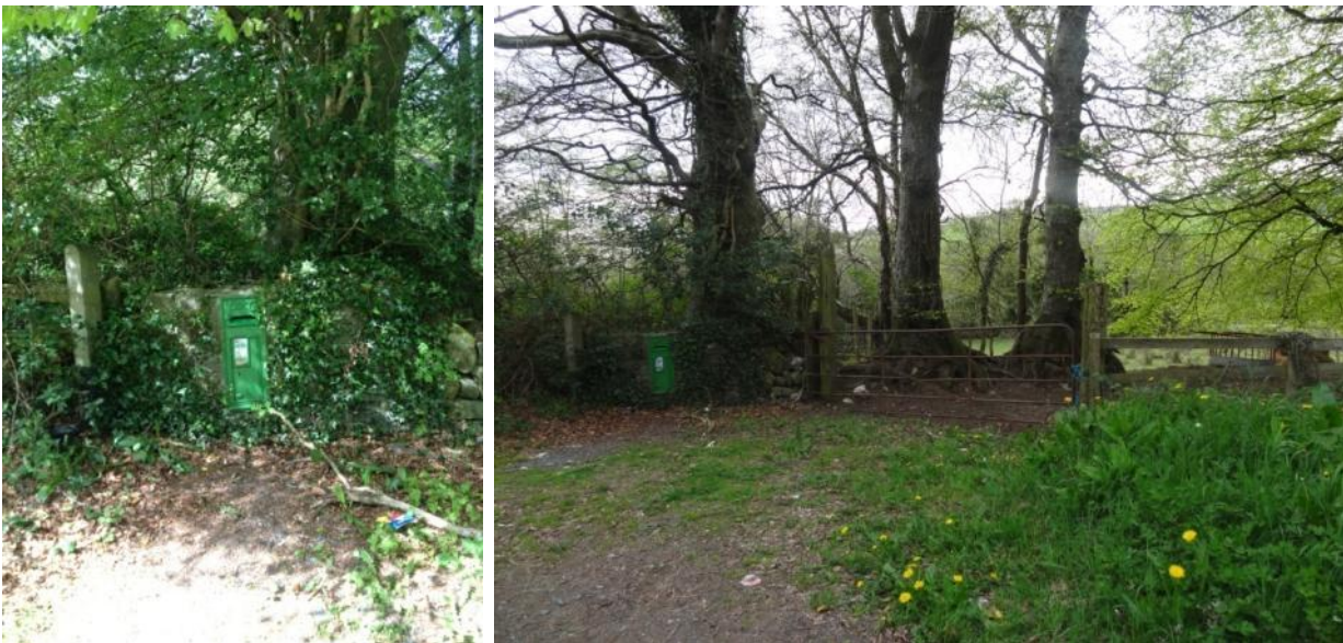
Pictured Left to right – The Post Box in Annacurra, the gate and fencing beside the postbox in need of replacement.
