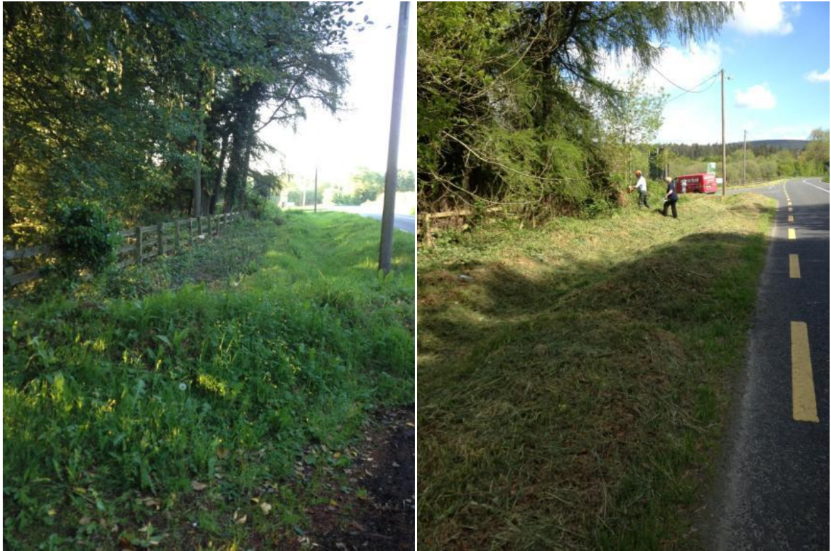
May 2013 – Clearing back the overgrowth at Annacurra Crossroads
