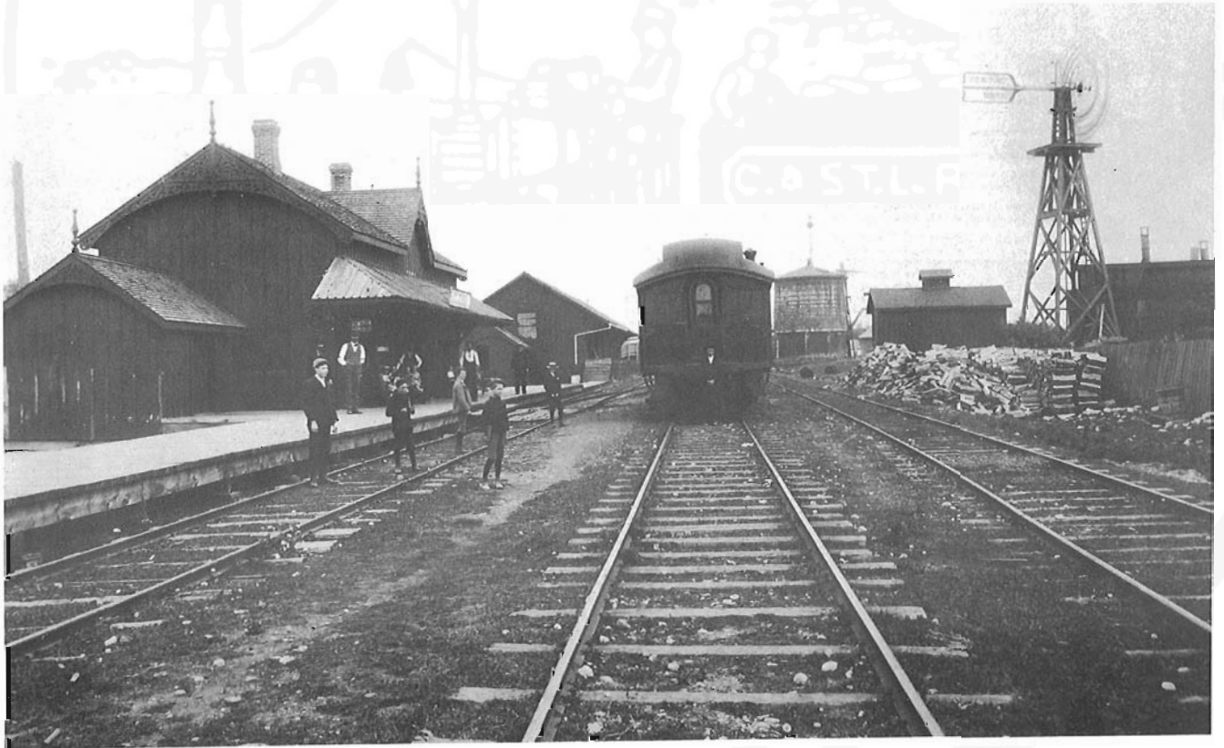
Canadian Pacific Railway station at Elora, Ontario photographed by J.W. Heckman on September 13, 1898. Note the loco house and the windmill to pump water into the tank. The coach was built by the Grand Trunk in the days when it controlled the TG&B. Canadian Pacific Corporate Archives, photo A-21030.
