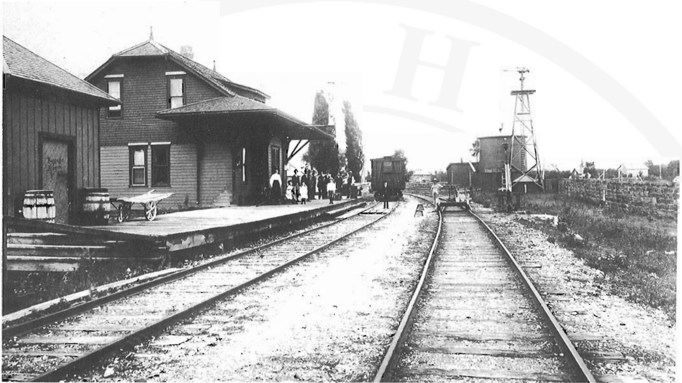
The CPR station at Wingham, Ontario was built in 1887. Here we see it as photographed by J. W. Heckman on August 25, 1898. Also visible are the roundhouse, windmill, water tank and baggage room. The station has a two-tone paint scheme. Canadian Pacific Corporate Archives, photo A-1554.
