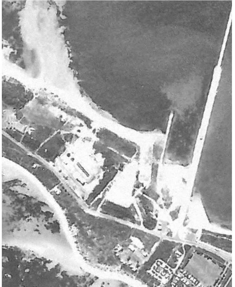
Right: Original sand trap groyne west of the Causeway - 1973 (1975 photograph)
