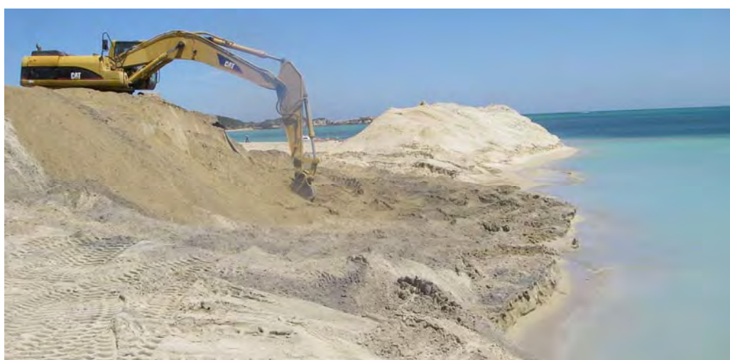
Figure 4: Sand trap at Point Peron during excavation works in November, 2007
