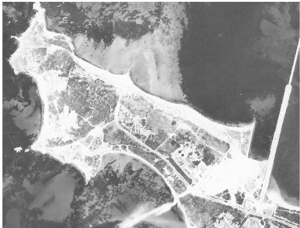
Below: Original sand trap groyne (1983 photograph)
