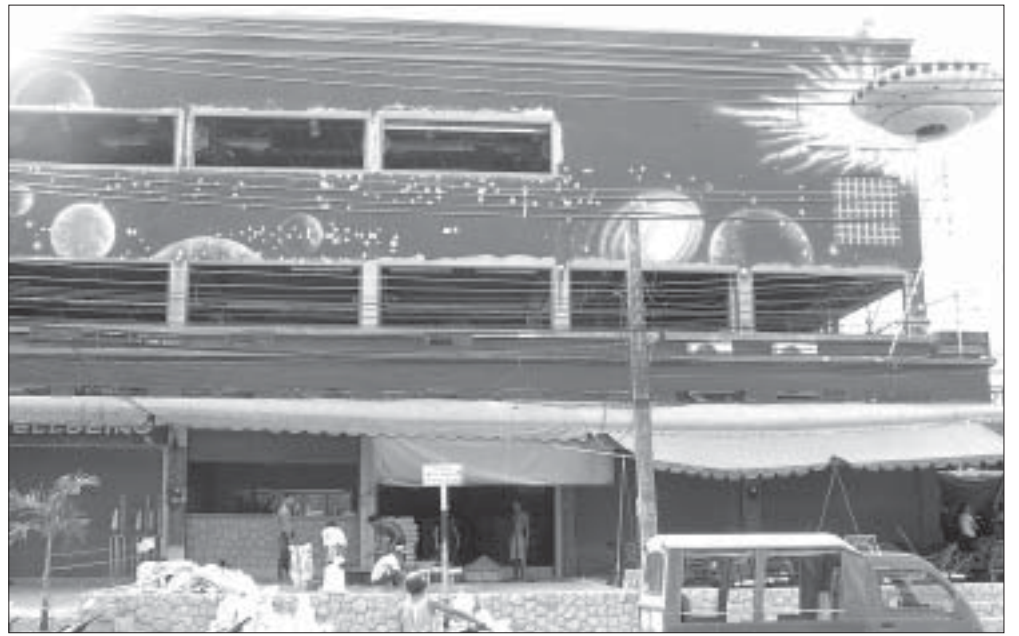
Let there be light: windows appear at Shark/Star Wars/Star World/Star Club. The outside has now been repainted a delightful puce color.
