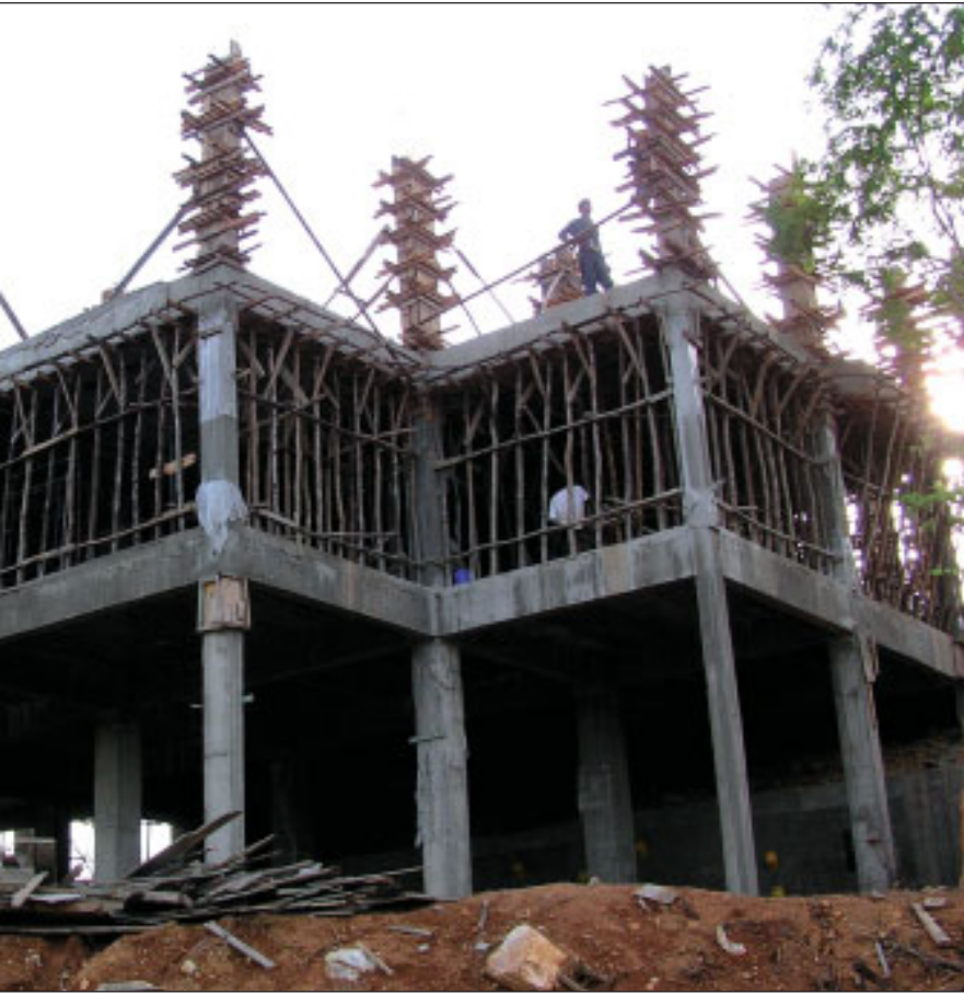
Construction is well advanced on the apartment blocks.
