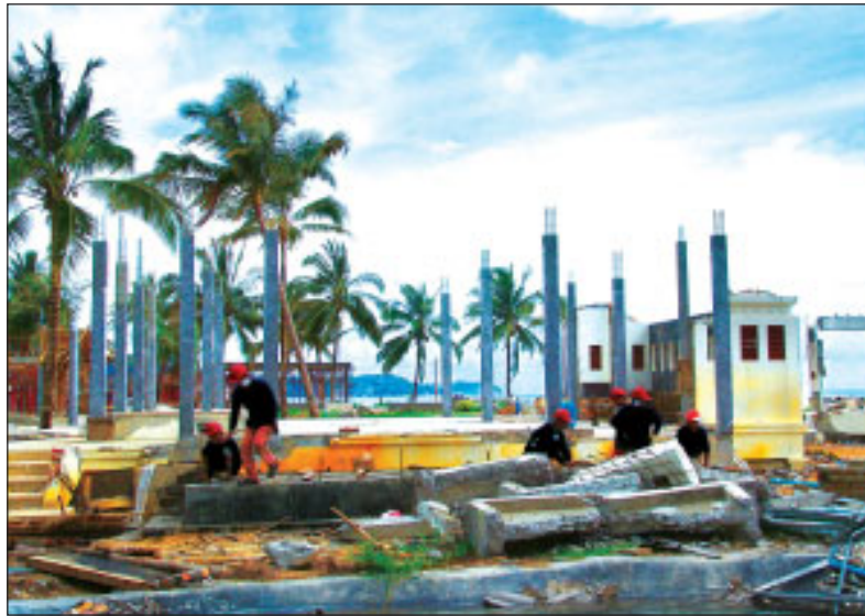
Among the Bang Niang resorts rapidly being rebuilt is the Mukdara.
