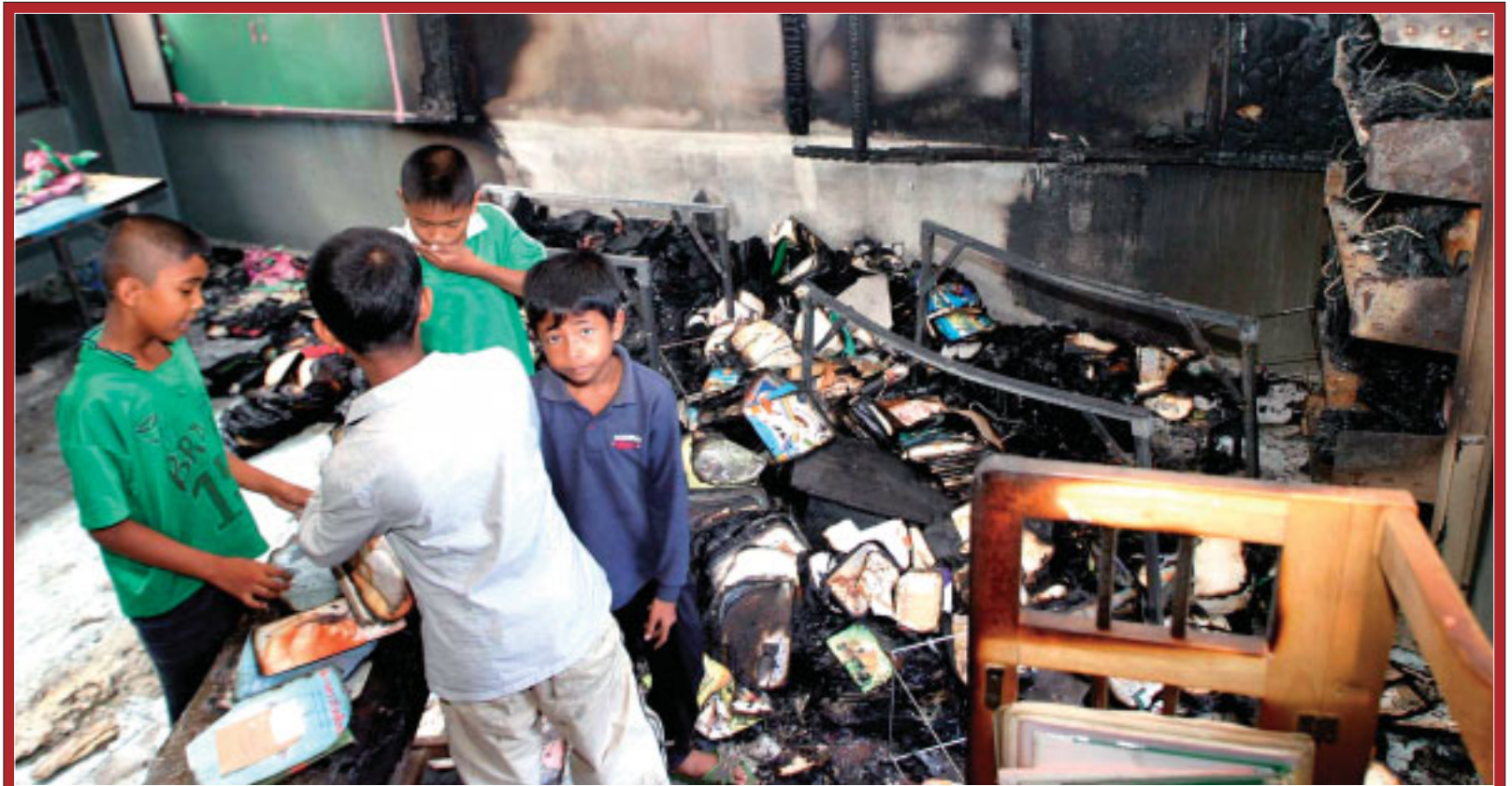
NO PLACE TO STUDY: Thai-Muslim children at Ban Kasot School in Yala try to salvage what they can from their burnt-out classroom, which was torched on the night of May 12. Many students in the Deep South are finding they have no place to study for the new school year after a spate of school burnings. While the arson attacks are thought to be the work of Muslim insurgents, their victims are often fellow Muslims.
