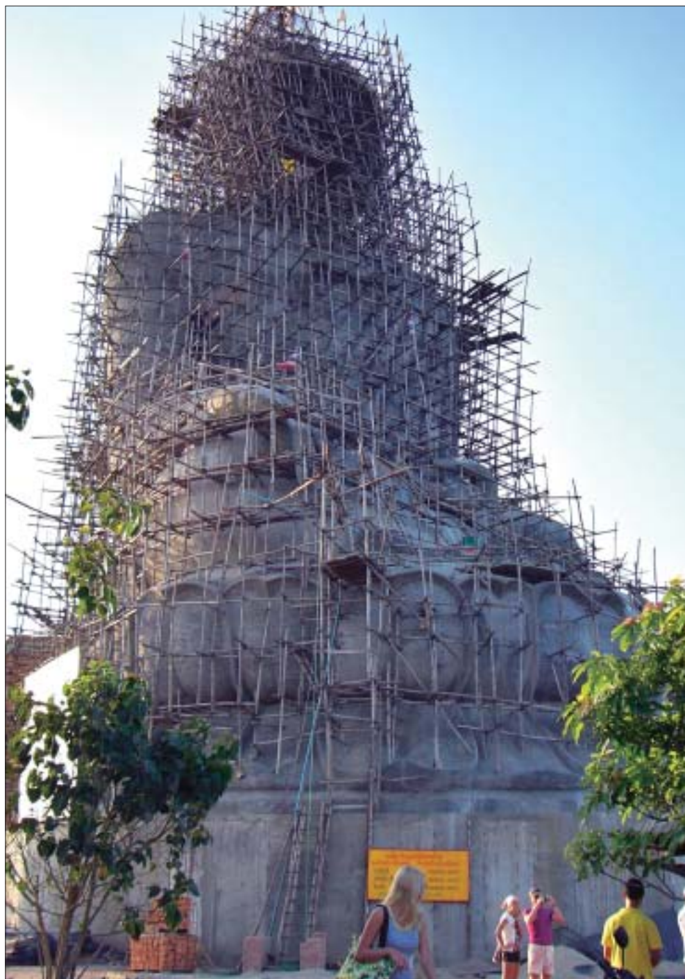
The Mingmongkol Buddha image is 45 meters high. Made of reinforced concrete which will be covered with white marble, the image is 24.5m across at the base, which features enormous lotus leaf motifs.
