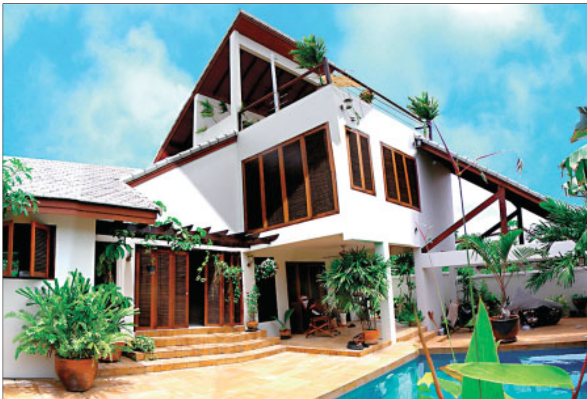
Look Ma, no aircon: The house is designed to take full advantage of natural airflows.
