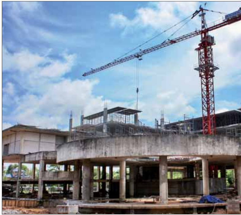
RISING HIGH: The new hospital under construction. Photo: Lesley Chittayanon
