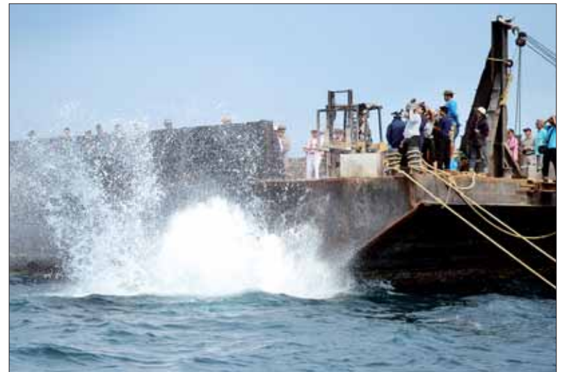
The 1,630 cubes, weighing a ton each, were placed in clusters of 80 to 100.
