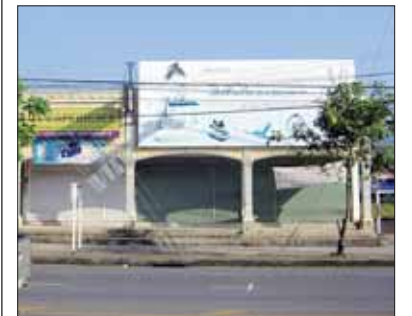
The already-vacated shops across from Tesco will be leveled to make way for the new retail complex.
