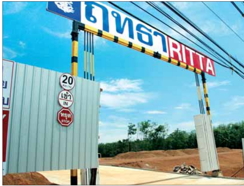
The site in Thalang has been cleared, ready for construction.
