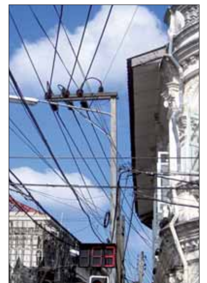
Cables along Dibuk Road, Phuket Town. Photo Chutharat Plerin
