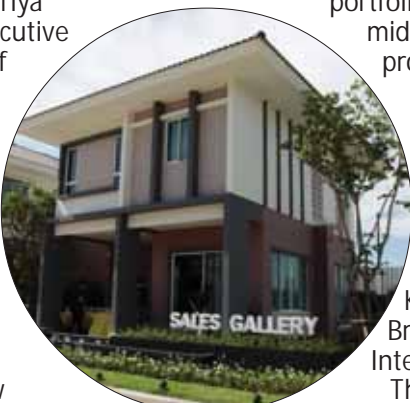
Habitia project in Kathu
