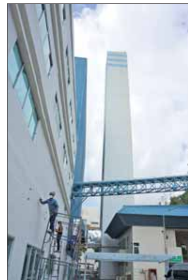
Outside the incinerator.
