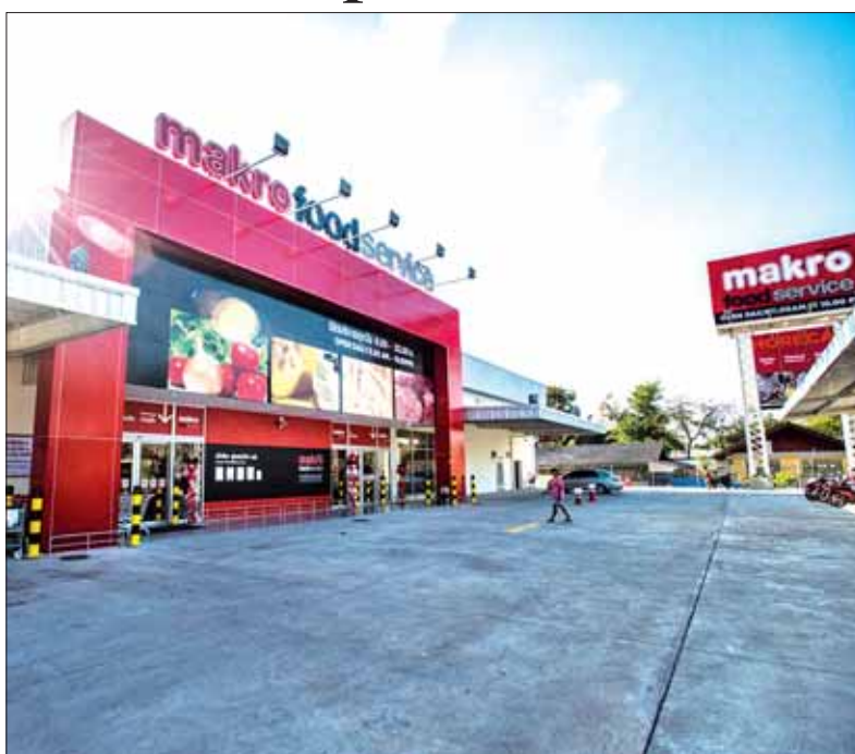
The new 1,700 square meter Makro in Rawai. Photo: Jeremie Schatz
