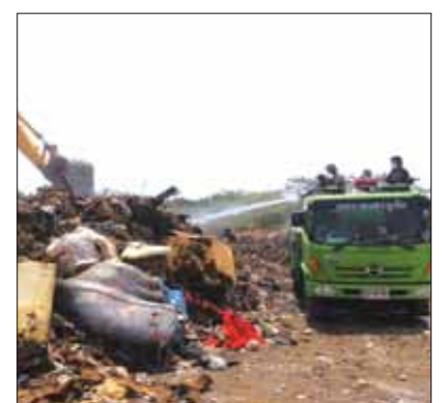
A water truck douses rubbish at the landfill.
