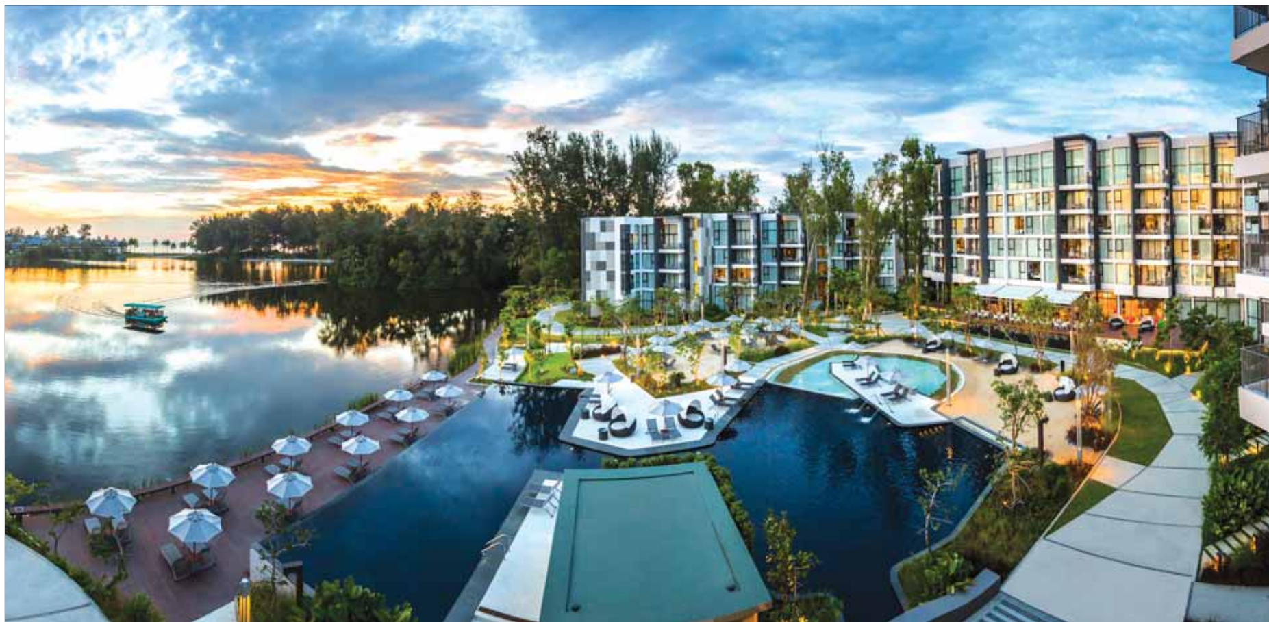
The Cassia Phuket apartment complex in the grounds of the Laguna Phuket resort overlooks an expansive lagoon and gives residents panoramic views of the Andaman Sea.
