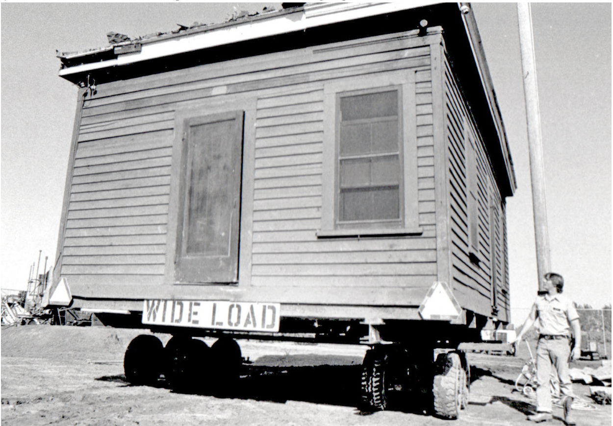
On November 4, 1984, Fisher Brothers House Moving Company transported Charles Weber’s first home in Stockton to the Museum, where staff and volunteers restored it to its appearance in 1848 and developed an area of the Museum’s campus to simulate Weber Point.
