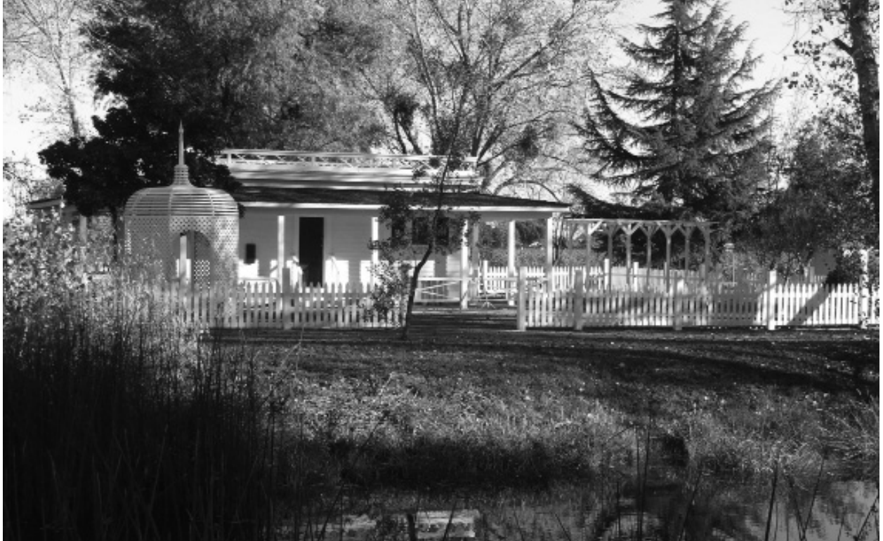
The 1848 Charles Weber cottage, ca. 2010.
