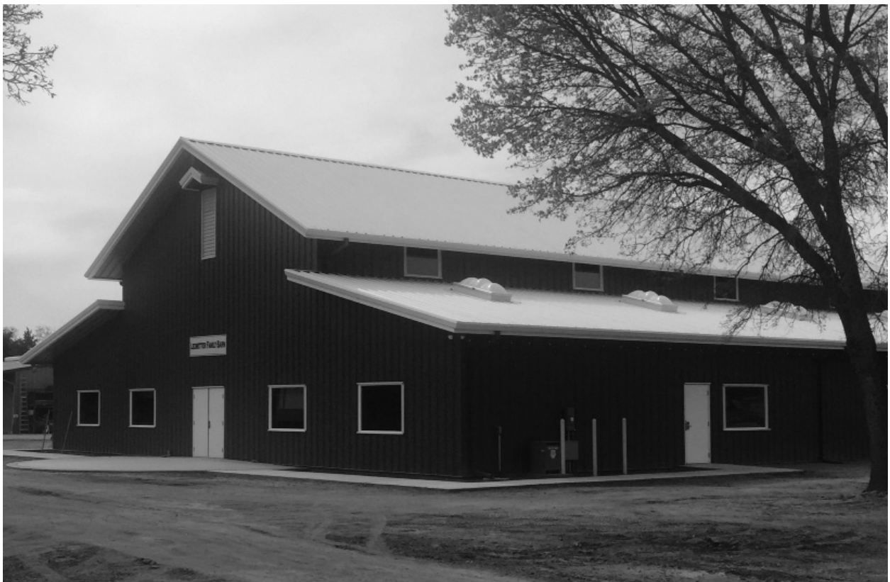
Ledbetter Family Barn exterior, 2015.
