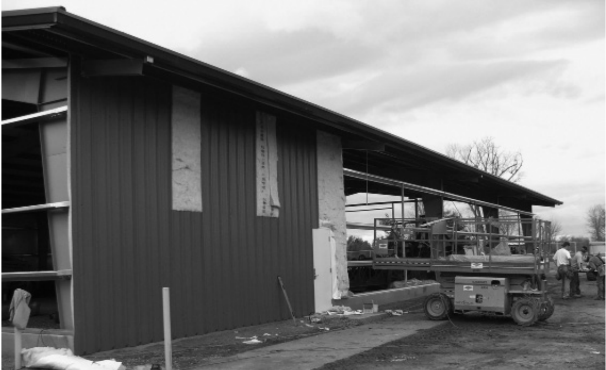
Enclosing the Brown-Jones Building with siding, 2011.
