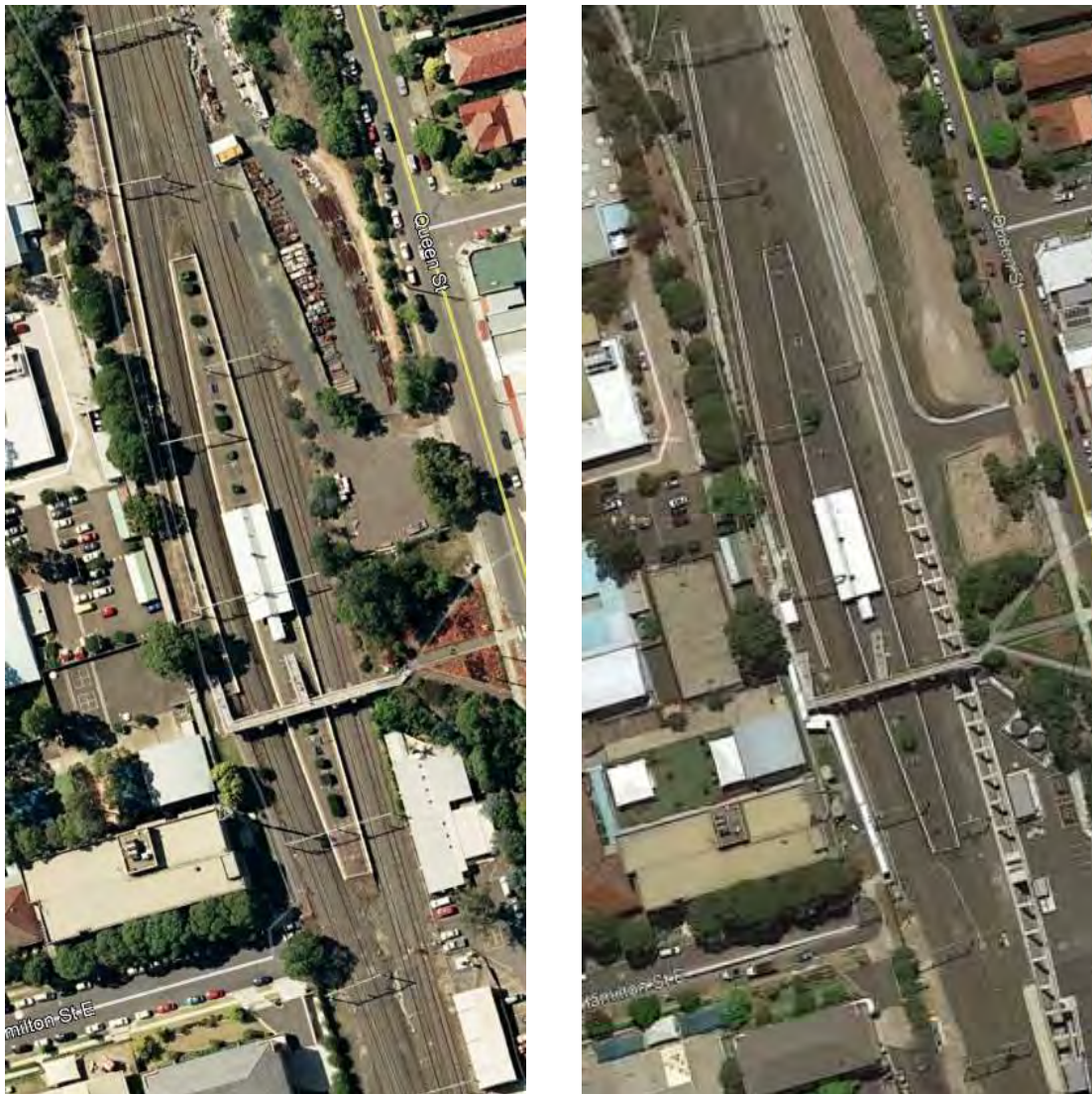
Figure 5. North Strathfield Station in 2009 (left) and in 2018 (right) showing the construction of the NSRU line in the intervening period. (Source: GoogleEarth)
