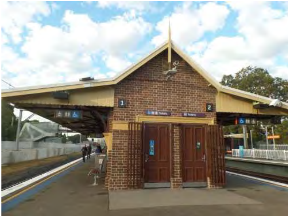
Figure 10. North Strathfield Railway Station - northern end of platform building
