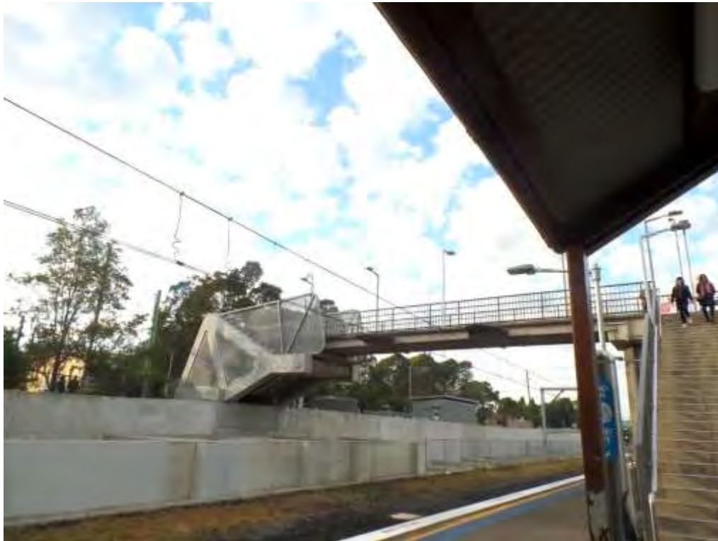
Figure 13. The non-original overhead pedestrian footbridge to North Strathfield Railway Station.
