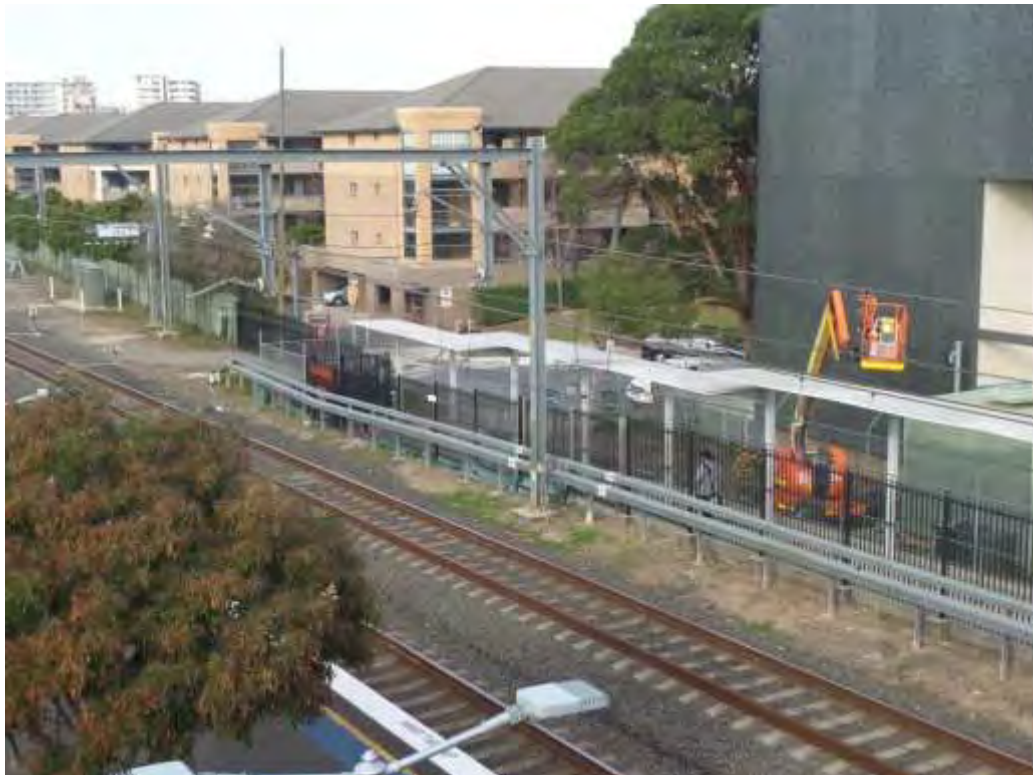
Figure 12. The pathway from Hamilton Street to North Strathfield Railway Station, below the white canopy roof carried on white posts.
