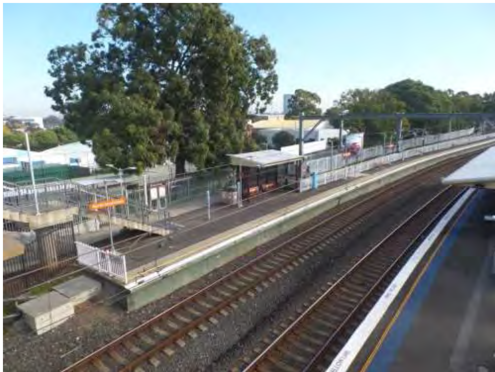
Figure 14. Platform 3 at North Strathfield Railway Station has no heritage buildings or structures
