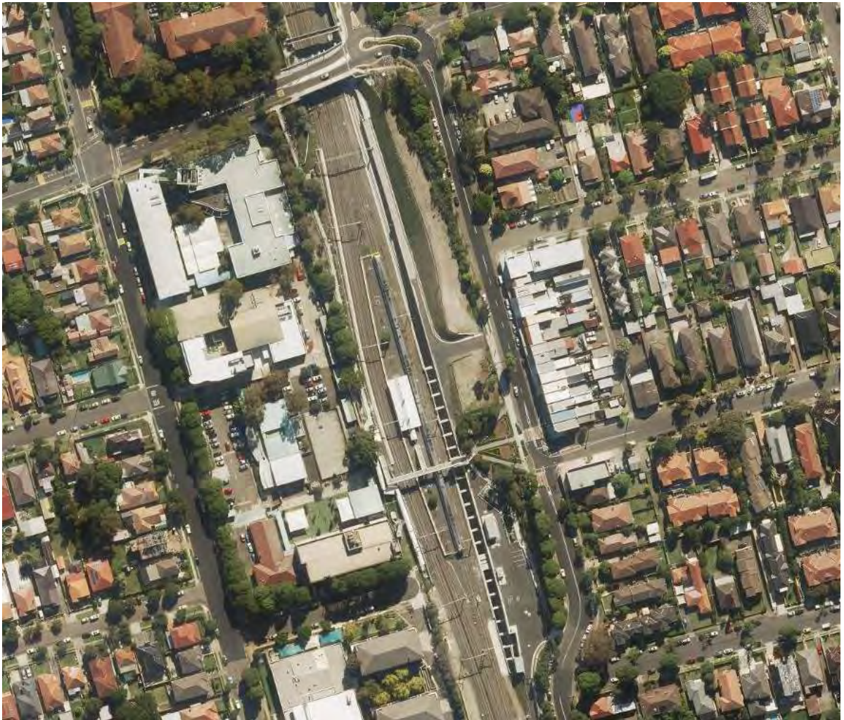
Figure 2. Aerial photograph of North Strathfield Railway. (Source: SIX LPI).
