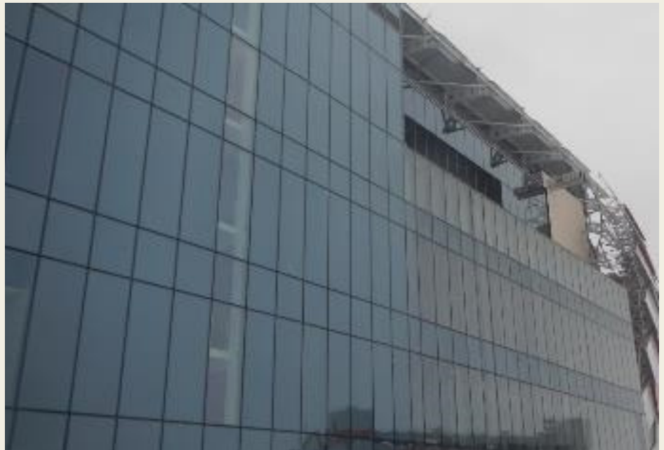
Fig. 5. Glazed facade of the stadium
