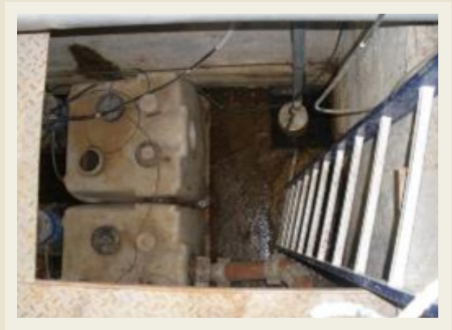
Fig. 54. Grease trap
