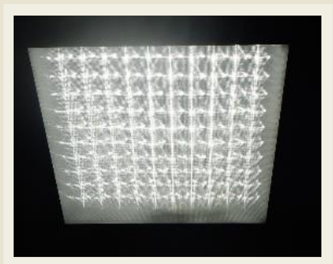
Fig. 38. Stadium illumination by LED lamps
