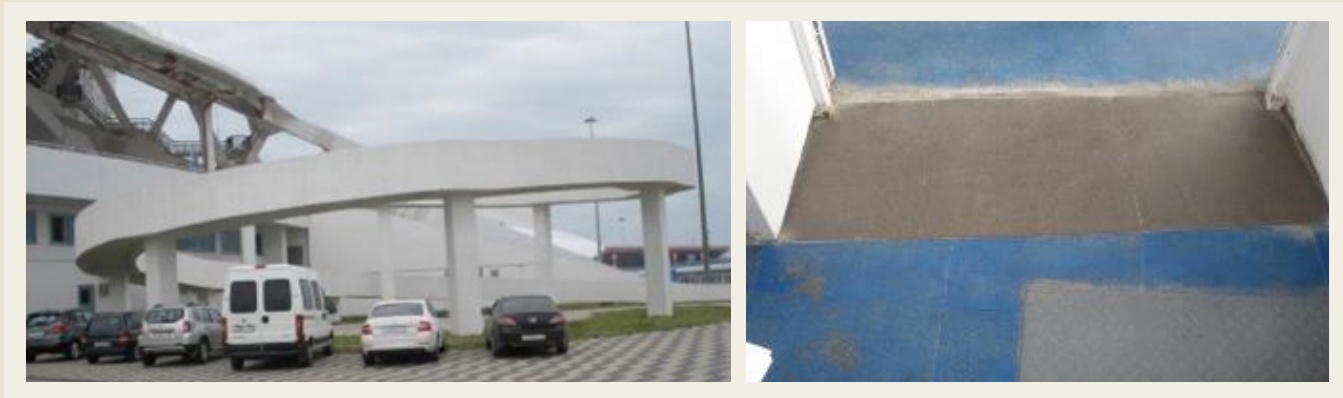
Fig. 48. Stadium infrastructure for disabled people and people with limited mobility. 1: Elevation to the upper levels; 2: Levelled sill
