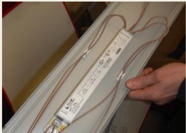
Fig. 12. 1: LED lamps installed at the stadium; 2: Electronic start control device on fluorescent lamps
