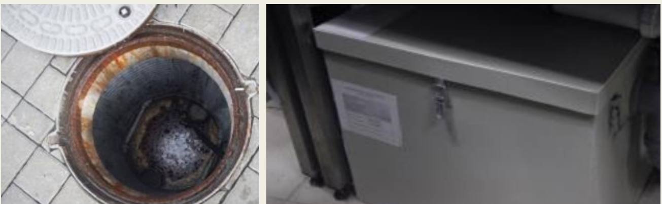
Fig. 19. Industrial and local grease traps at Spartak Stadium
