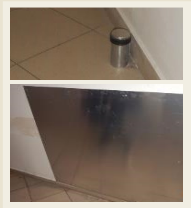
Fig. 14. Wall protection elements
