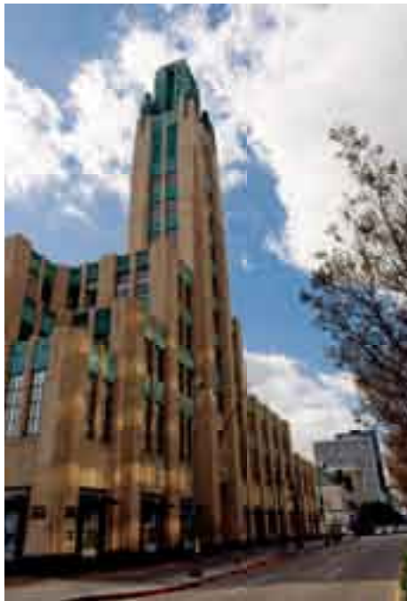
The historic Bullock's Wilshire building, Los Angeles, which today houses Southwestern Law School. Photo: Emile Askey. (GCI)
