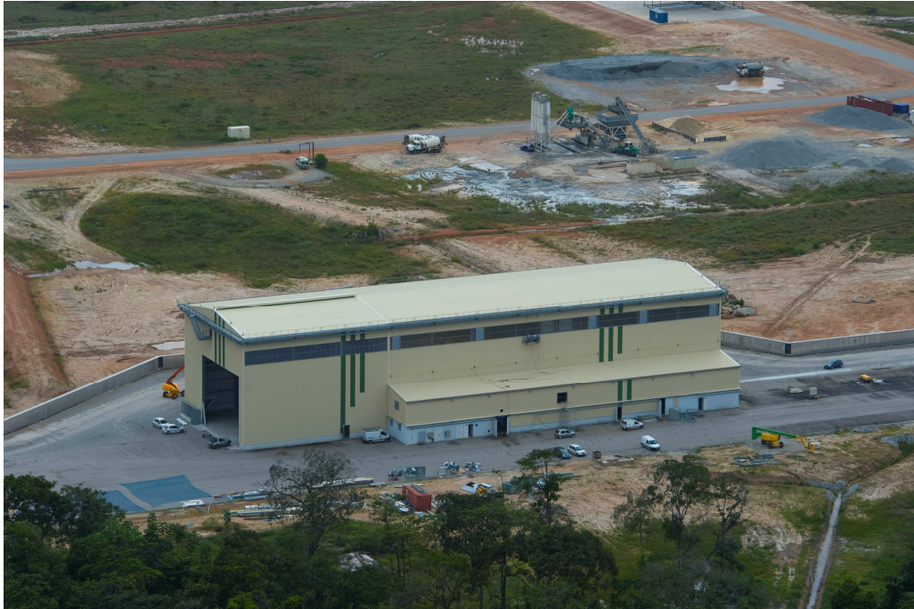
Figure 6.2.3.2.1a – LV assembly building (MIK)
