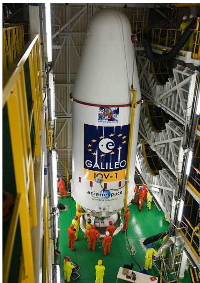
Figure 6.2.3.2.2c – Upper composite hoisting on Launch Vehicle
