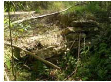
Figure 39 Retaining wall south of the culvert outlet.
