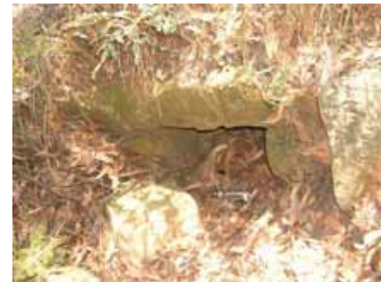
Figure 44 The intake of culvert 7 from south side
