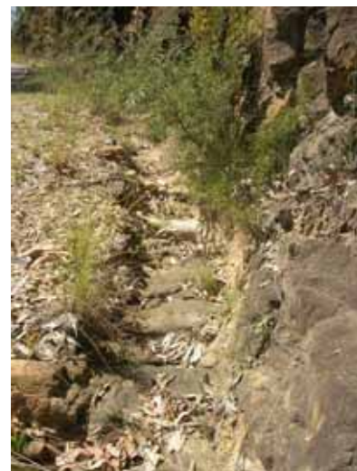
Figure 48 Drainage at base of rock cutting
