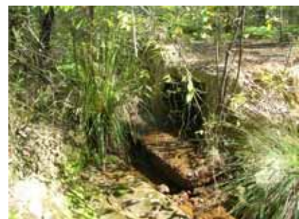
Figure 38 Culvert on Brookside Creek
