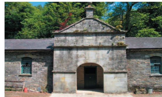
Central block of the stables (c. 1840) at the Allt-y-rodin estate showing the size of the ashlar blocks formerly available from Gwarallt Quarry.
