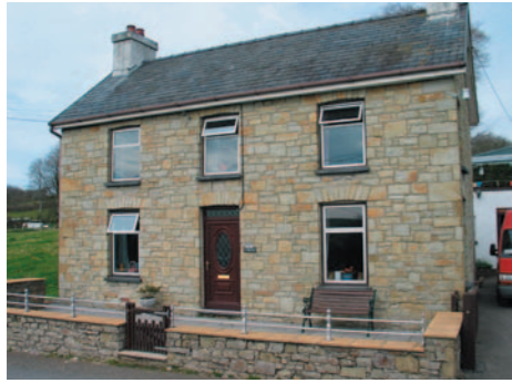
Early 20 th C. house in Talgarreg (newly cleaned) built with Gwarallt Stone.
