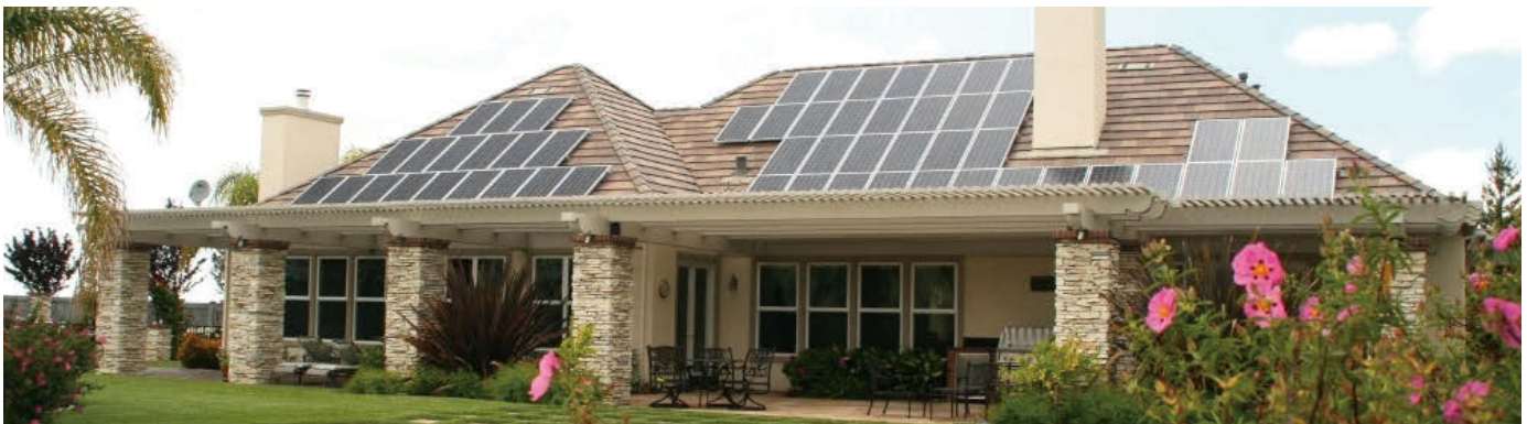
Residential PV installation in California
