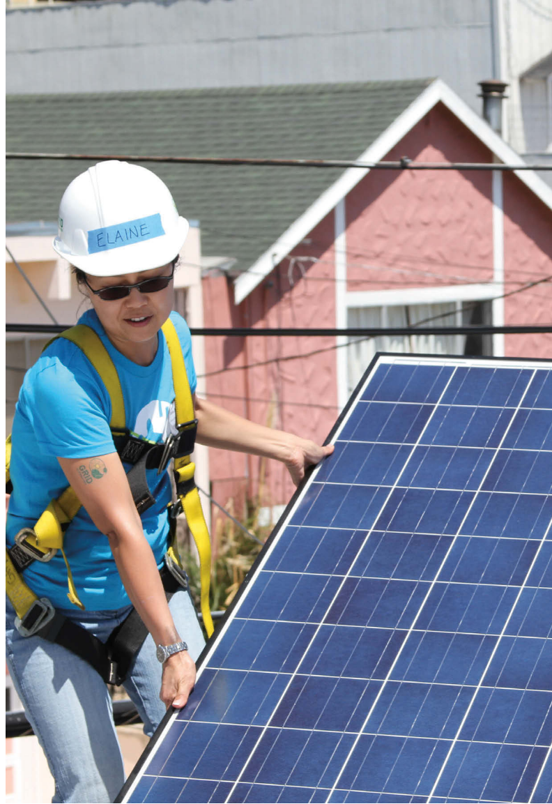
Worker installing PV system
