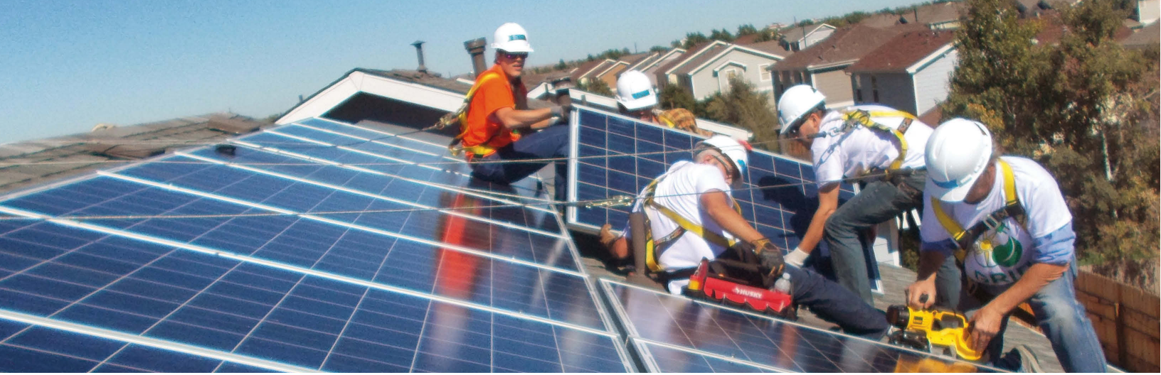
Workers installing PV modules
