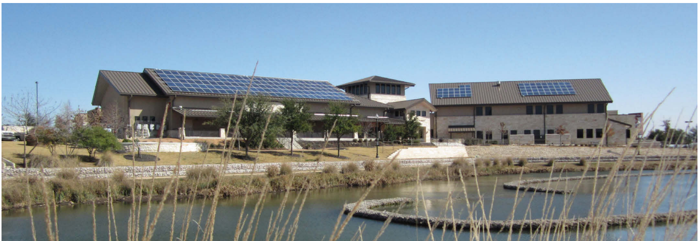
Non-profit PV installation in Austin, Texas
