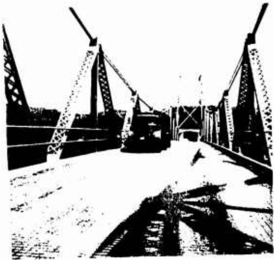
Fig. 2. On Bridge Deck. Test Vehicle
