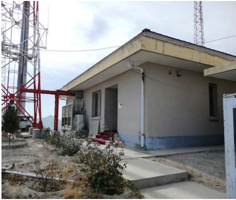
[Photo25] Appearance of Kabul TV Transmission Site
