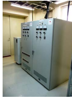
[Photo28] AVR for TV Transmitter
