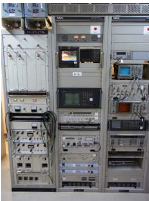
[Photo27] STL/TSL, PIE, Measuring Instrument Rack
