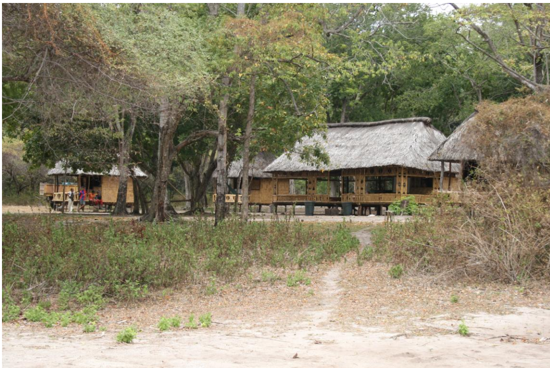
Figure 1.5. Ecotourism village under construction adjacent to a beach near Jaco Island.
