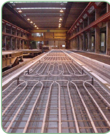
Photo 1: Prefabrication of slabs with integrated piping.
