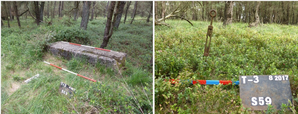
Figure 6 (left): Concrete part of a construction, found in the direct vicinity of the Freya radar. According to an employee of landowner Natuurmonumenten, it has been removed from it's in situ spot by foresters during the 80s of the last century as it stood in the way. Figure 7 (right): one of the iron anchors for guy-wiring in situ at the location of one of the eight known antenna masts for transmission (Photographs by M. Reinders, August 2017).
