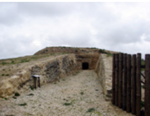
Tunnel. Fort Zambujal. Photo: MM
