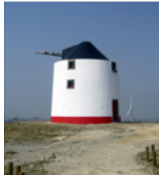
Windmill at Fort Novo. Photo: MSMA
