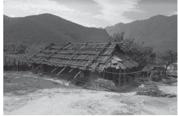
Plate 4 The houses of the H'mong people are made of planks split by axe from trunks of Taiwania and Fokienia (Cupressaceae).
