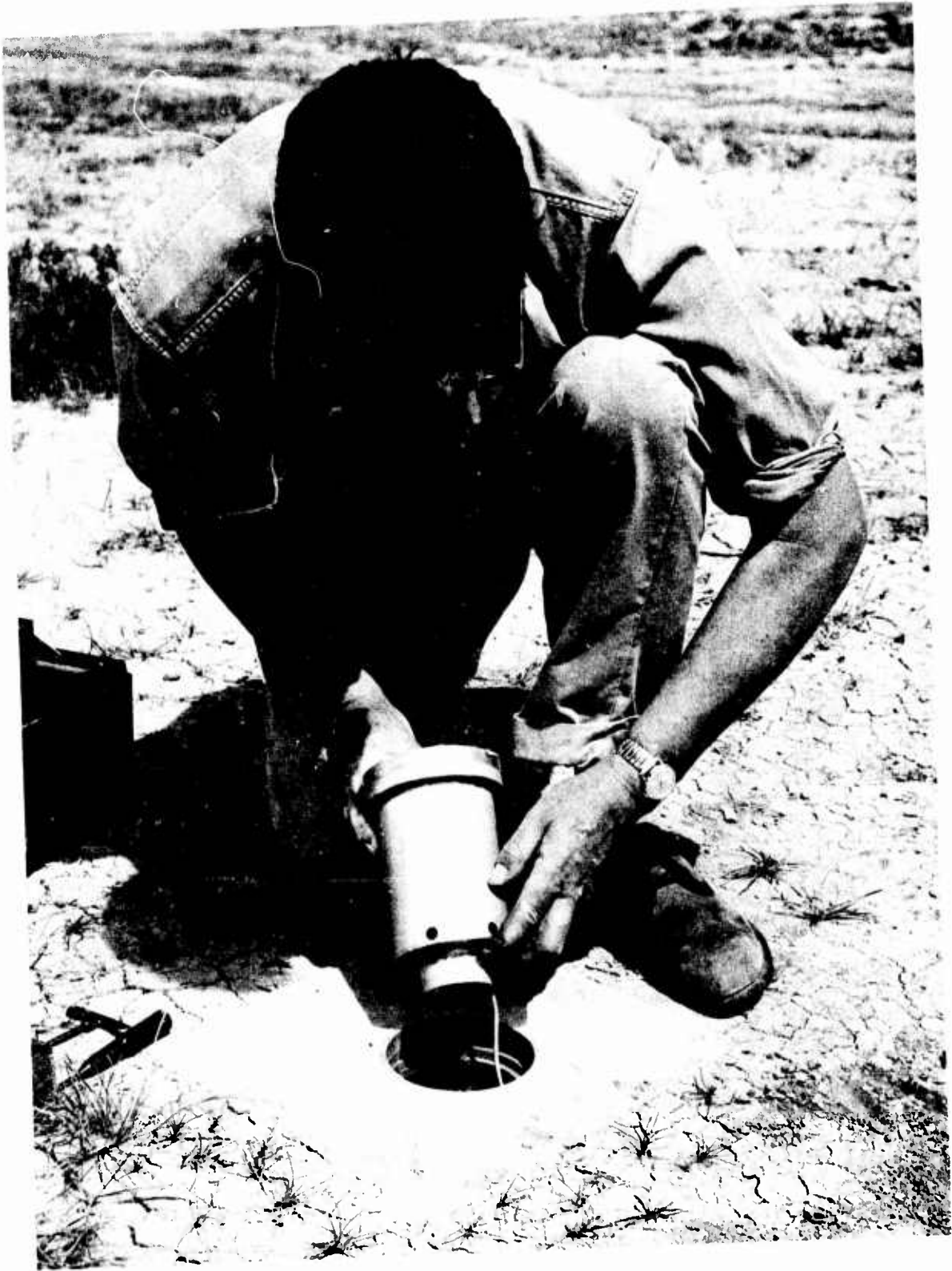
Figure 2.4 Installation of Self-Recording Gage
