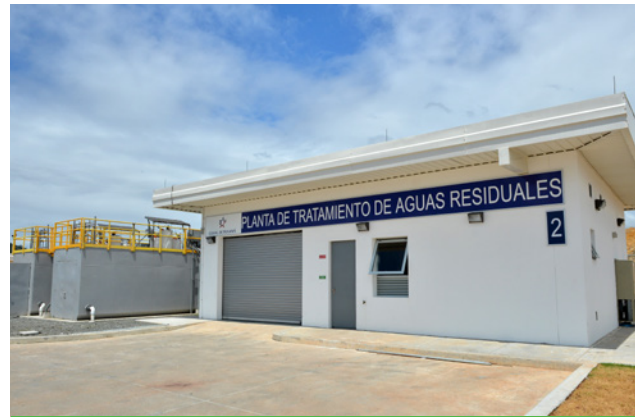
Wastewater Treatment Plant in Cocolí Locks
