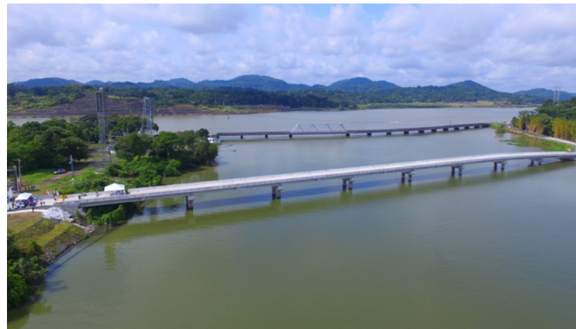
New Gamboa Bridge over the Chagres River
