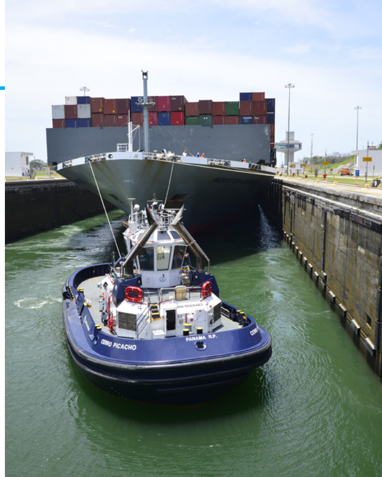
Tugboat assisting Neopanamax vessel in lockage operation
