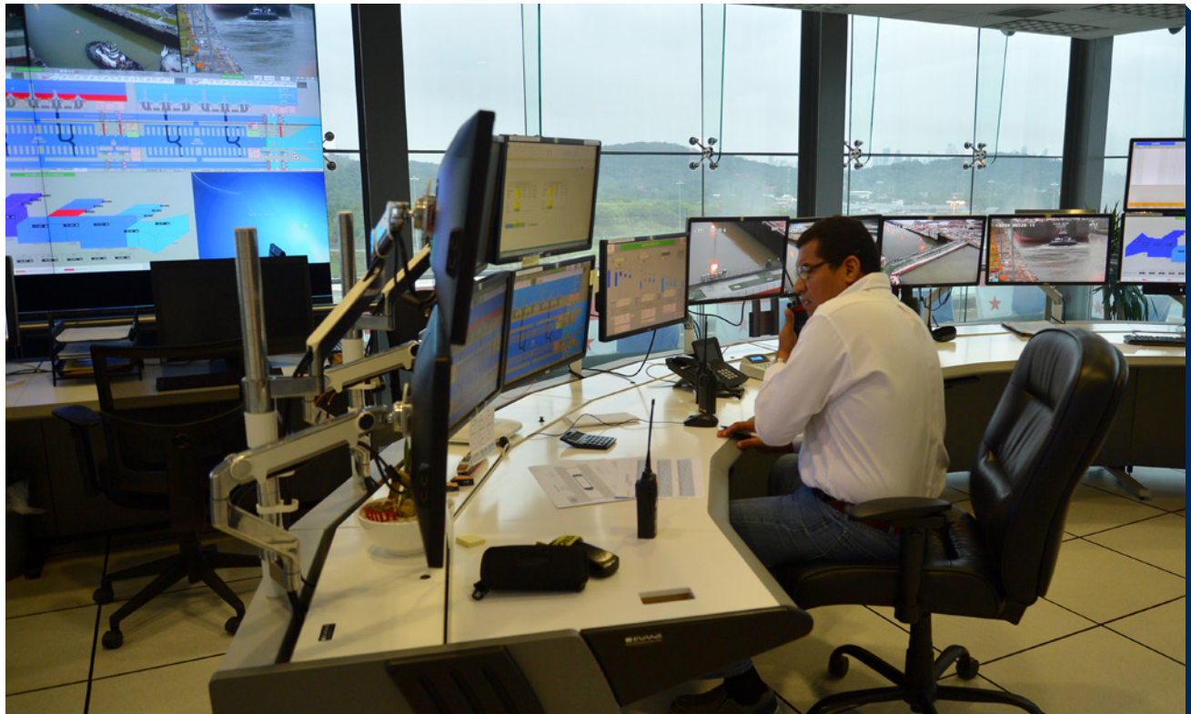
Employee working in the Neopanamax Locks Control House Operations Center
