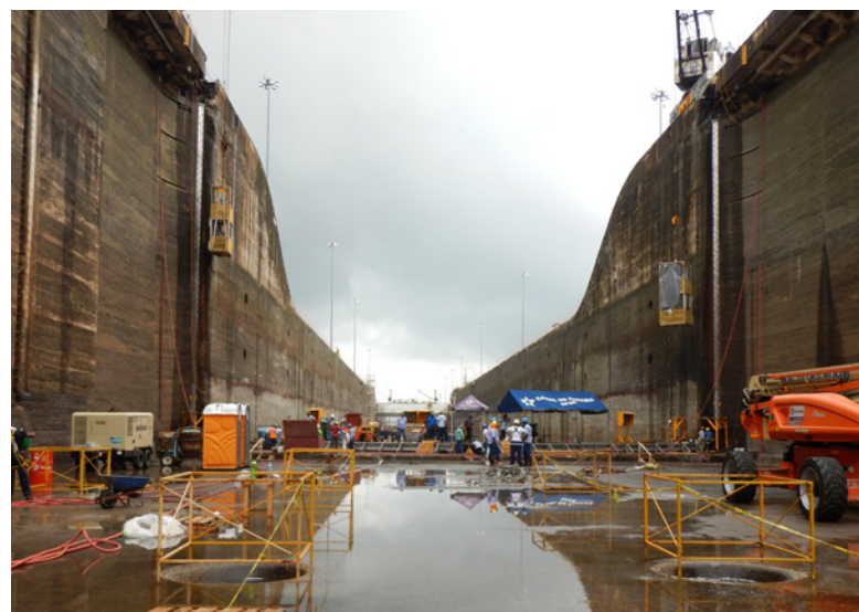
Panamax Locks' submerged equipment reconditioning
