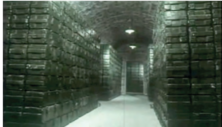
Protected ammunition and supply depots
