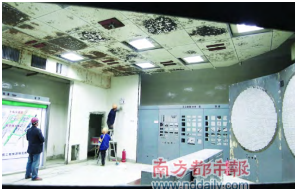
Control Room under repair
