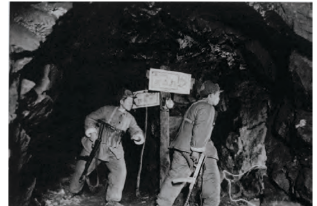
To carry out training activities in the tunnel.
