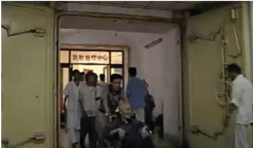
Heavy blast/anti-radiation doors on underground hospital
