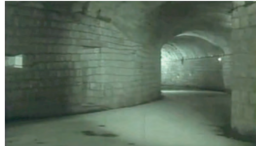
Part of interior lined with the old city walls of Beijing
