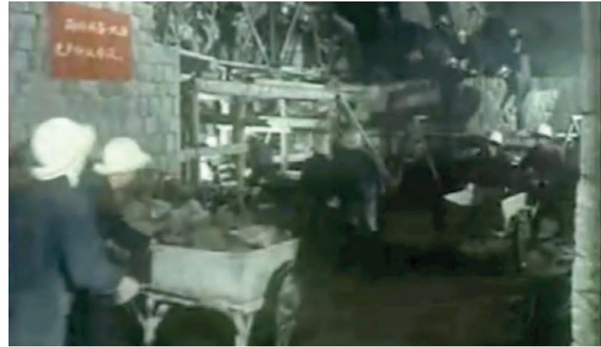
400,000 civilians participated in construction
