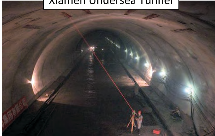
Xiamen Undersea Tunnel
