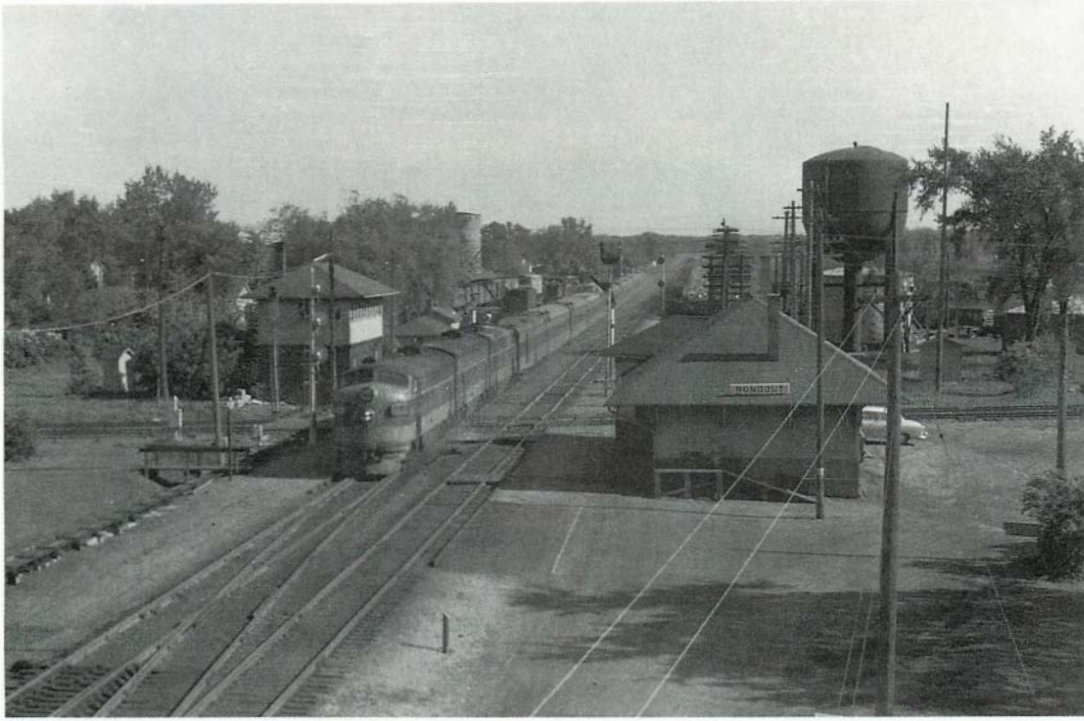
TOP LEFT: A set of FP7s power Milwaukee's Olympian Hiawatha through Rondout on May 15, 1955. Note the depot (razed in 1967) and the full extent of interlocking plant pipes connected to the tower. Also, the 1941 water tank is still in place—steam had three more months to run. BOTTOM LEFT: A pair of Fairbanks-Morse Erie-buils lead a CM-StP&P Milwaukee-Chicago train under the North Shore and through Rondout on March 16, 1957. The train is crossing over from the east-bound to the westbound main, probably to avoid a commuter or a freight train. Two photos, Barry Lennon collection
