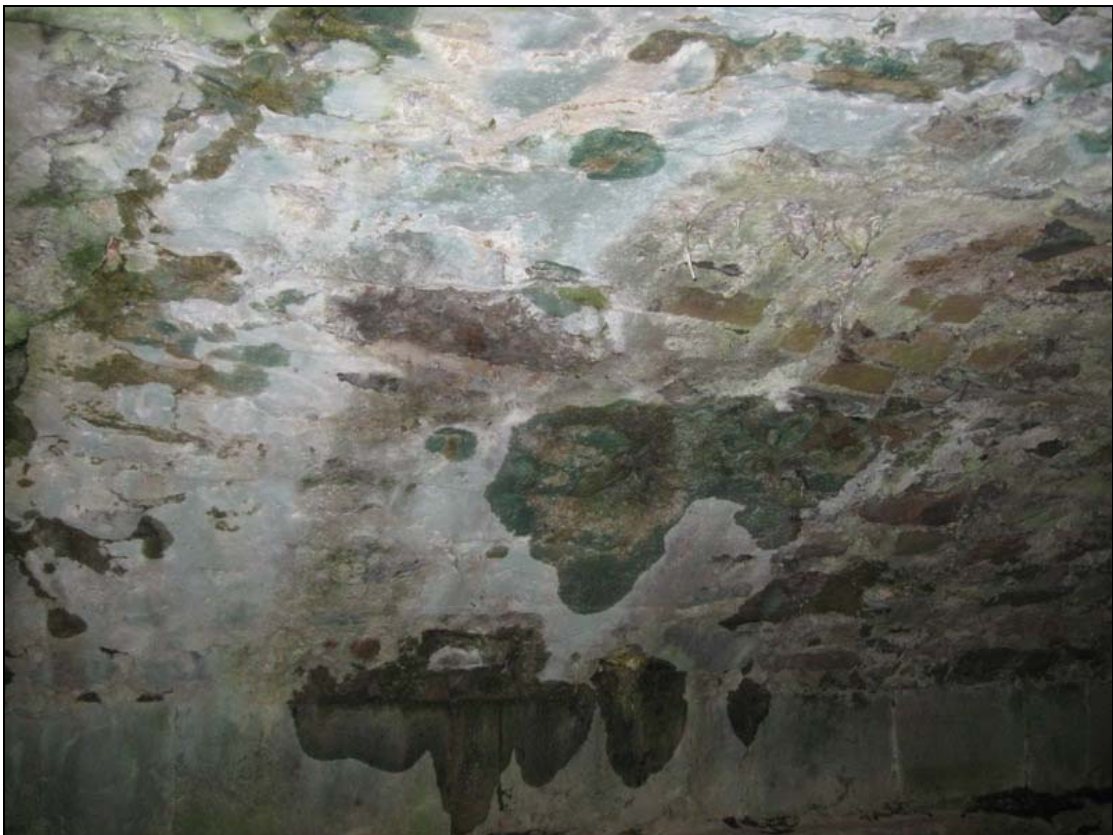
FHBS-09-NH-02 ~ Bridge underarch - lack of crevices
