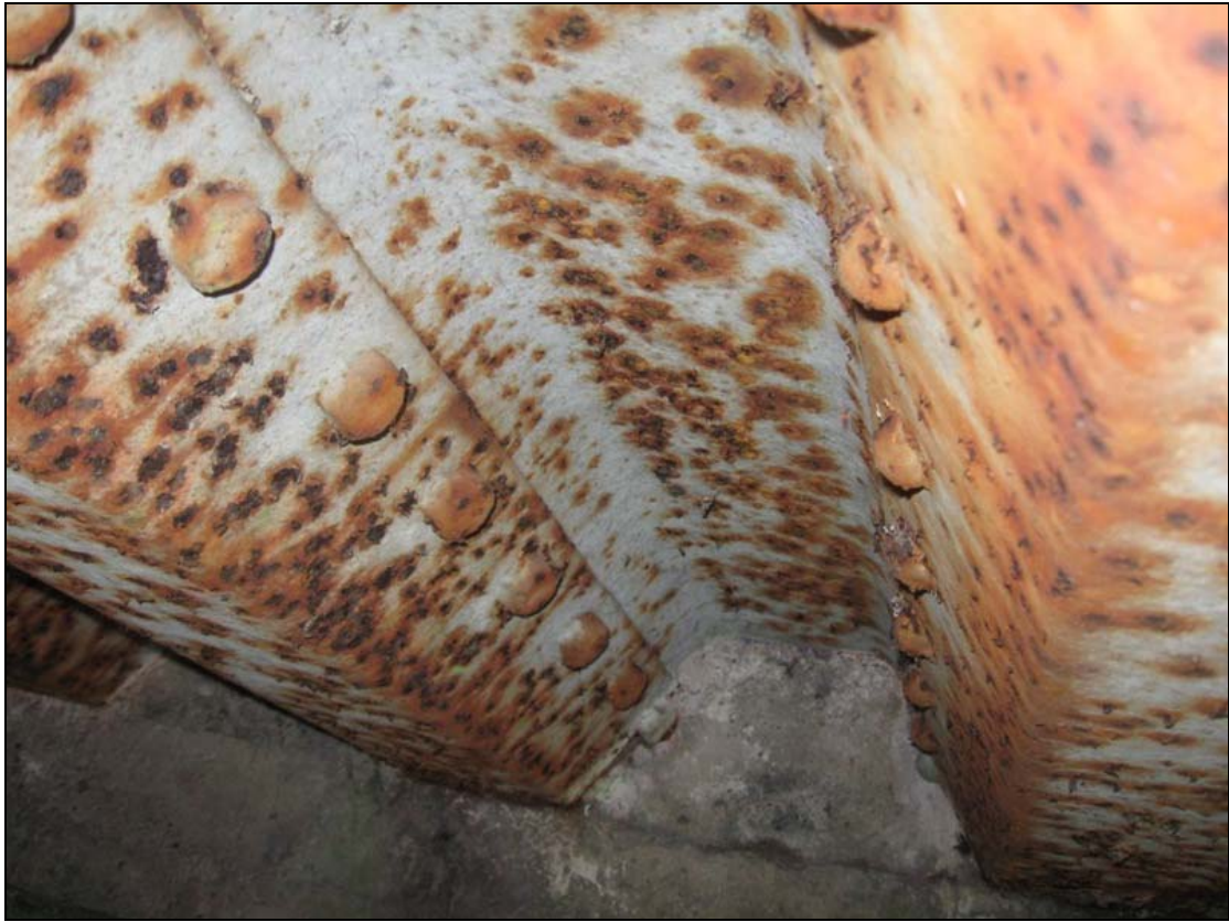
FHBS-05-NH-01 ~ Bridge underarch unsuitable for bat activity
