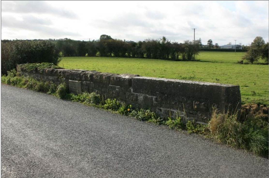
FHBS-03-BH-03 ~ West parapet from road
