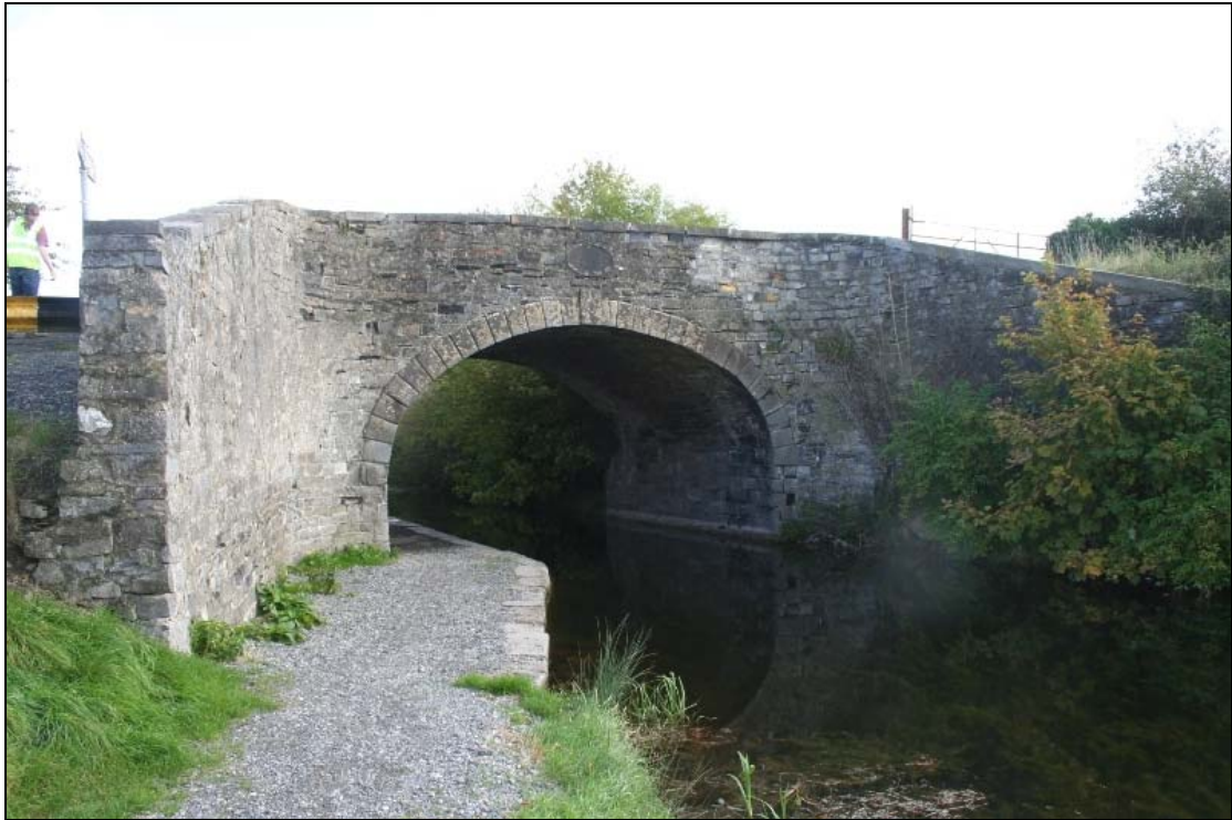
FHBS-15-BH-01 ~ West elevation of canal bridge
