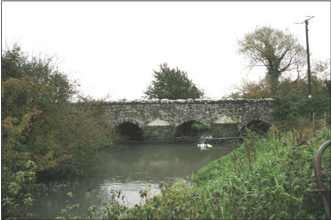
FHBS-12-BH-01 ~ West upstream elevation
