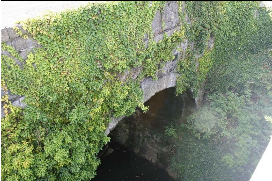
FHBS-13-BH-01 ~ East elevation from southern end of adjacent footbridge
