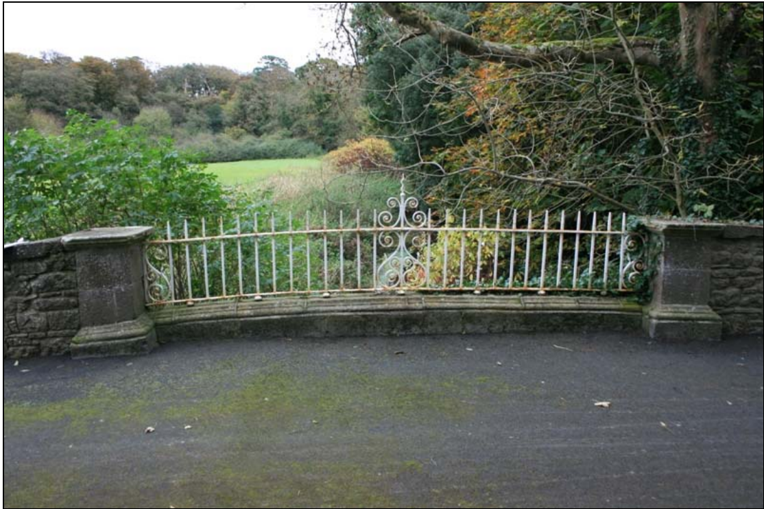
FHBS-09-BH-04 ~ East parapet from path
