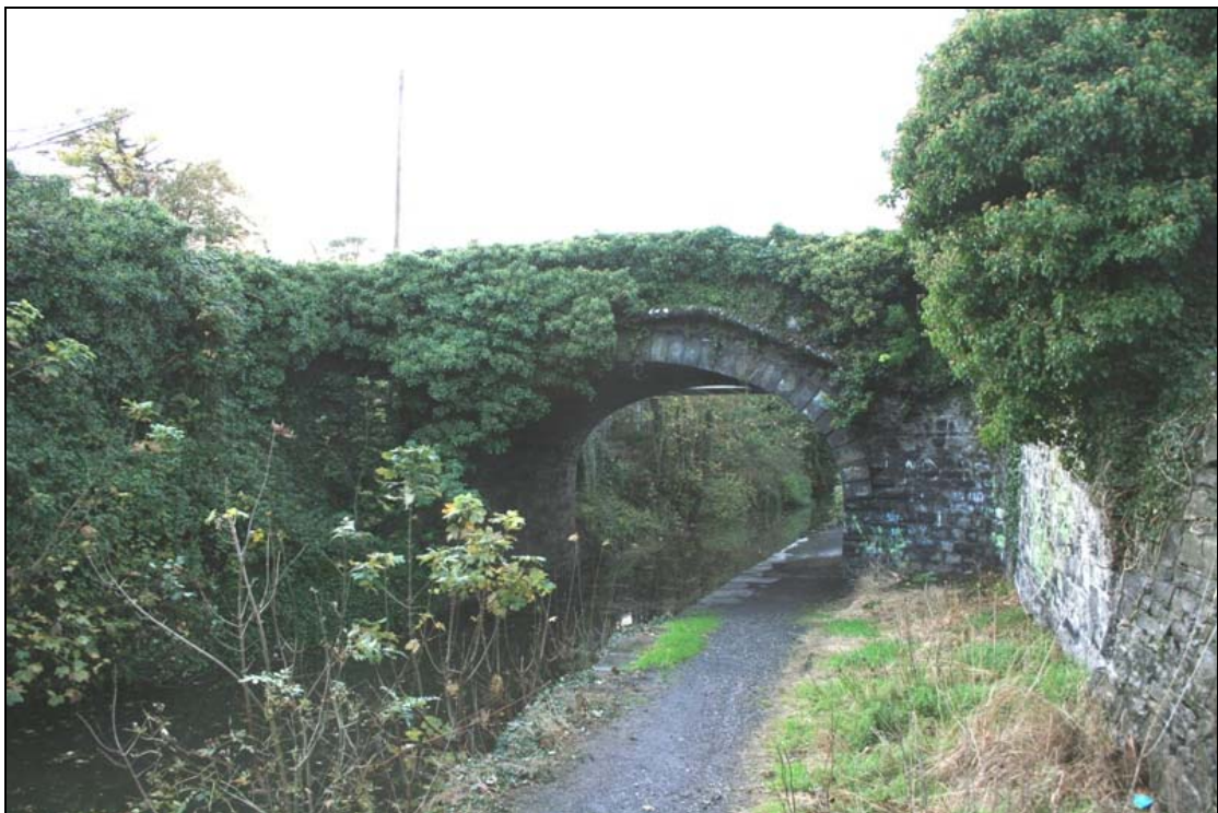
FHBS-14-BH-02 ~ East elevation
