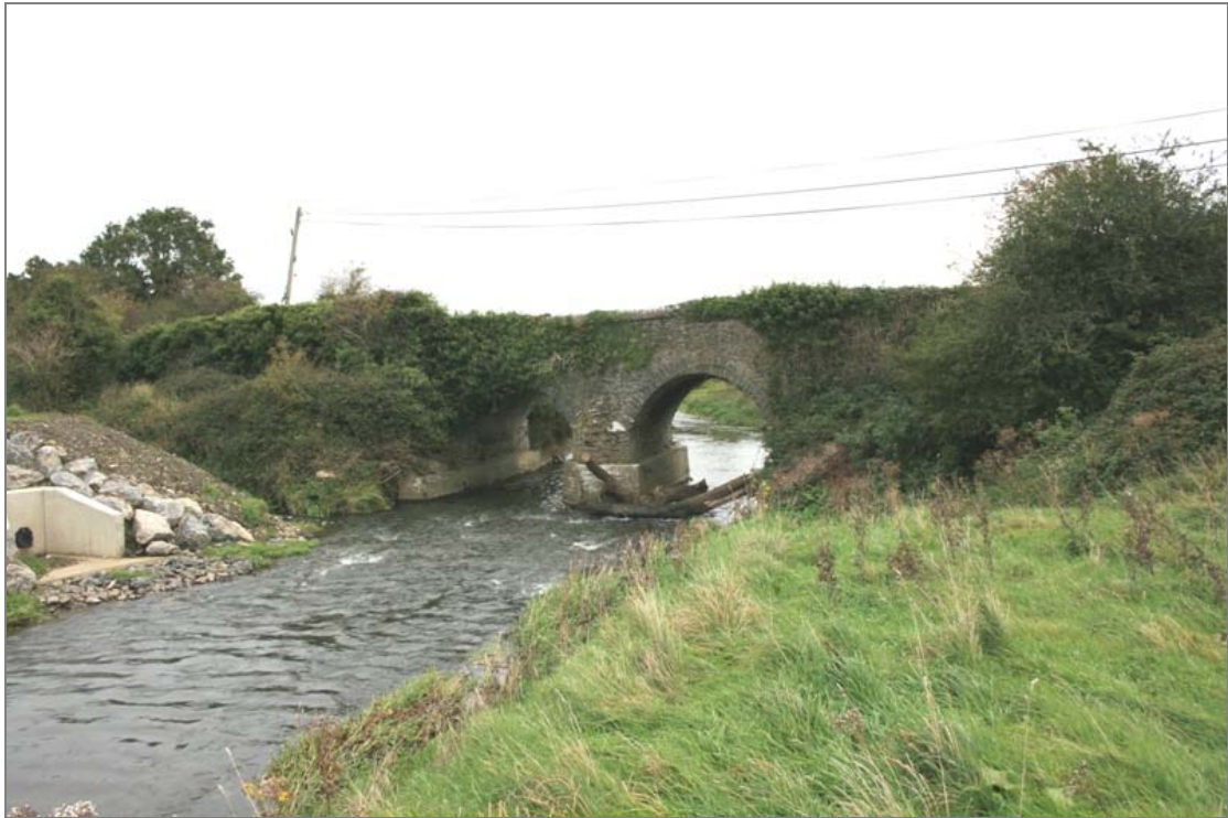
FHBS-07-BH-01 ~ West upstream elevation
