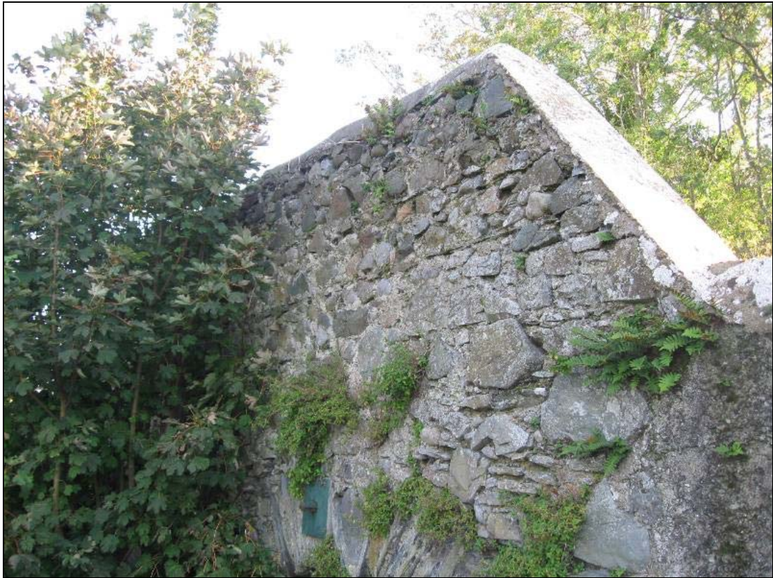
FHBS-01-NH-03 ~ Plant species diversity on bridge parapet
