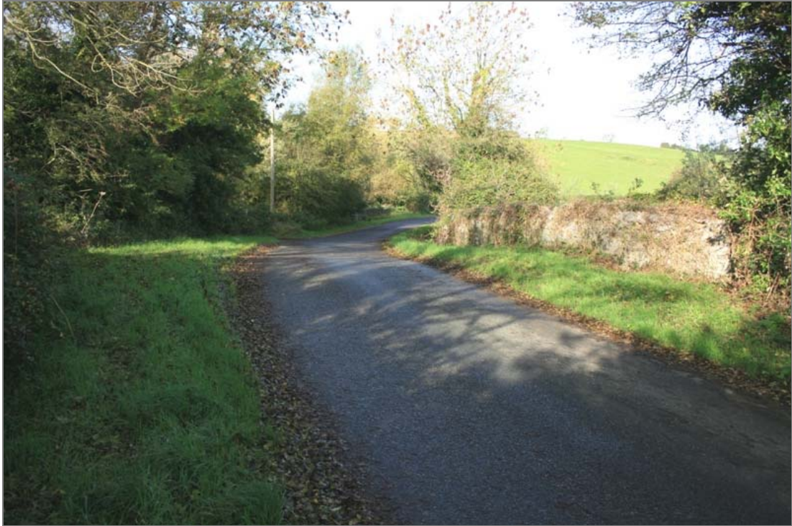
FHBS-02-BH-06 ~ General view of bridge from southeast
