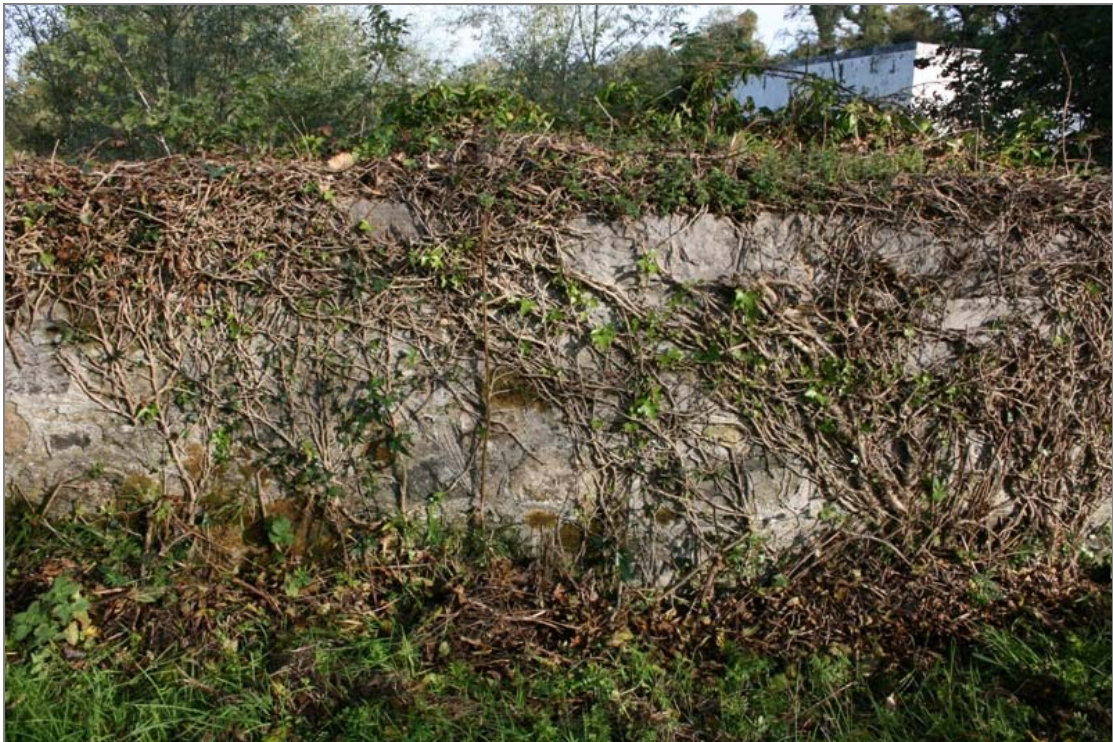
FHBS-02-BH-03 ~ North parapet from road
