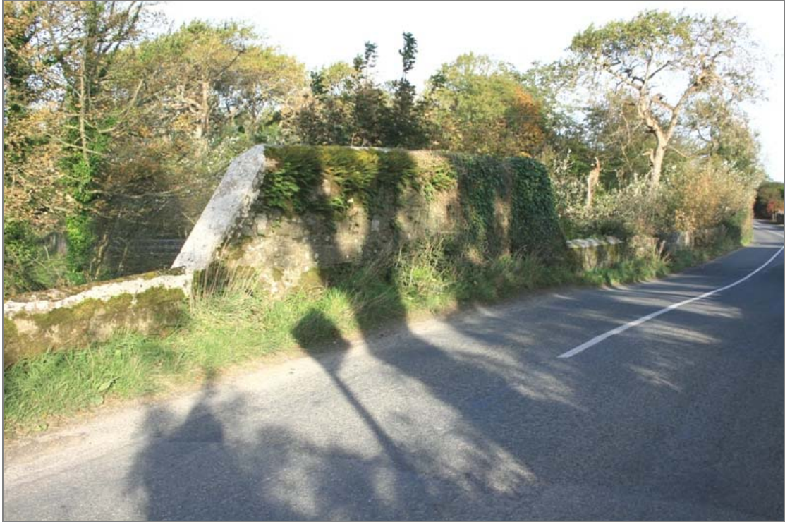
FHBS-01-BH-03 ~ West parapet from road
