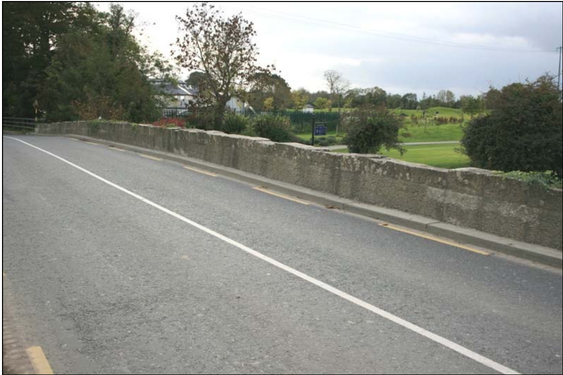
FHBS-08-BH-03 ~ West parapet from road
