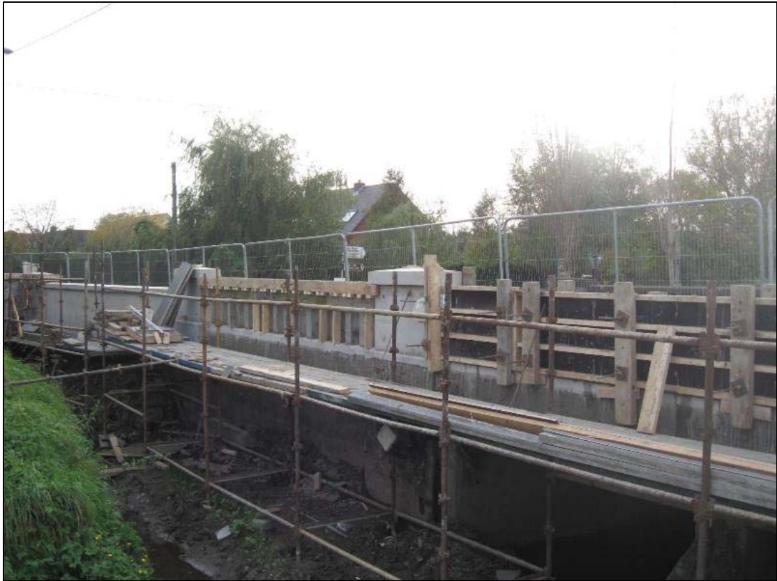
FHBS-06-NH-04 ~ Ongoing construction on downstream parapet
