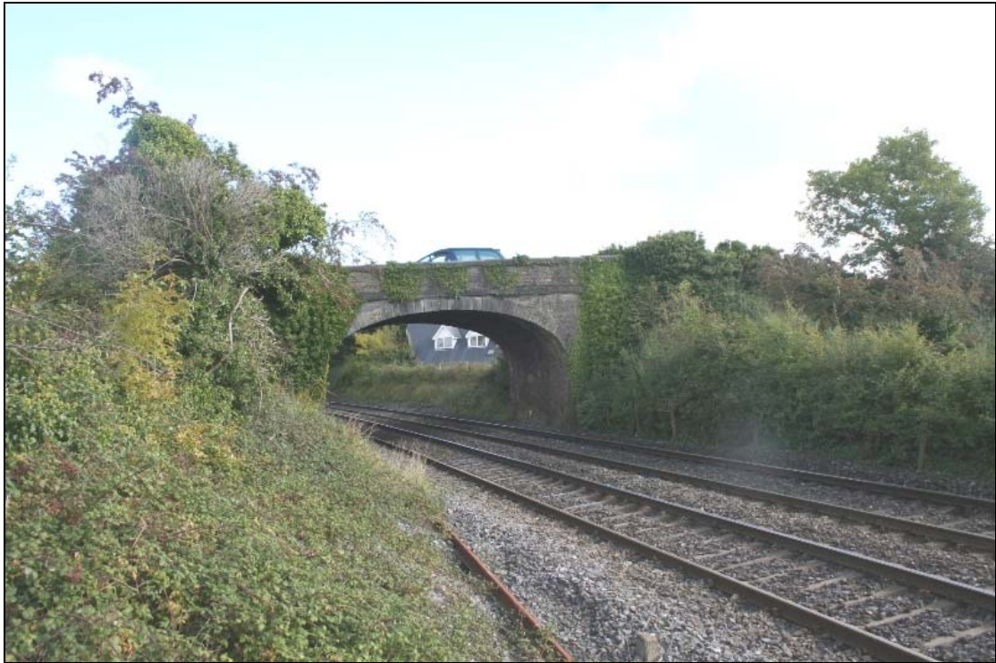
FHBS-15-BH-11 ~ West elevation of rail bridge
