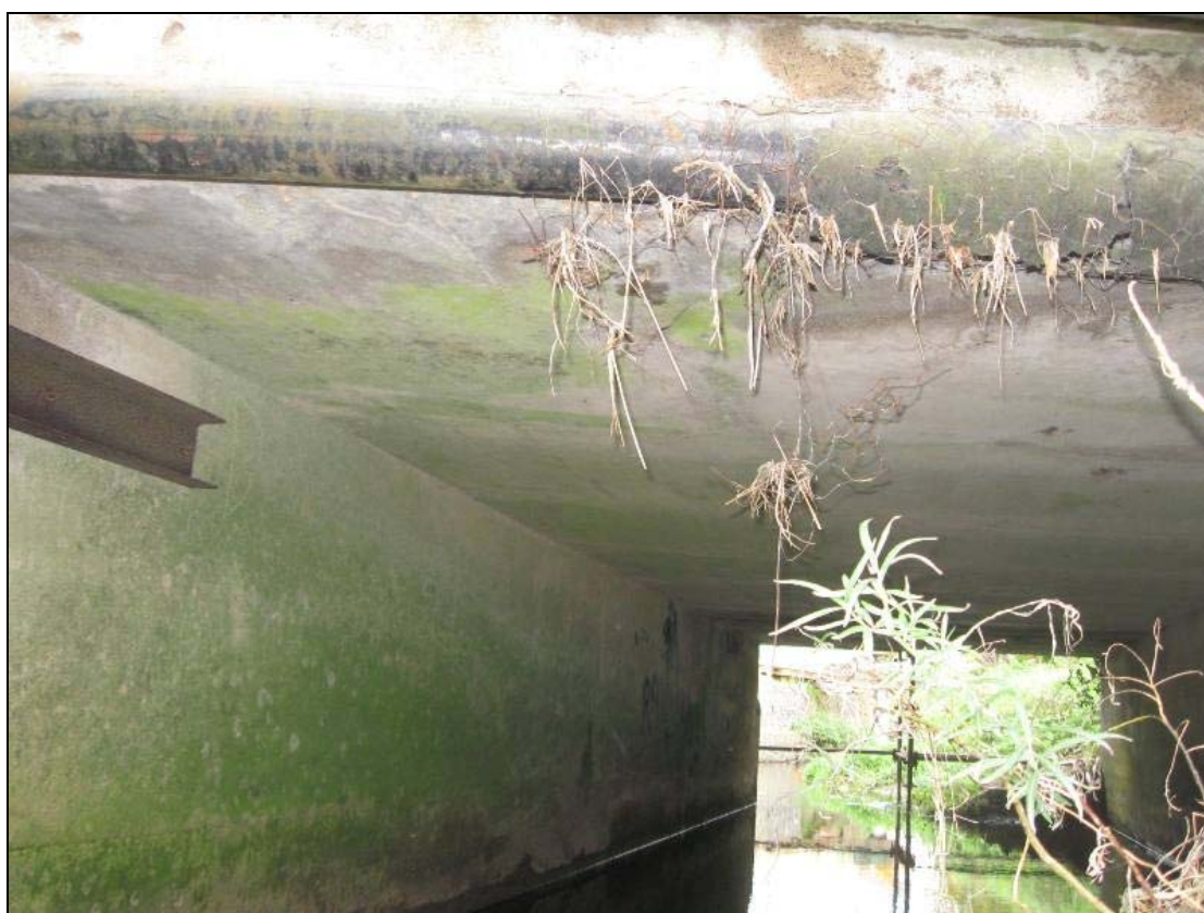
FHBS-06-NH-01 ~ Bridge underarch of cased concrete
