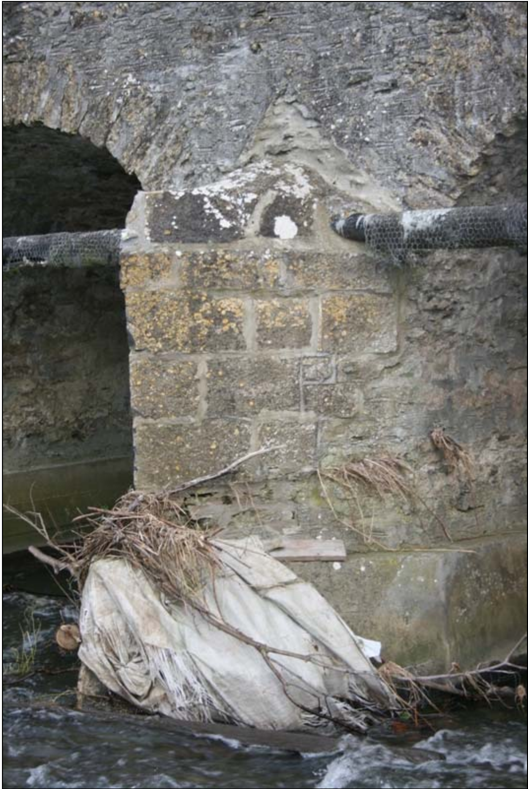
FHBS-08-BH-05 ~ Re-built stone cap of western cutwater
