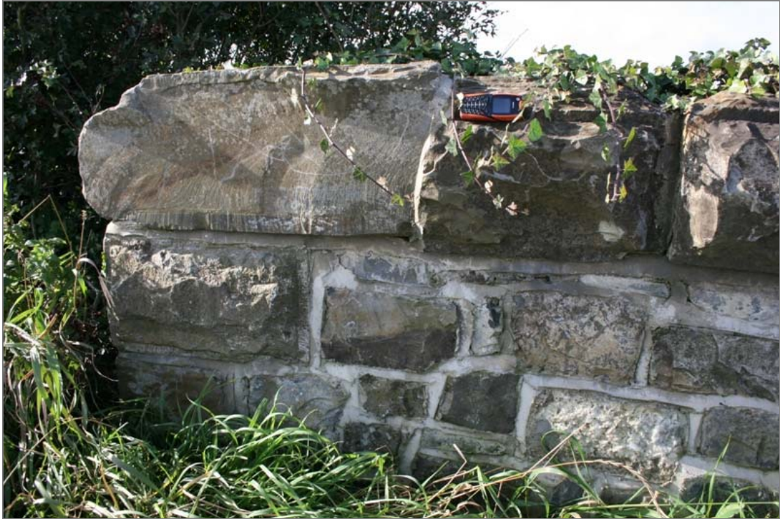
FHBS-03-BH-05 ~ Repaired west parapet
