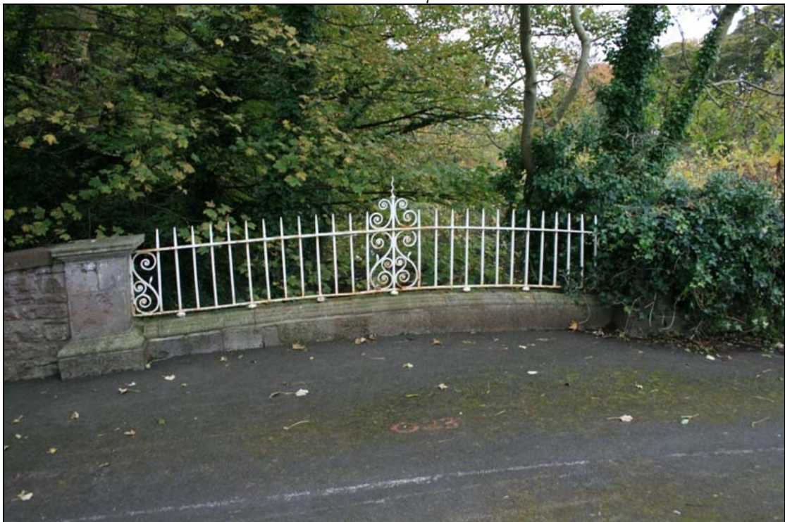
FHBS-09-BH-03 ~ West parapet from path
