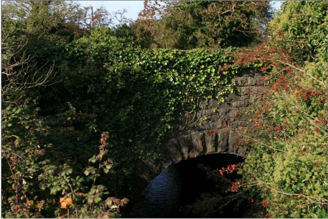
FHBS-04-BH-02 ~ East downstream elevation
