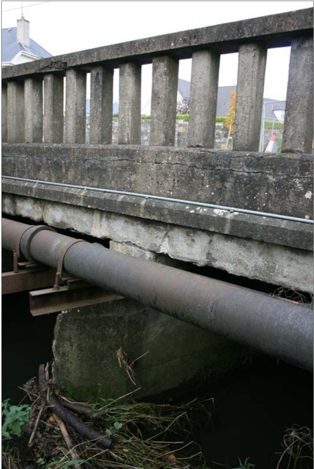
FHBS-06-BH-03 ~ West parapet from upstream
