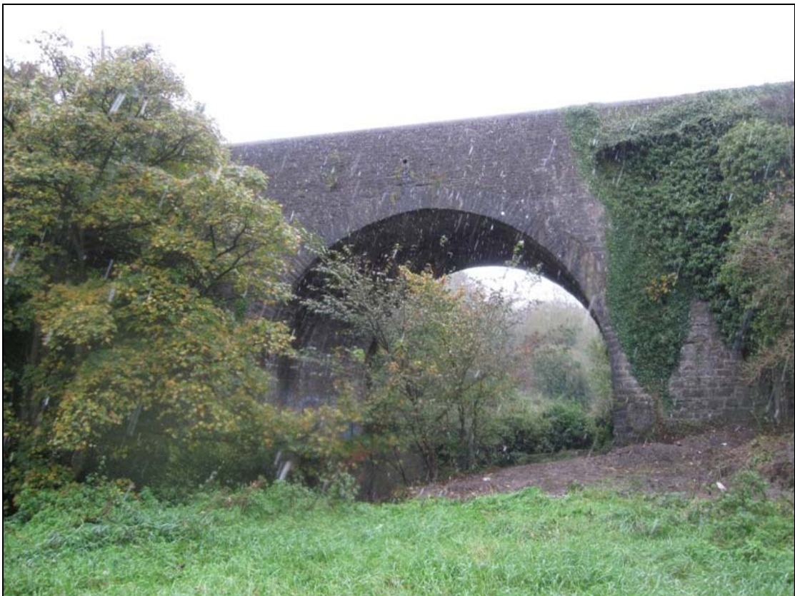
FHBS-11-NH-05 ~ Knocksedan bridge downstream parapet walls
