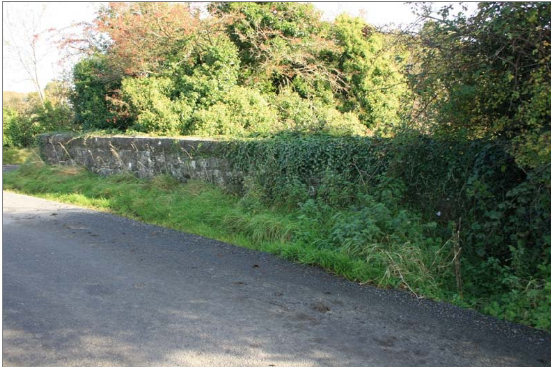
FHBS-04-BH-04 ~ East parapet from road
