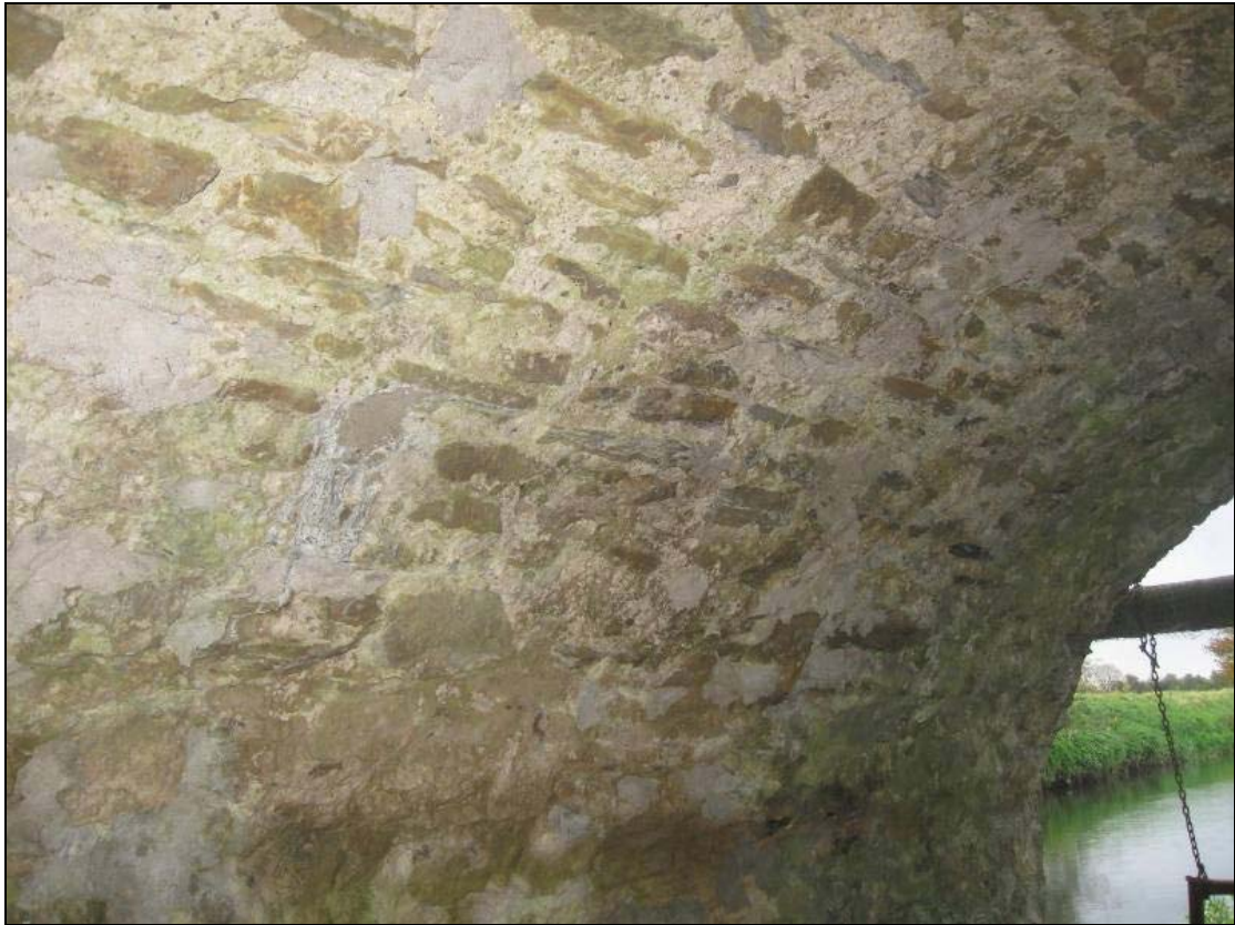
FHBS-08-NH-03 ~ Repointed bridge underarch
