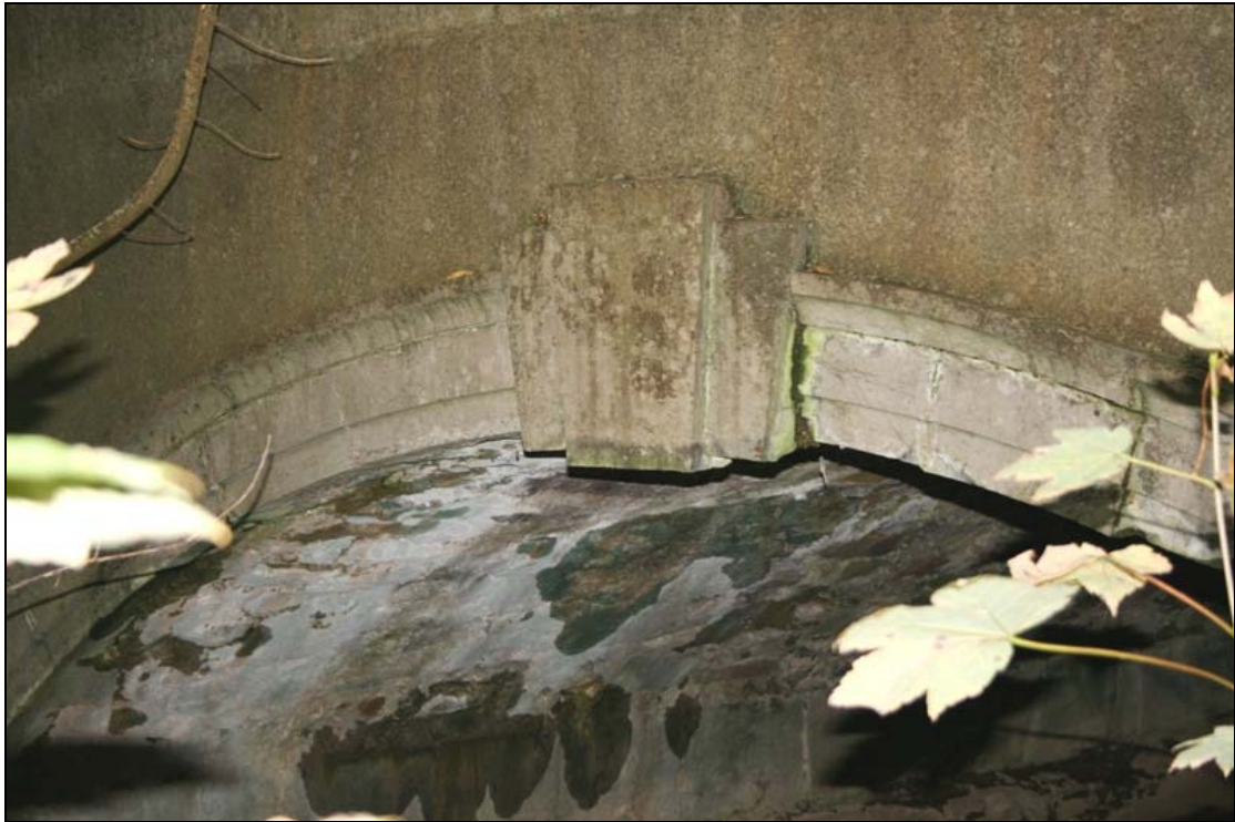
FHBS-09-BH-06 ~ Carved limestone archivolt and keystone on west elevation
