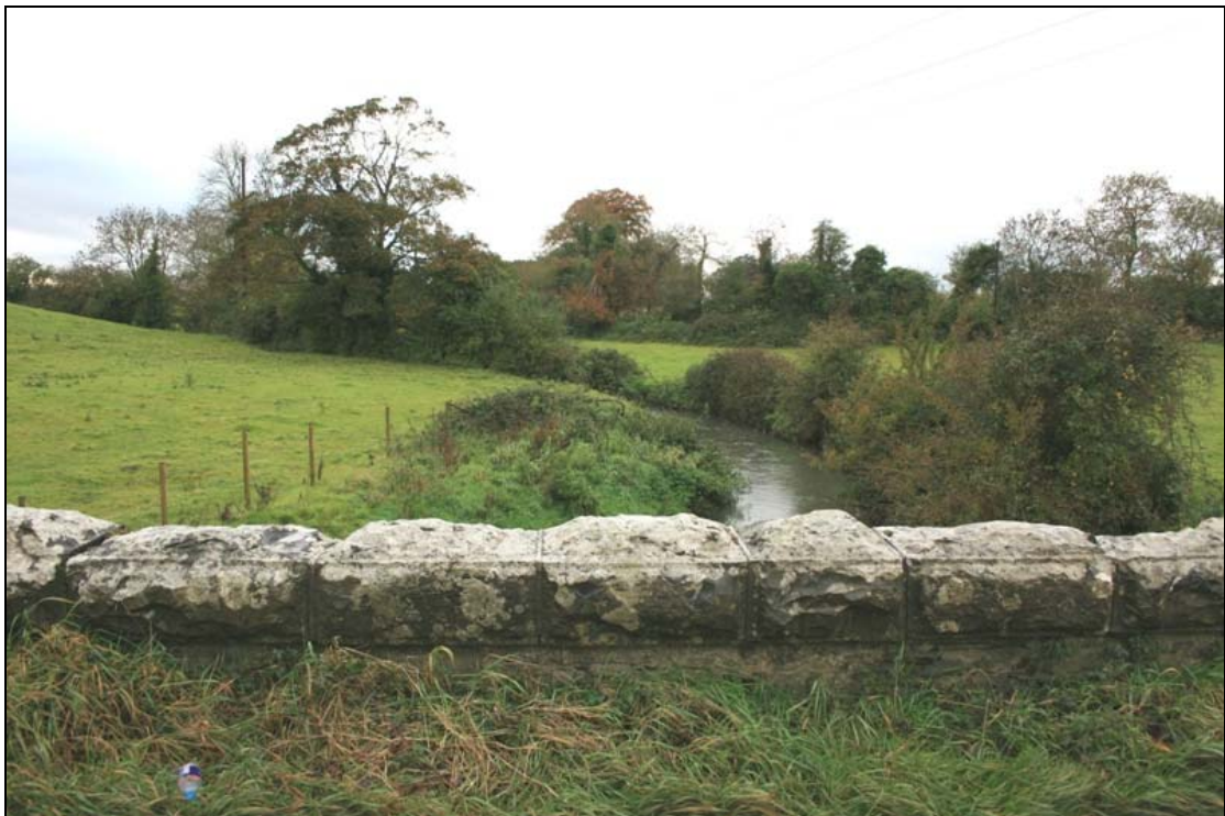
FHBS-12-BH-09 ~ View upstream to west
