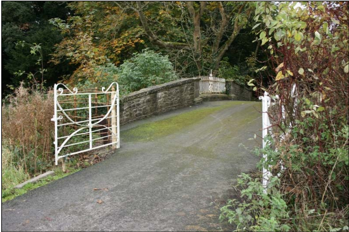
FHBS-09-BH-08 ~ View over bridge from north
