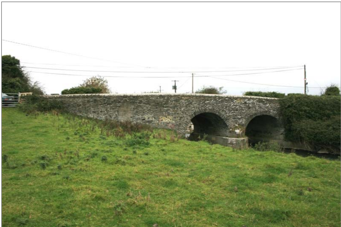
FHBS-07-BH-02 ~ East downstream elevation
