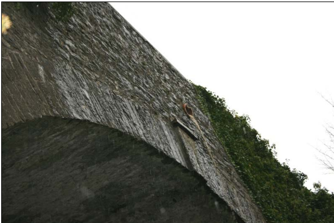
FHBS-11-BH-09 ~ Road drainage through west parapet
