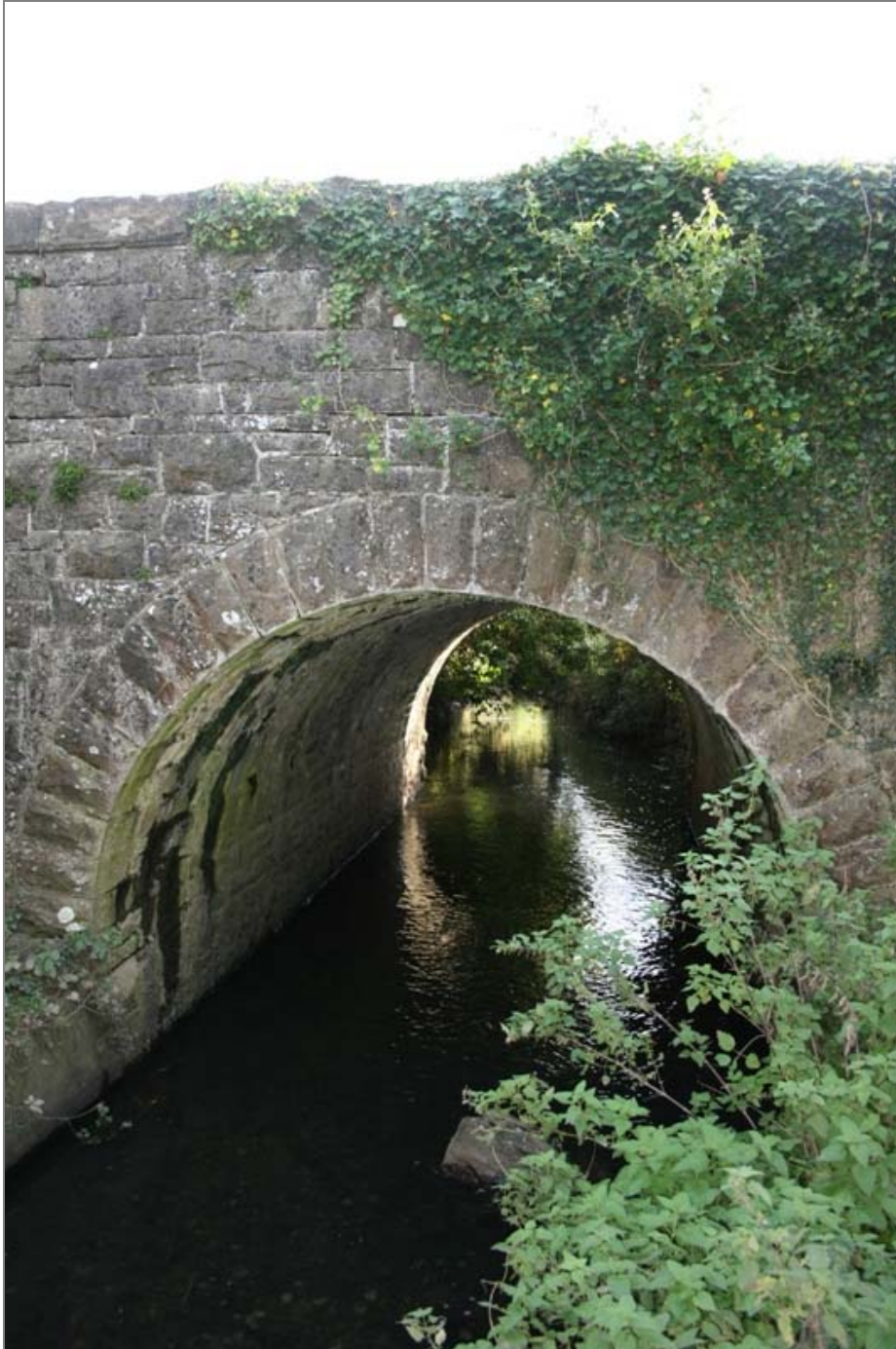
FHBS-04-BH-01 ~ West upstream elevation
