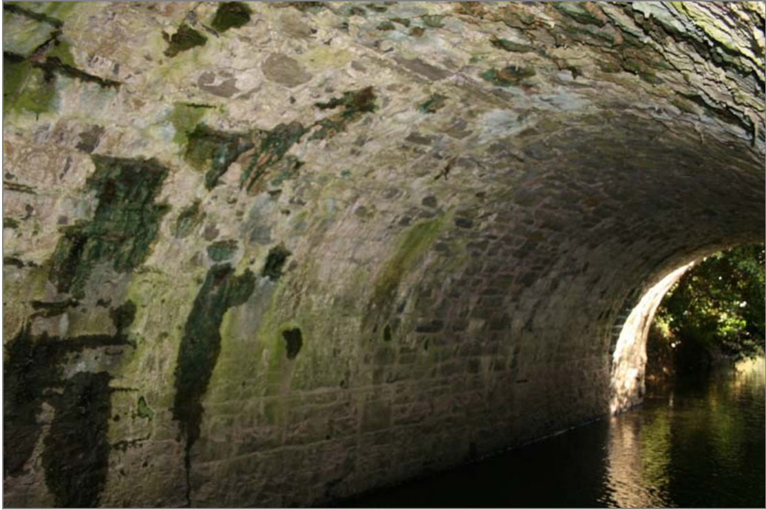
FHBS-04-BH-07 ~ Soffit of southern arch from east
