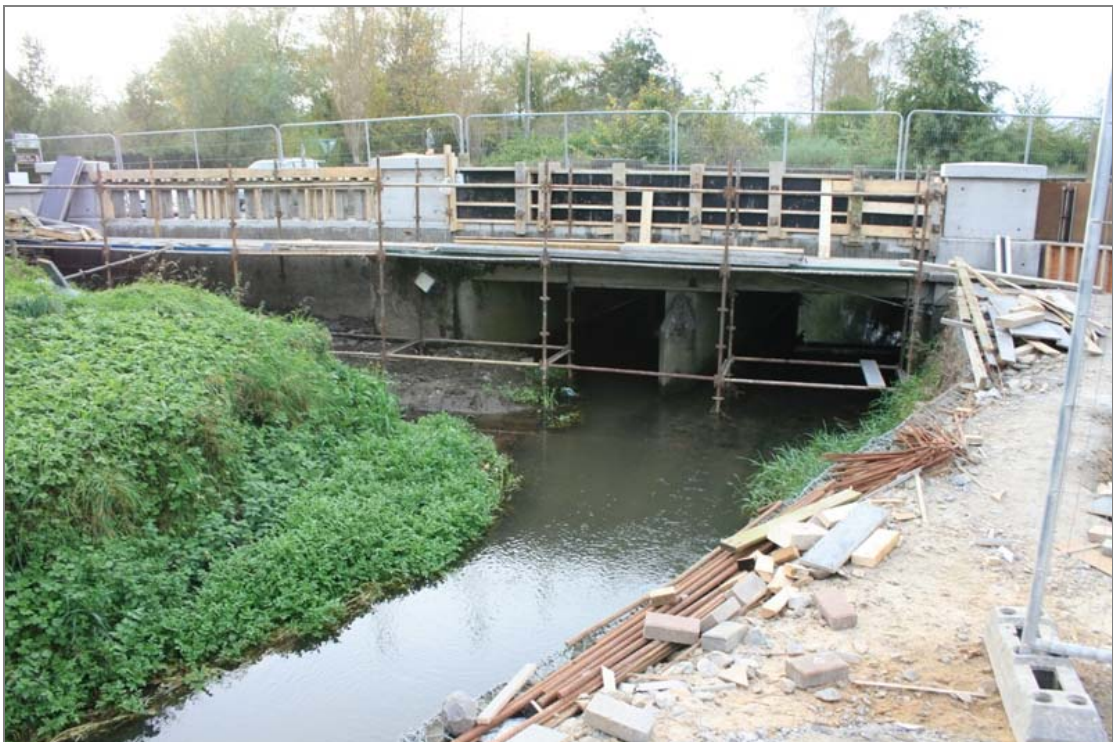
FHBS-06-BH-02 ~ East downstream elevation
