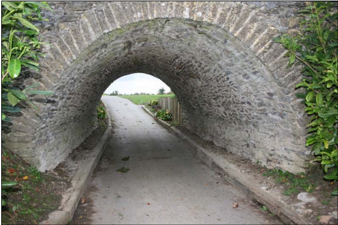
FHBS-08-BH-07 ~ Dry arch on southern bank from eastern side
