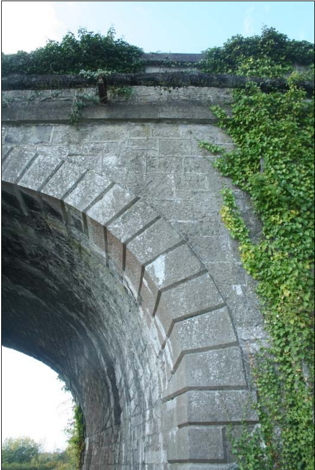
FHBS-15-BH-13 ~ Detail of north east corner of rail bridge
