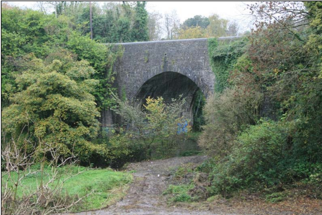
FHBS-11-BH-01 ~ East downstream elevation
