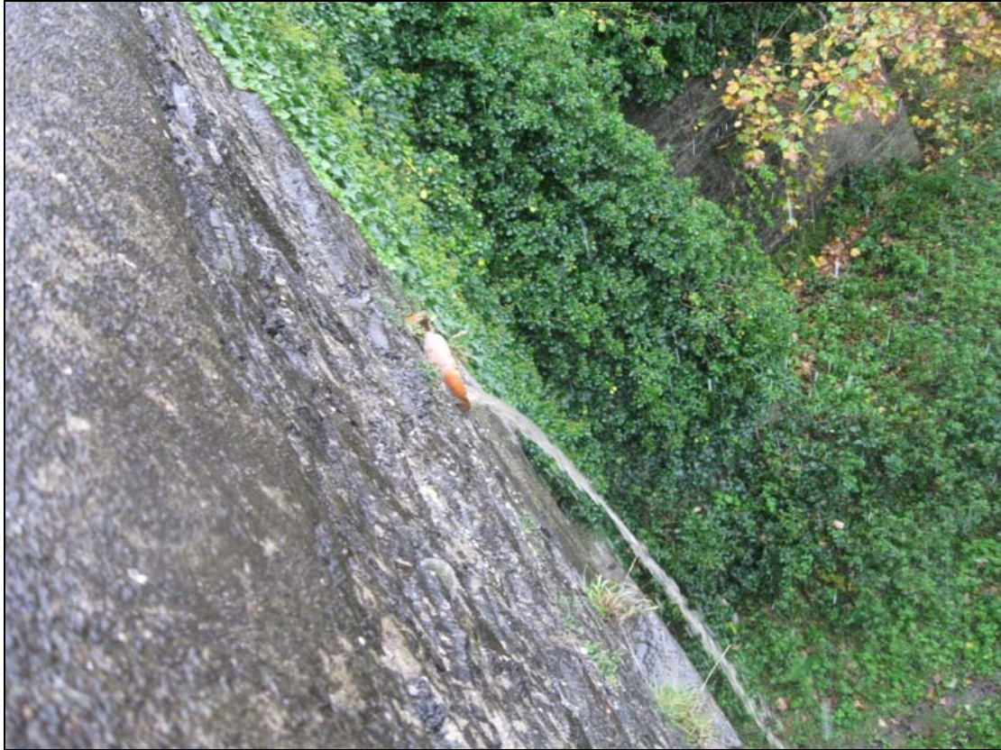
FHBS-11-NH-01 ~ Bridge drainage on upstream parapet wall
