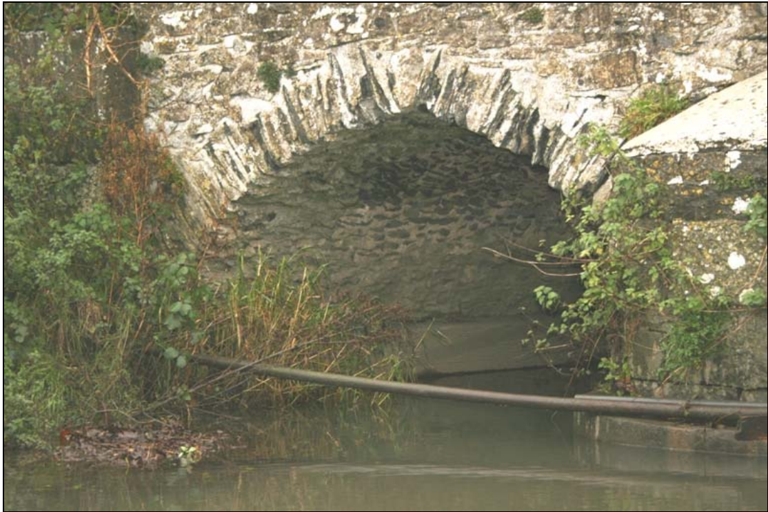
FHBS-12-BH-08 ~ Northern arch from west
