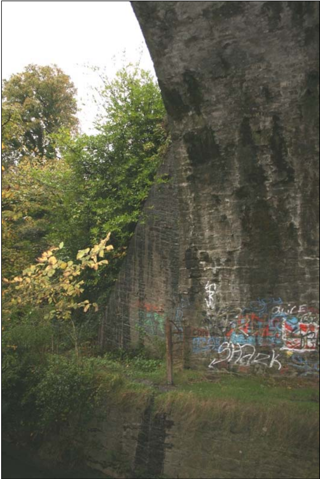
FHBS-11-BH-11 ~ South east corner of bridge with iron pedestrian gate
