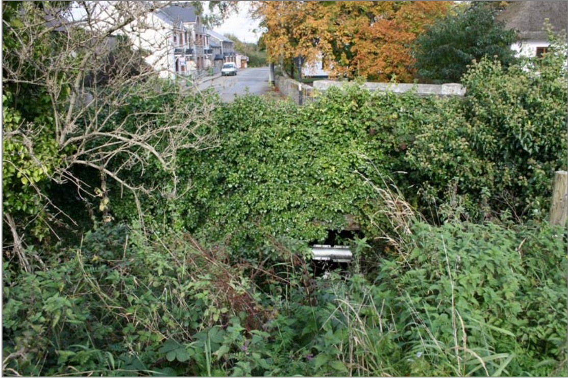
FHBS-05-BH-01 ~ South upstream elevation
