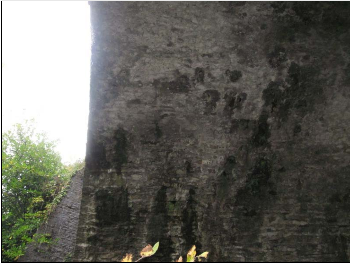
FHBS-11-NH-02 ~ Bridge underarch
