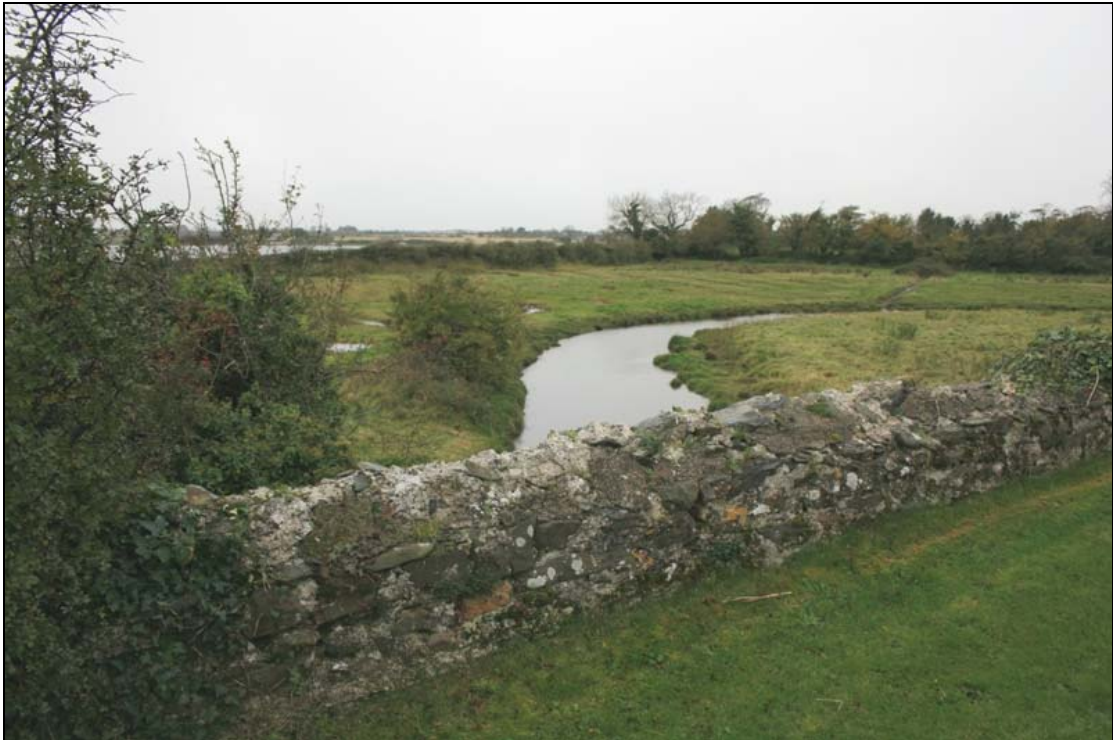
FHBS-10-BH-03 ~ South parapet from top of bridge
