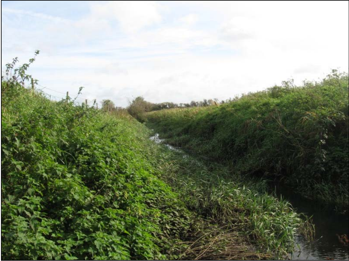
FHBS-03-NH-03 ~ Scarcity of connectivity within bridge environs
