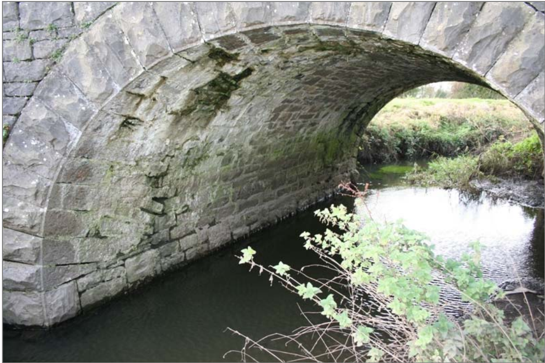
FHBS-03-BH-07 ~ Soffit of arch from east
