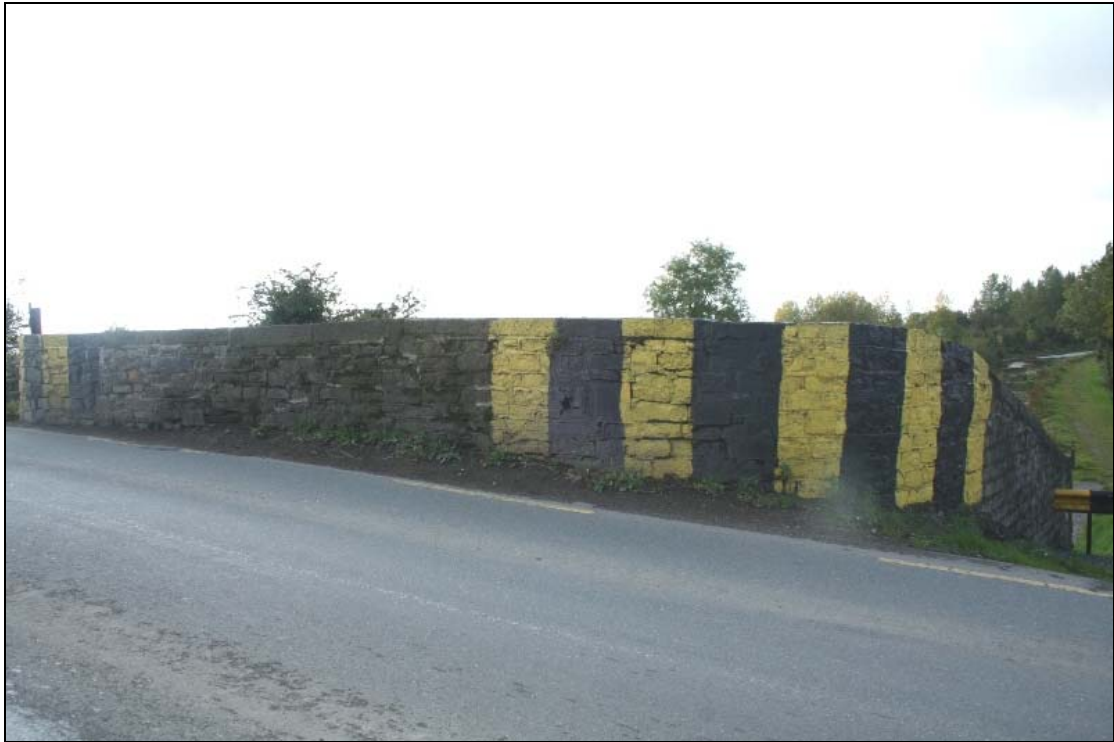
FHBS-15-BH-03 ~ West parapet of canal bridge from road
