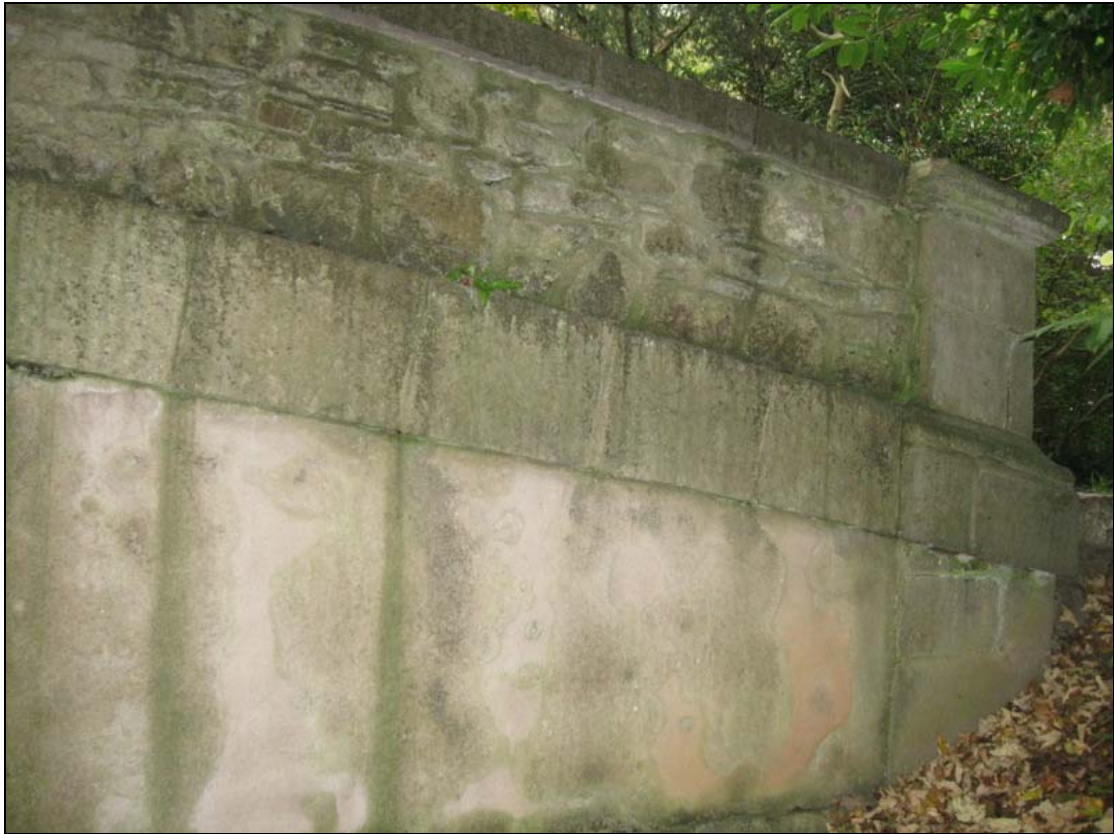
FHBS-09-NH-03 ~ Parapet bridge walls
