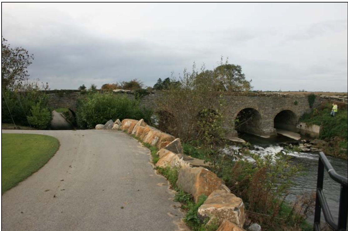
FHBS-08-BH-02 ~ East downstream elevation
