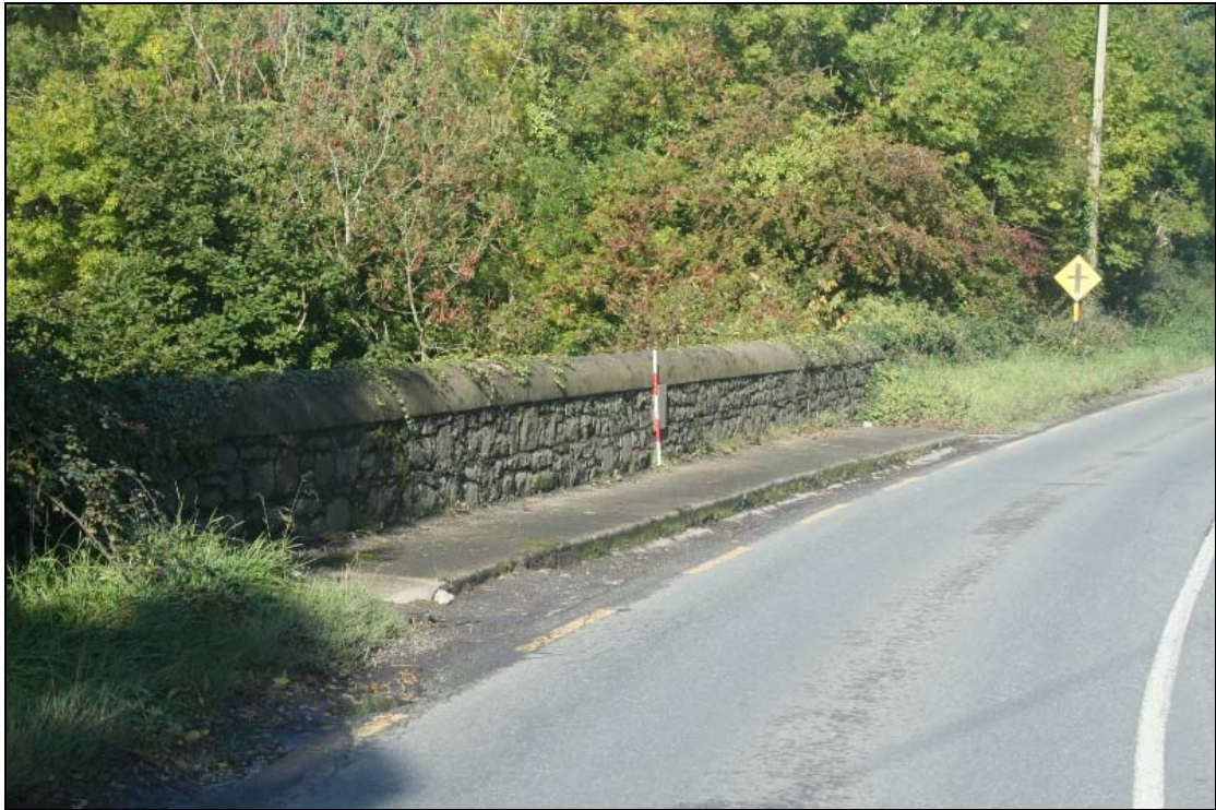
FHBS-11-BH-05 ~ West parapet from road
