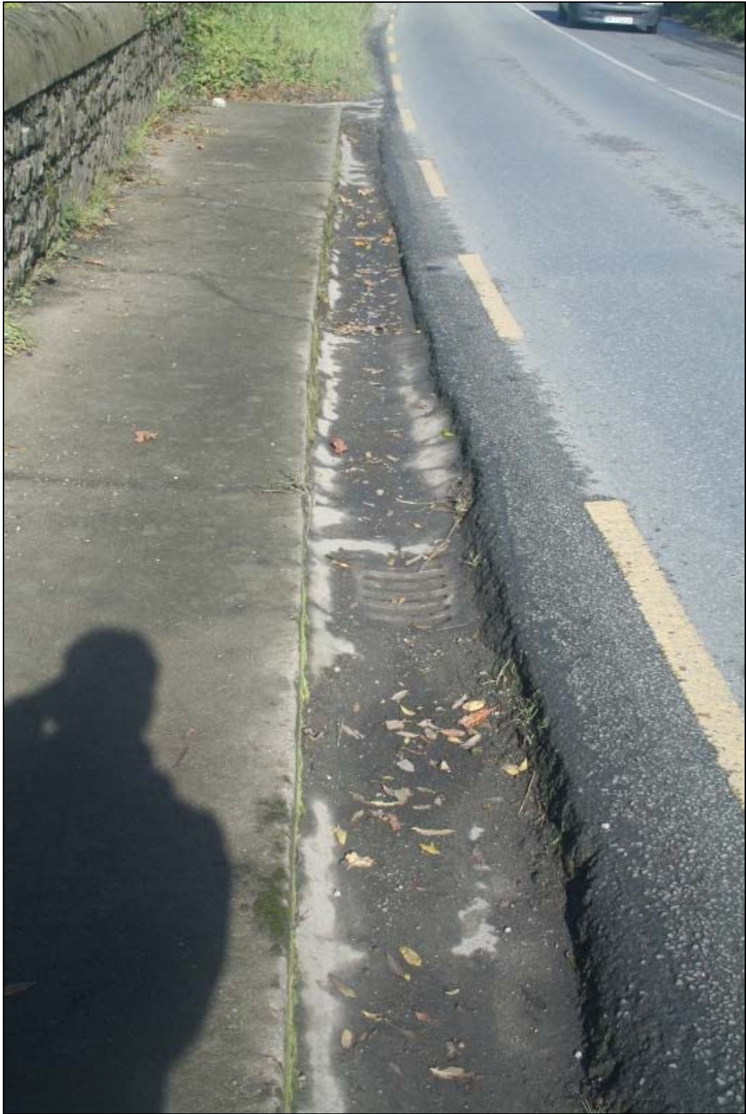
FHBS-11-BH-07 ~ Detail of road drainage beside footpath on west parapet
