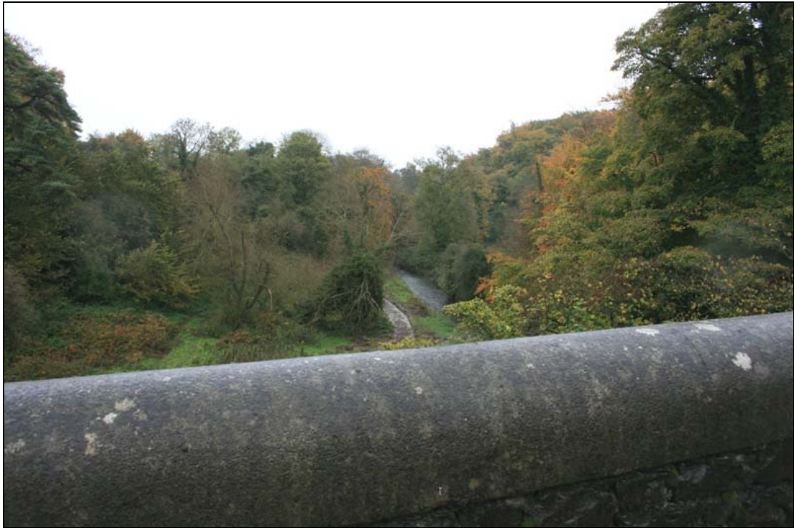
FHBS-11-BH-14 ~ View downstream over east parapet wall
