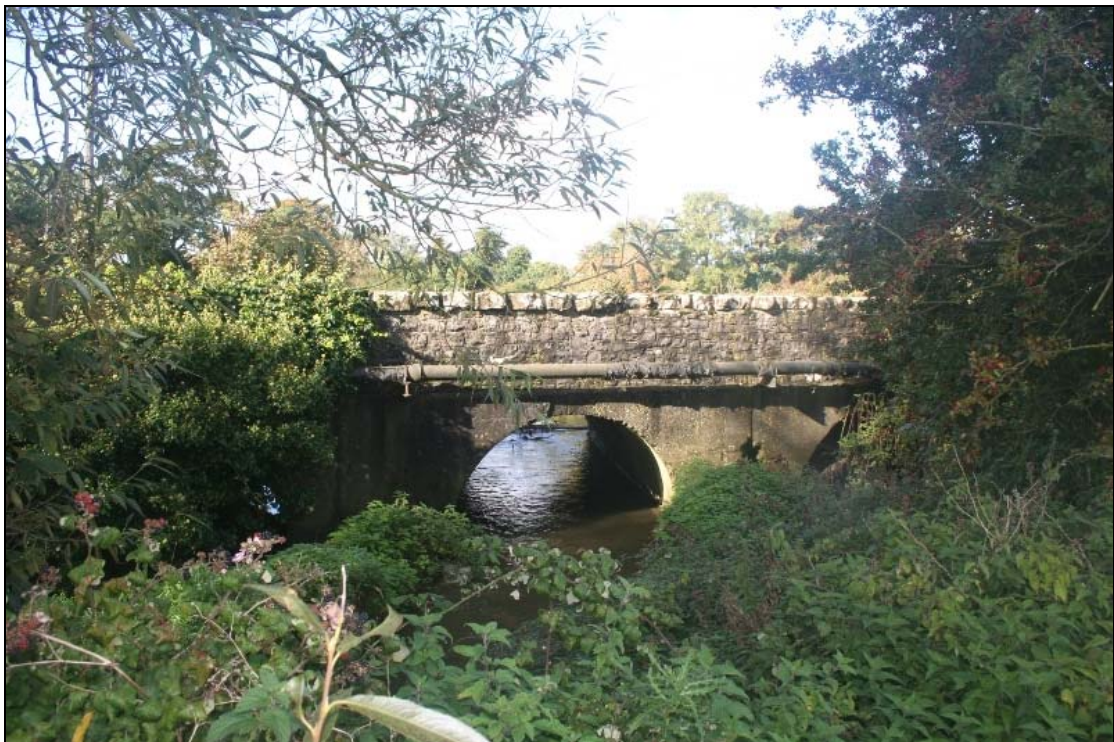
FHBS-12-BH-02 ~ East downstream elevation
