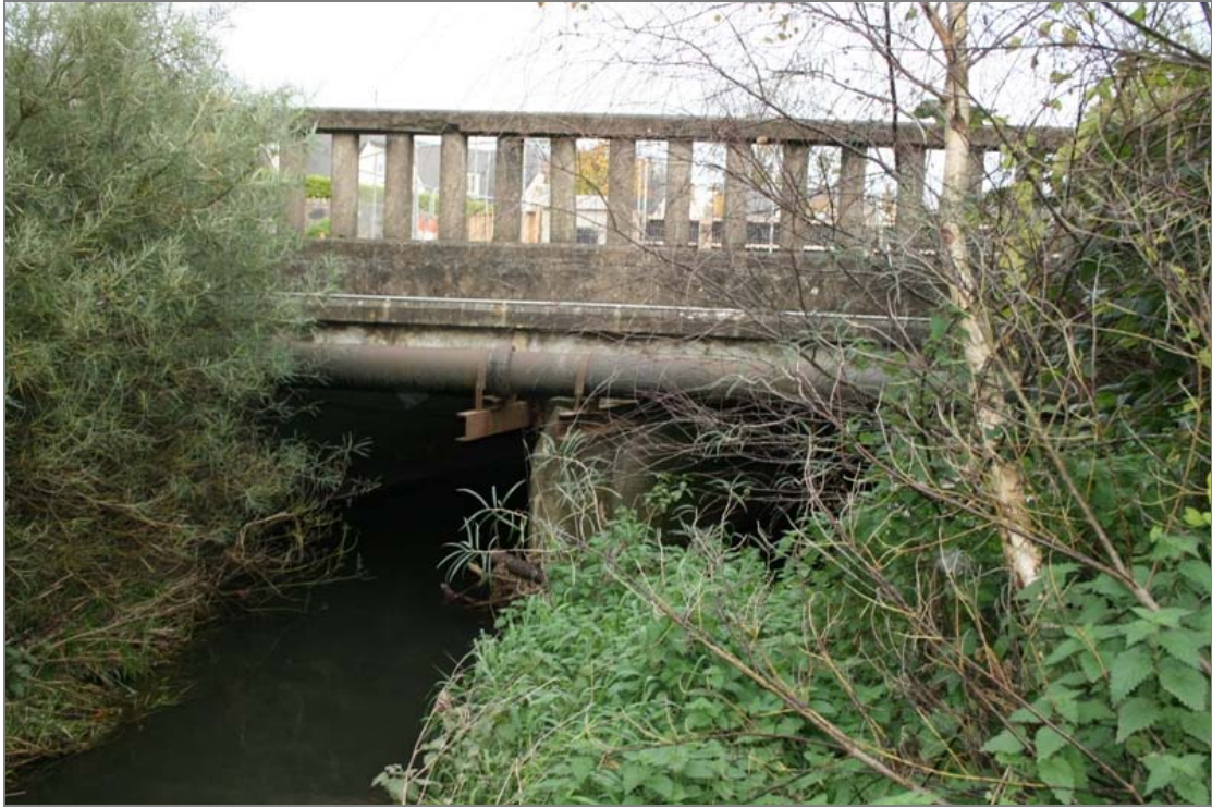
FHBS-06-BH-01 ~ West upstream elevation
