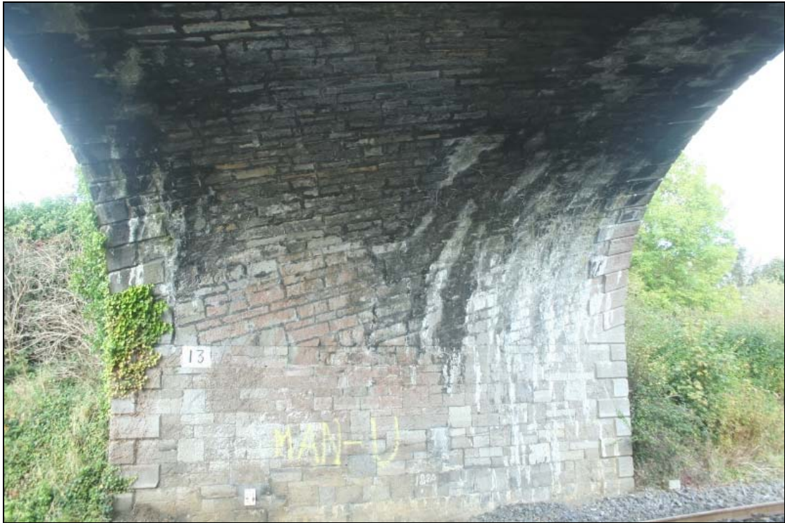
FHBS-15-BH-14 ~ South side of rail bridge's skewed arch soffit
