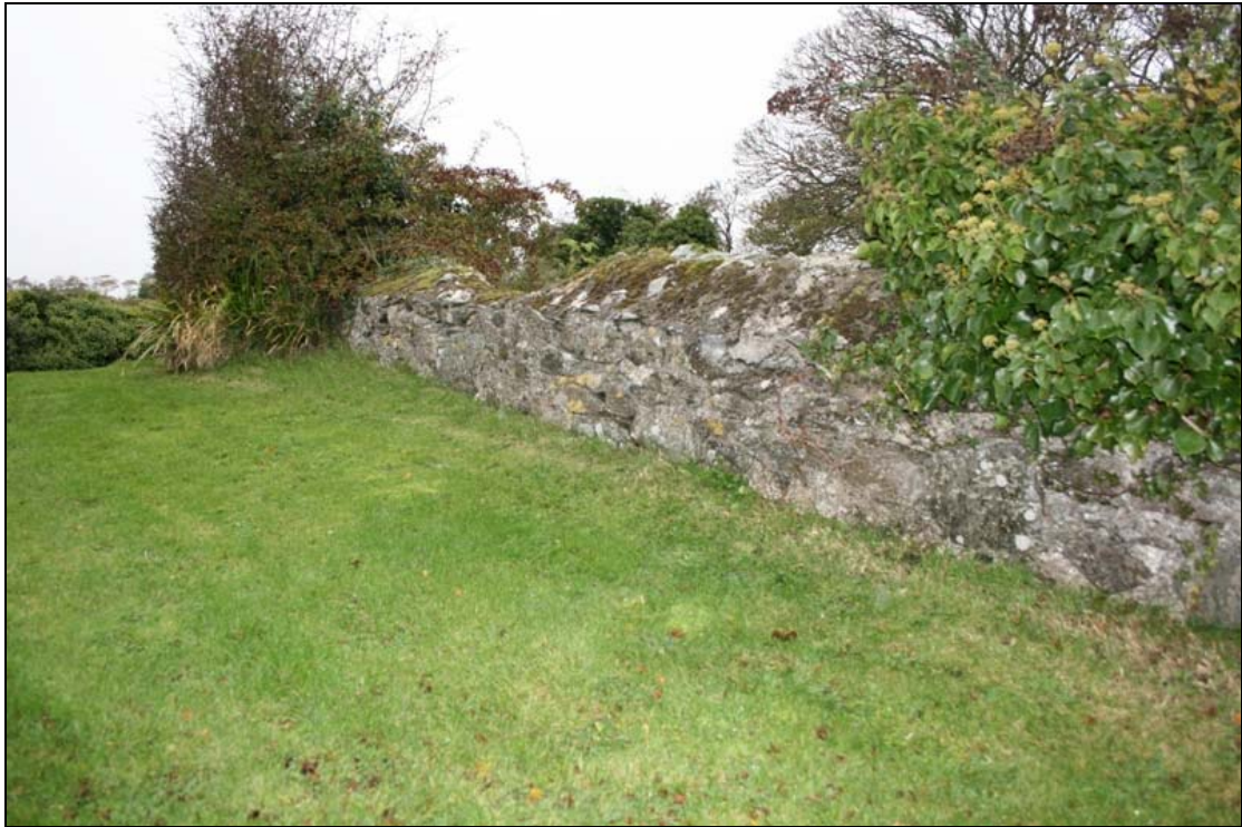
FHBS-10-BH-04 ~ North parapet from top of bridge
