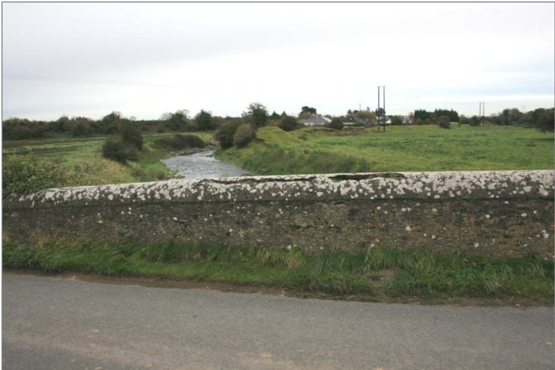
FHBS-07-BH-04 ~ East parapet from road
