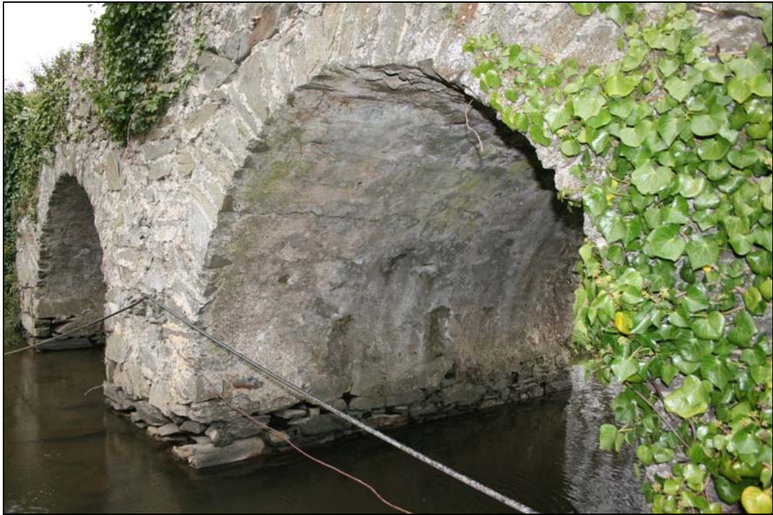
FHBS-10-NH-03 ~ Bridge underarch - restricted bat potential
