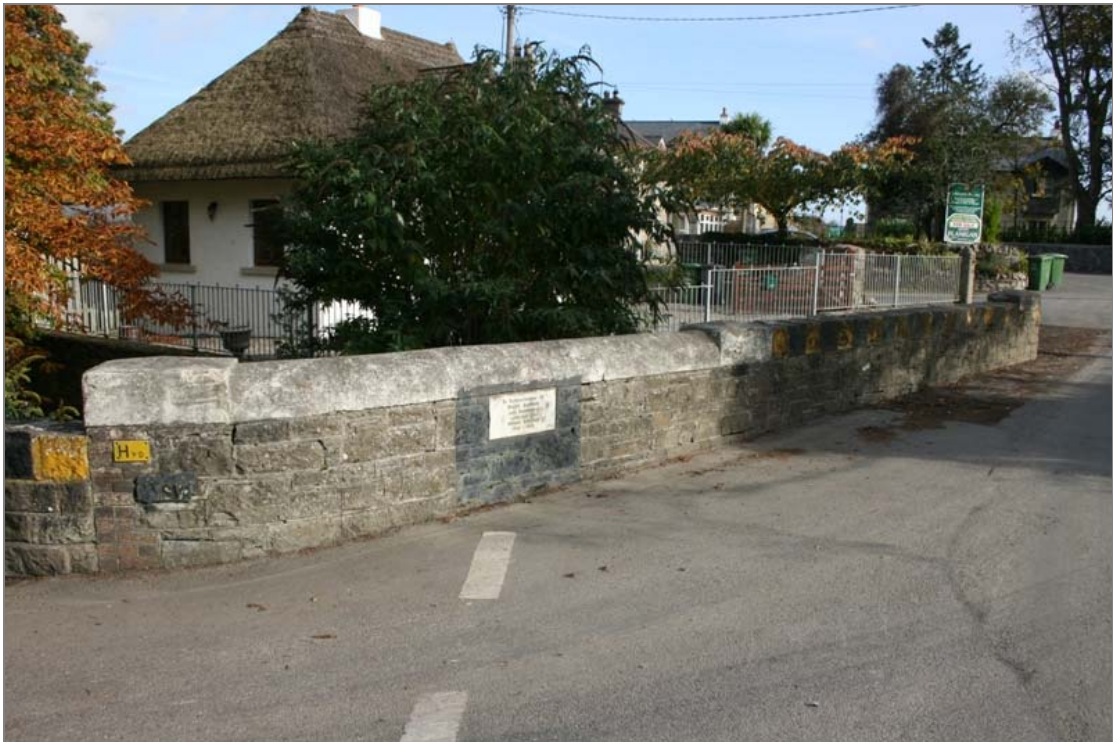
FHBS-05-BH-04 ~ North parapet from road
