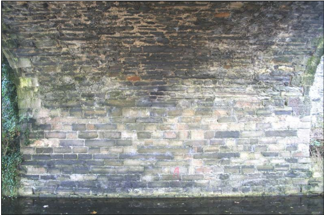
FHBS-14-BH-07 ~ South side of arch soffit
