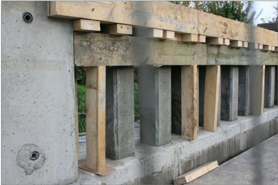
FHBS-06-BH-06 ~ Replacement, reinforced cast concrete balusters to east parapet.
