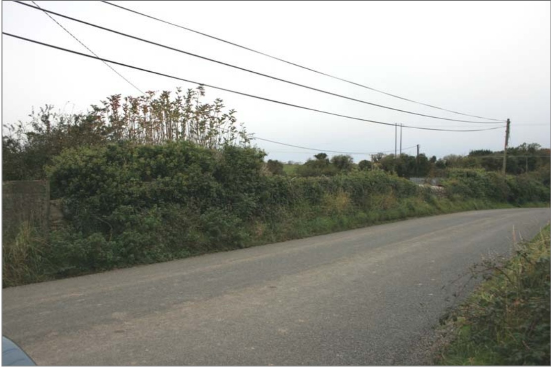
FHBS-07-BH-03 ~ West parapet from road
