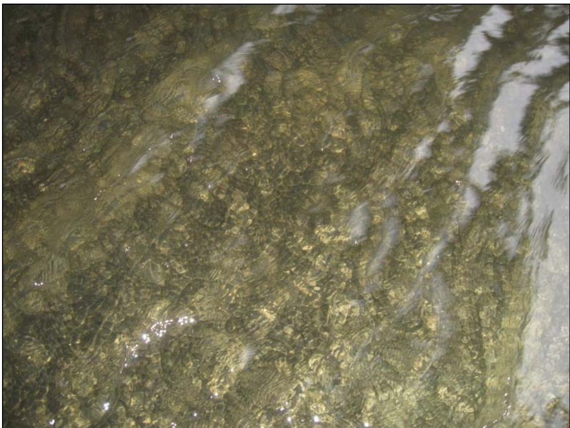
FHBS-07-NH-02 ~Concrete substrate underneath bridge arch
