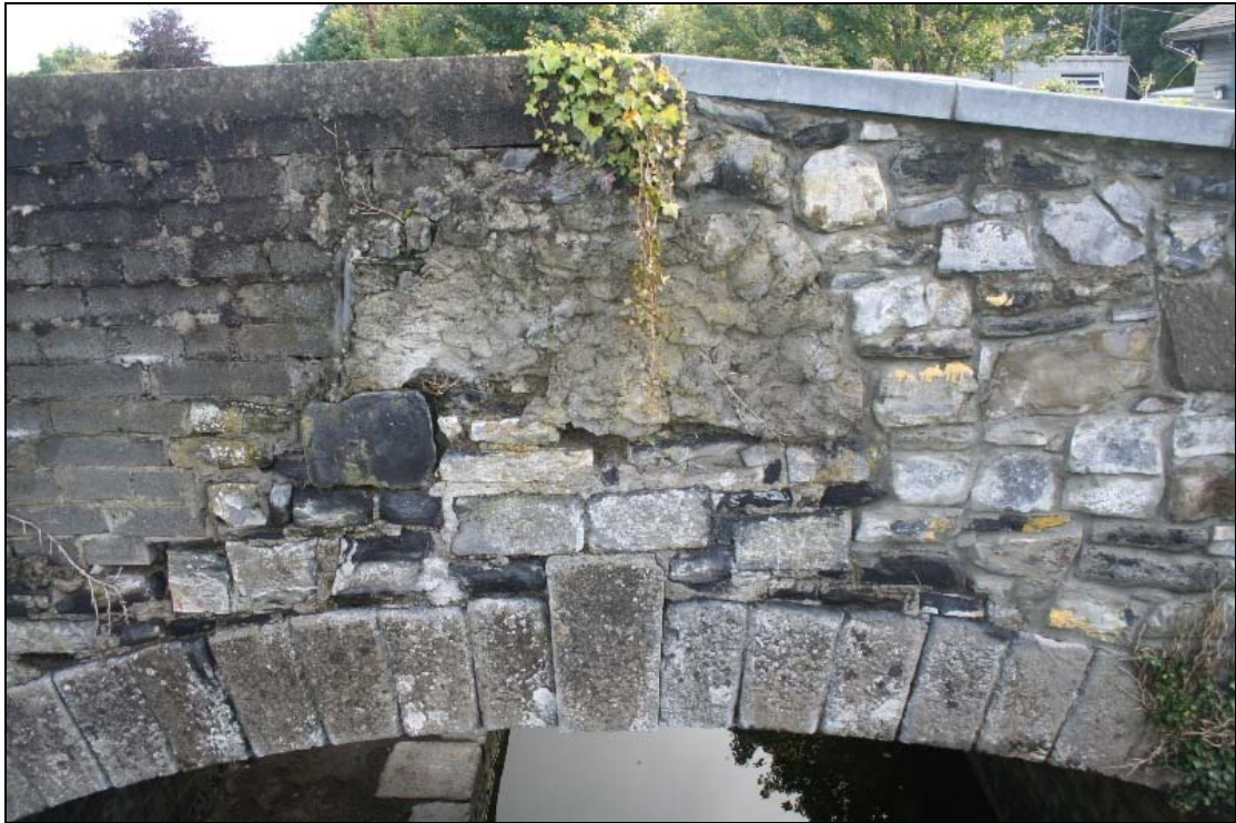
FHBS-14-BH-05 ~ Apex of west elevation showing variety of repair materials
