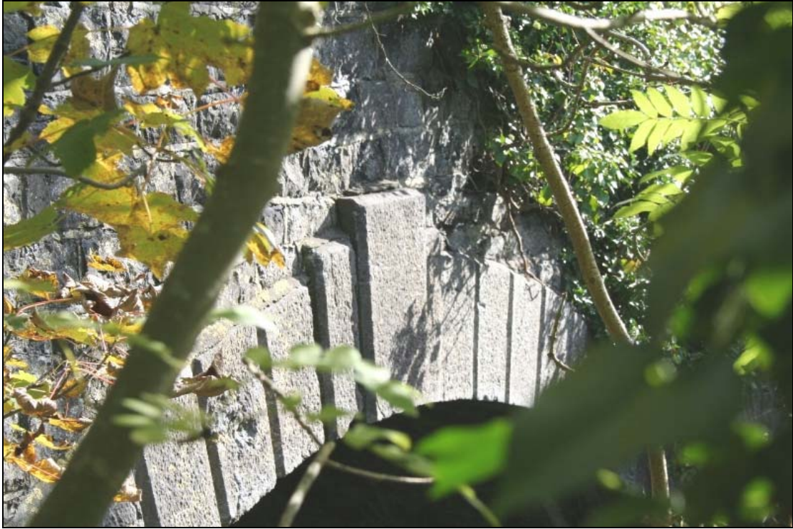
FHBS-13-BH-05 ~ Detail of ashlar voussoirs and keystone on west elevation
