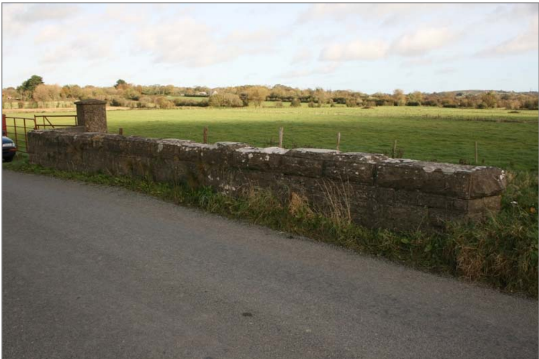
FHBS-03-BH-04 ~ East parapet from road
