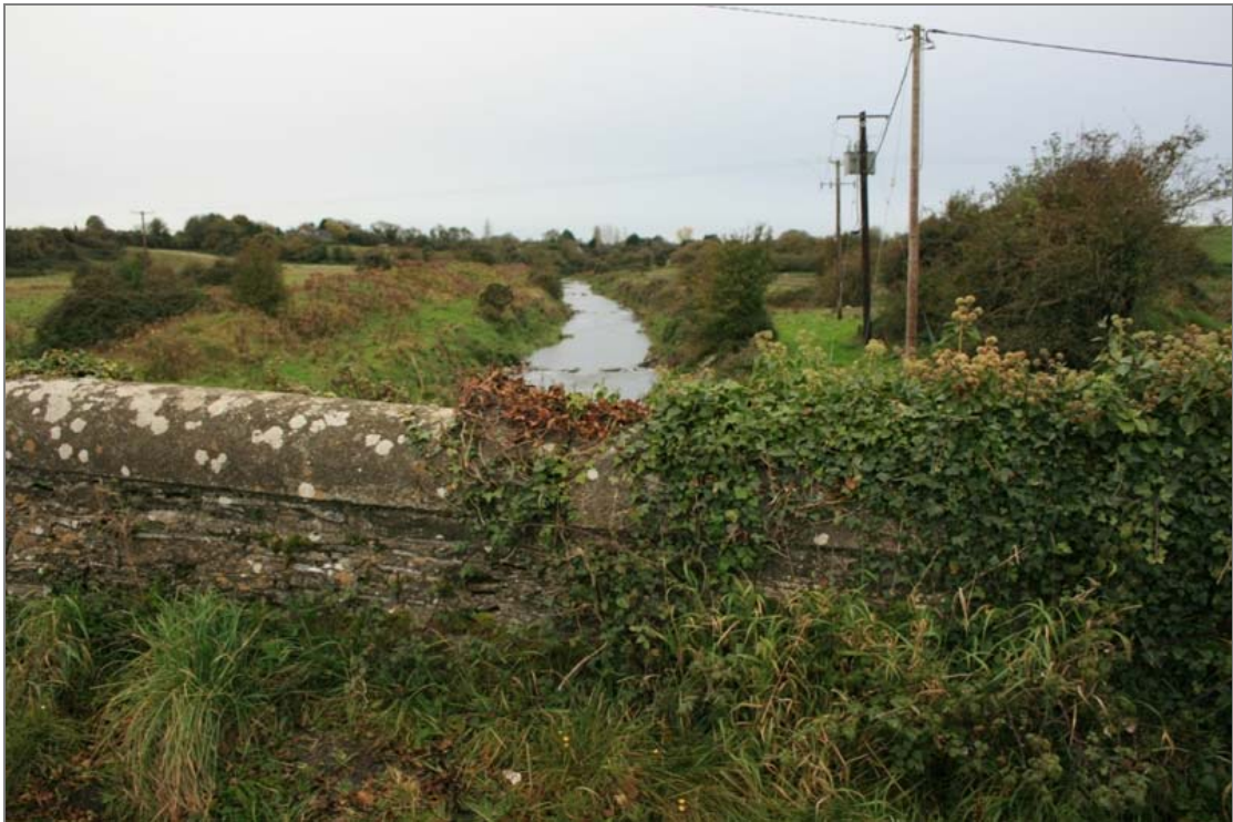
FHBS-07-BH-08 ~ View upstream to west
