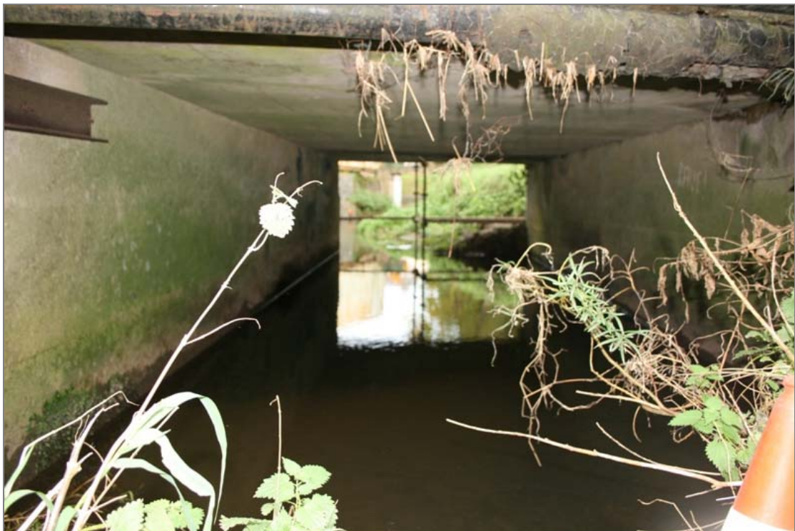
FHBS-06-BH-07 ~ Soffit of southern arch from west
