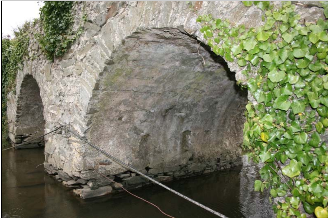
FHBS-10-BH-06 ~ Soffit of eastern arch from south
