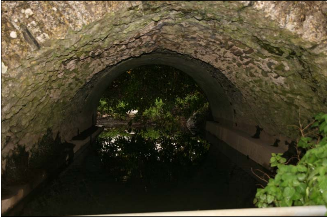
FHBS-12-NH-01 ~ Bridge underarch - northerly underarch
