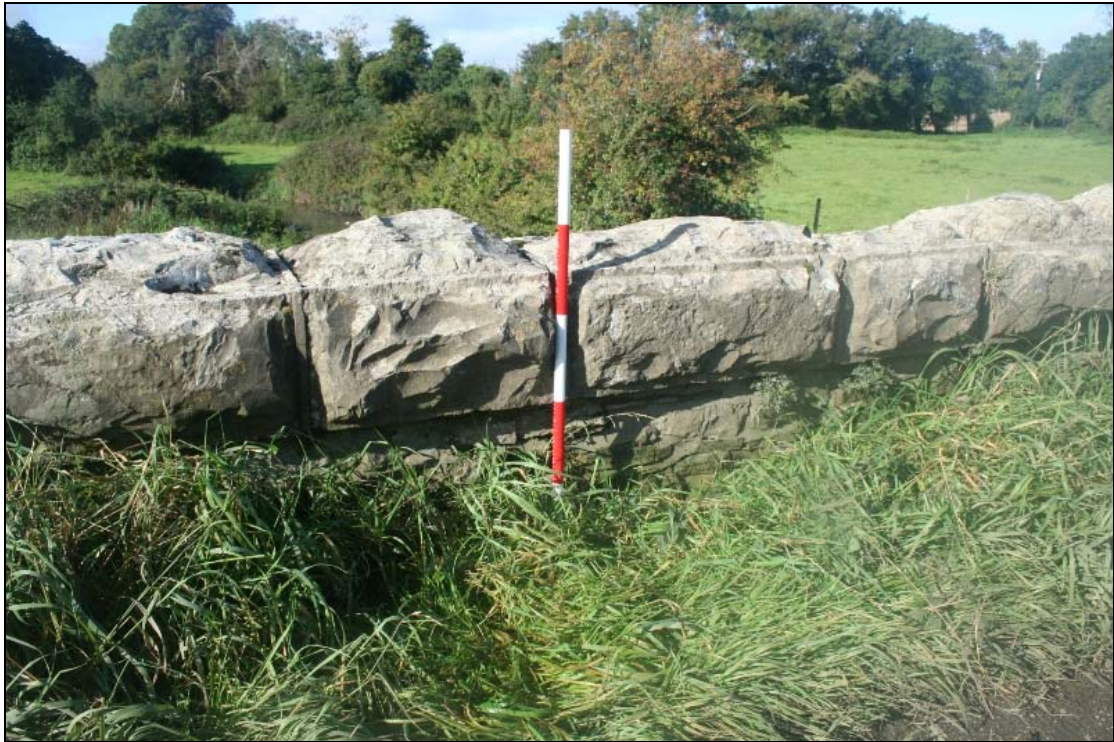
FHBS-12-BH-03 ~ West parapet from road
