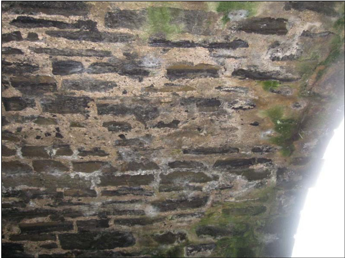
FHBS-15-NH-01 ~ Bridge underarch
