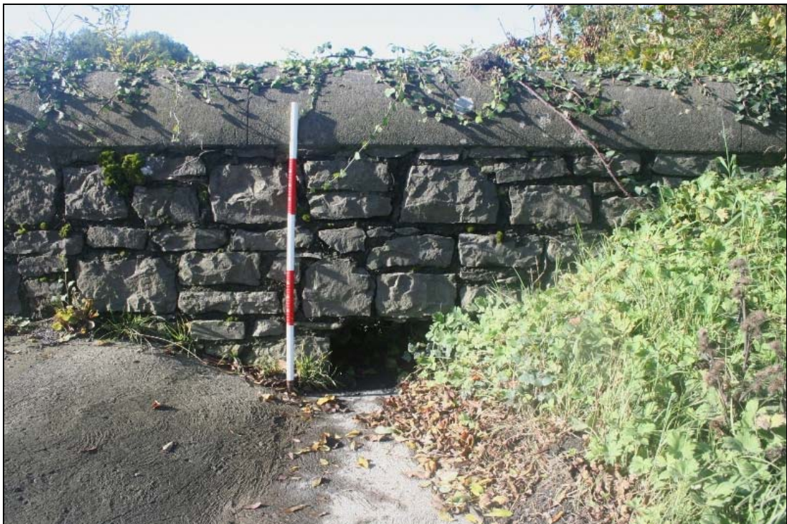
FHBS-11-BH-06 ~ Detail of west parapet masonry and road drainage duct
