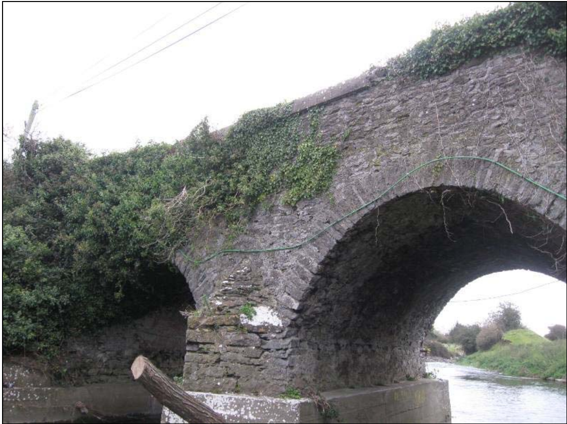
FHBS-07-NH-03 ~ Ivy cover on downstream side of the bridge
