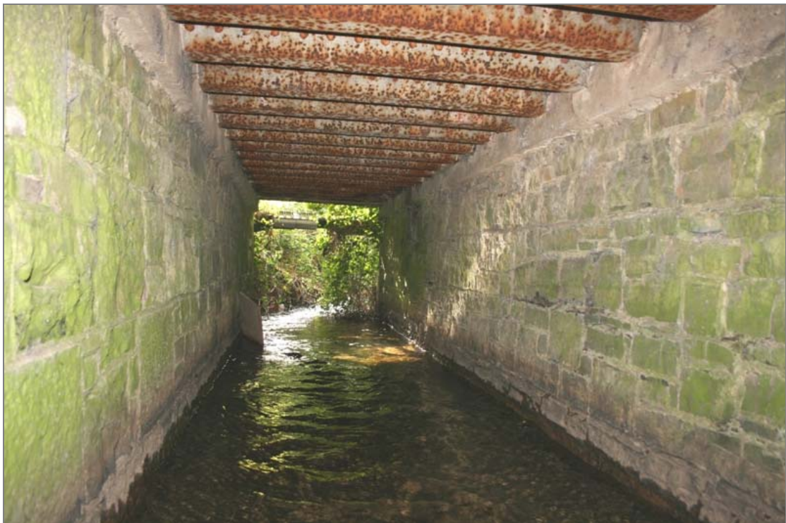
FHBS-05-BH-06 ~ Soffit of arch from north
