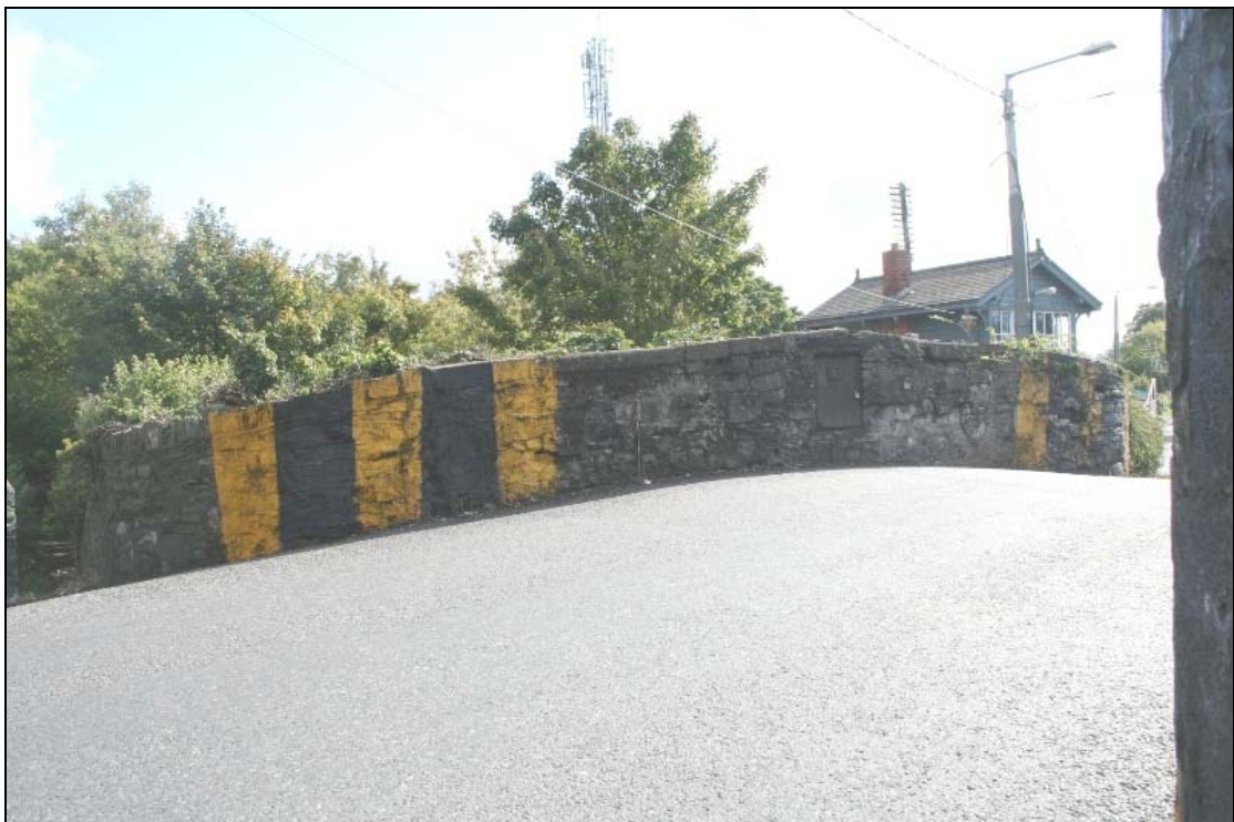
FHBS-14-BH-04 ~ East parapet from road
