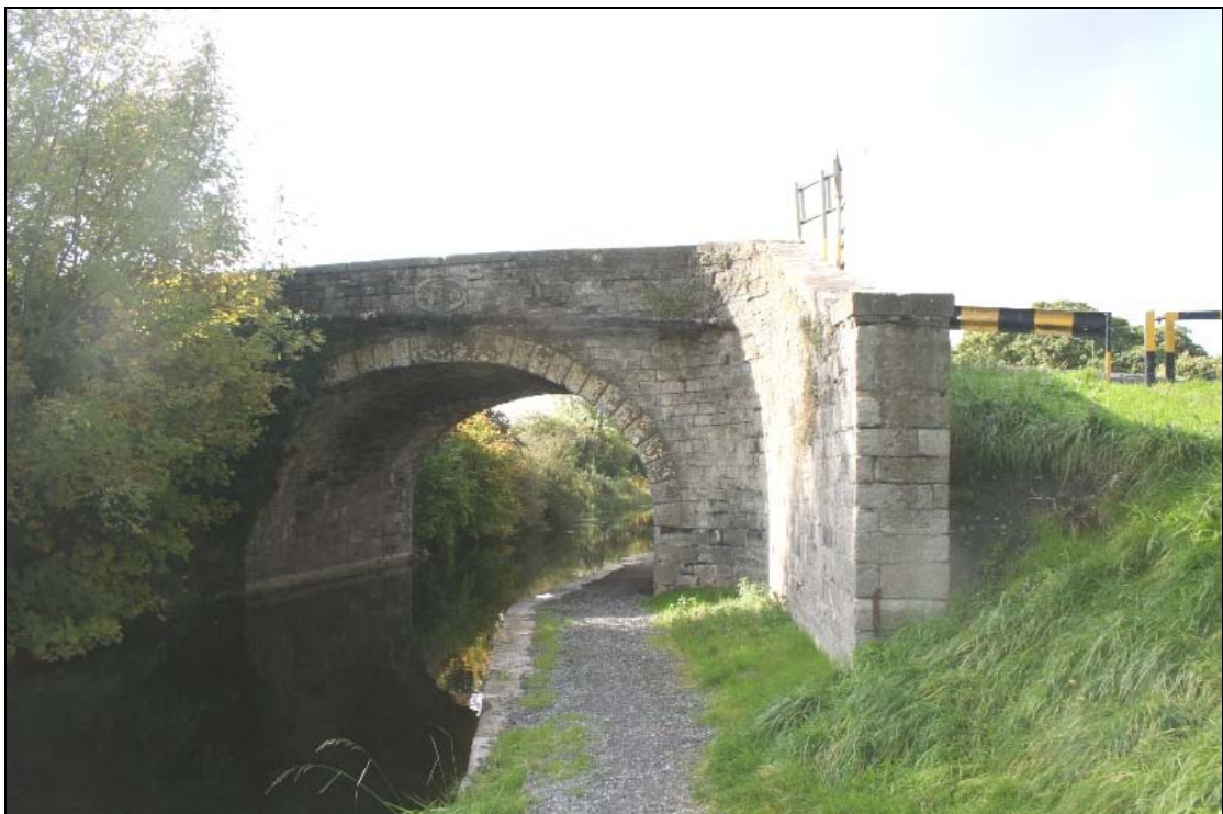
FHBS-15-BH-02 ~ East elevation of canal bridge
