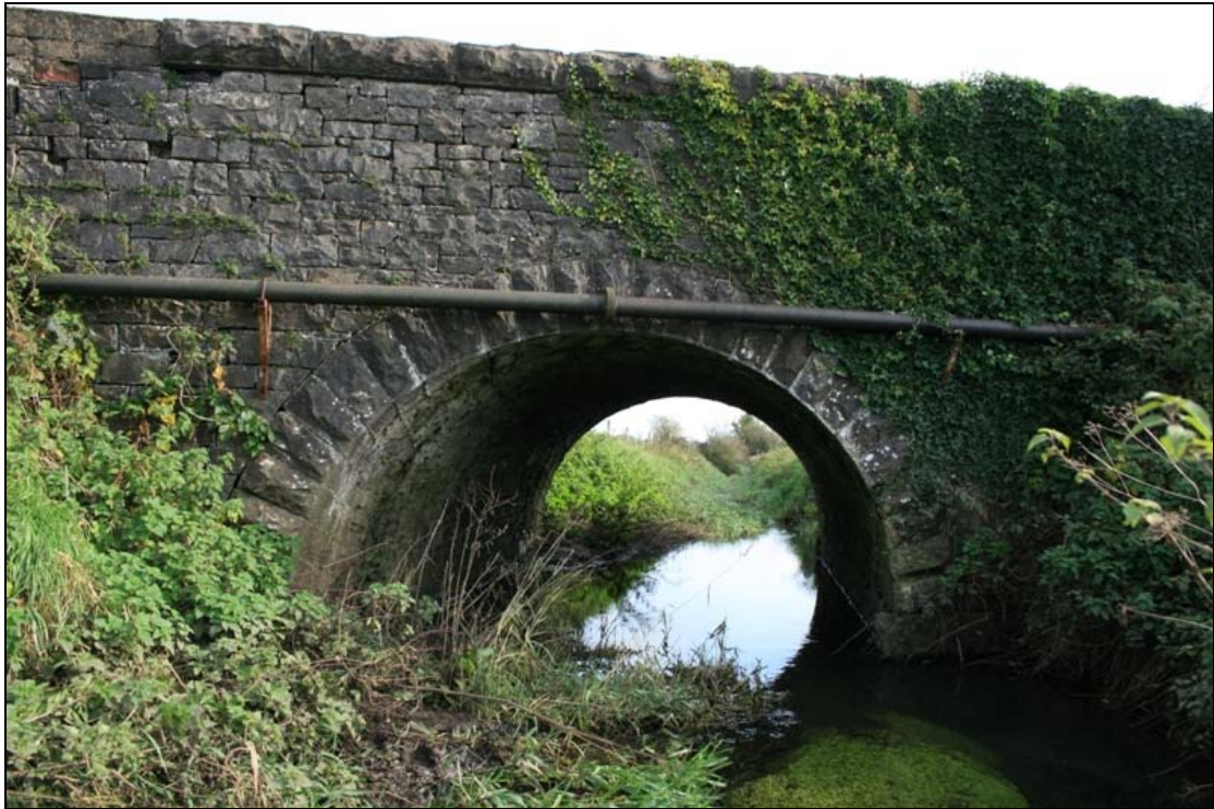
FHBS-03-BH-01 ~ West upstream elevation
