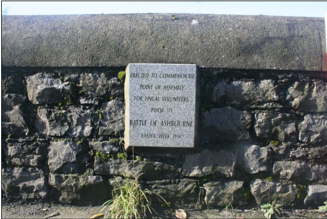
FHBS-11-BH-08 ~ Granite plaque on west parapet
