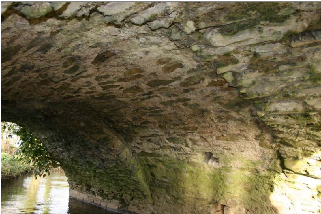
FHBS-01-BH-08 ~ Soffit of southern arch from east
