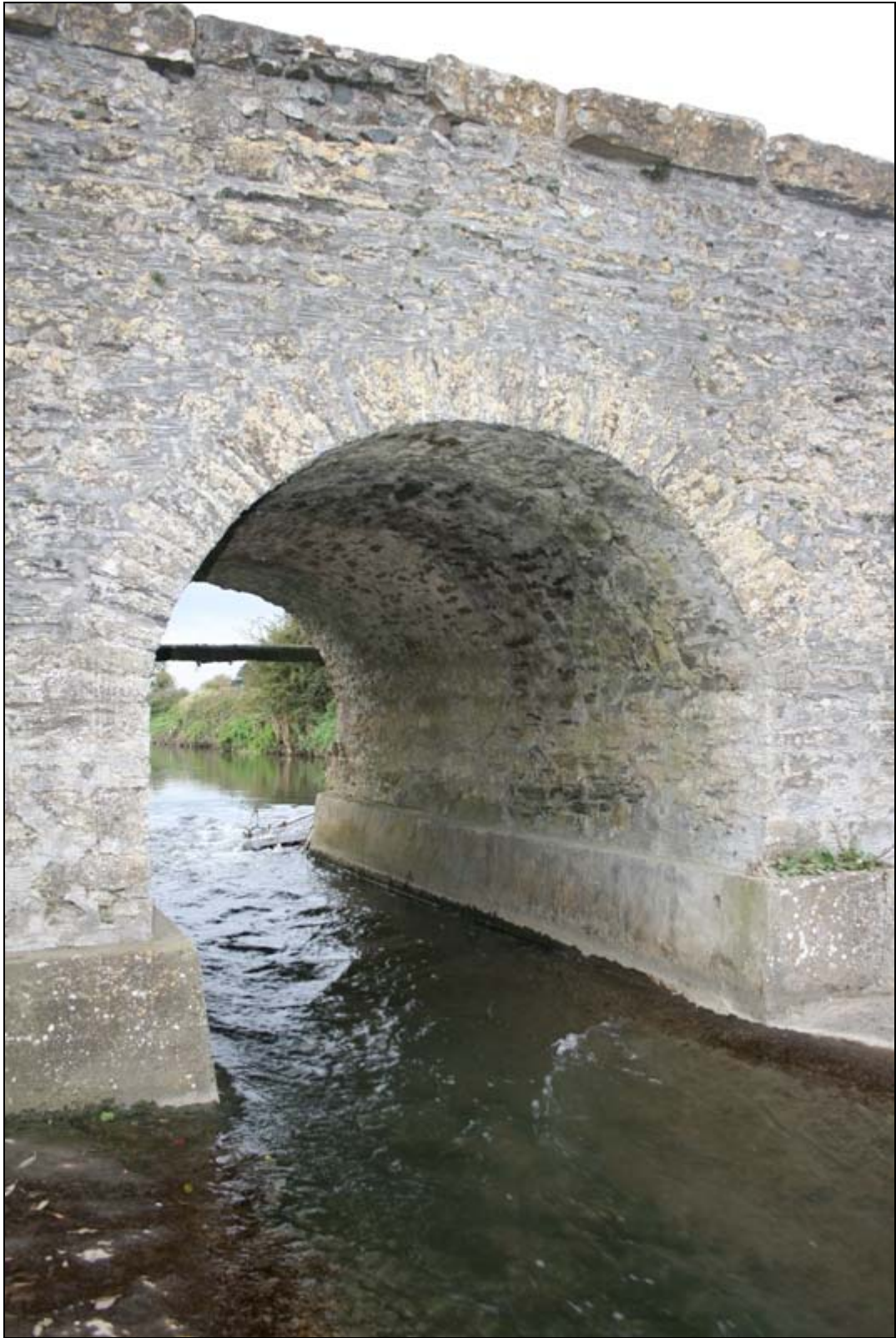
FHBS-08-BH-06 ~ Central opening of 5-arch bridge looking upstream
