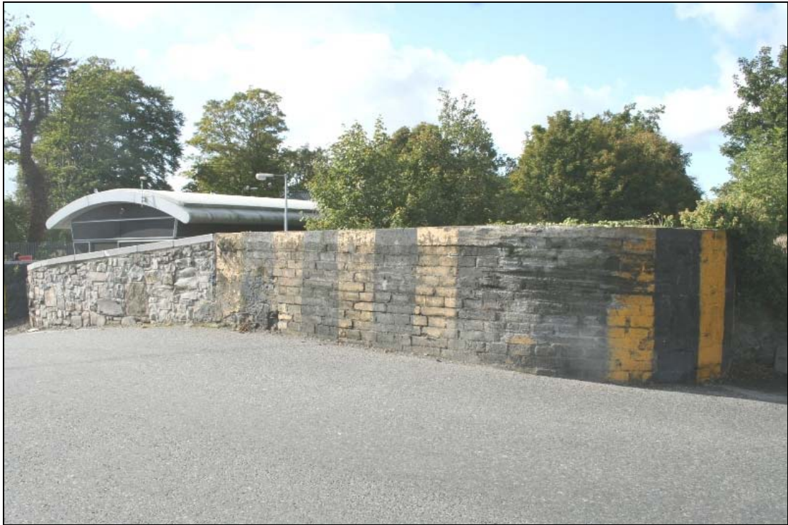
FHBS-14-BH-03 ~ West parapet from road
