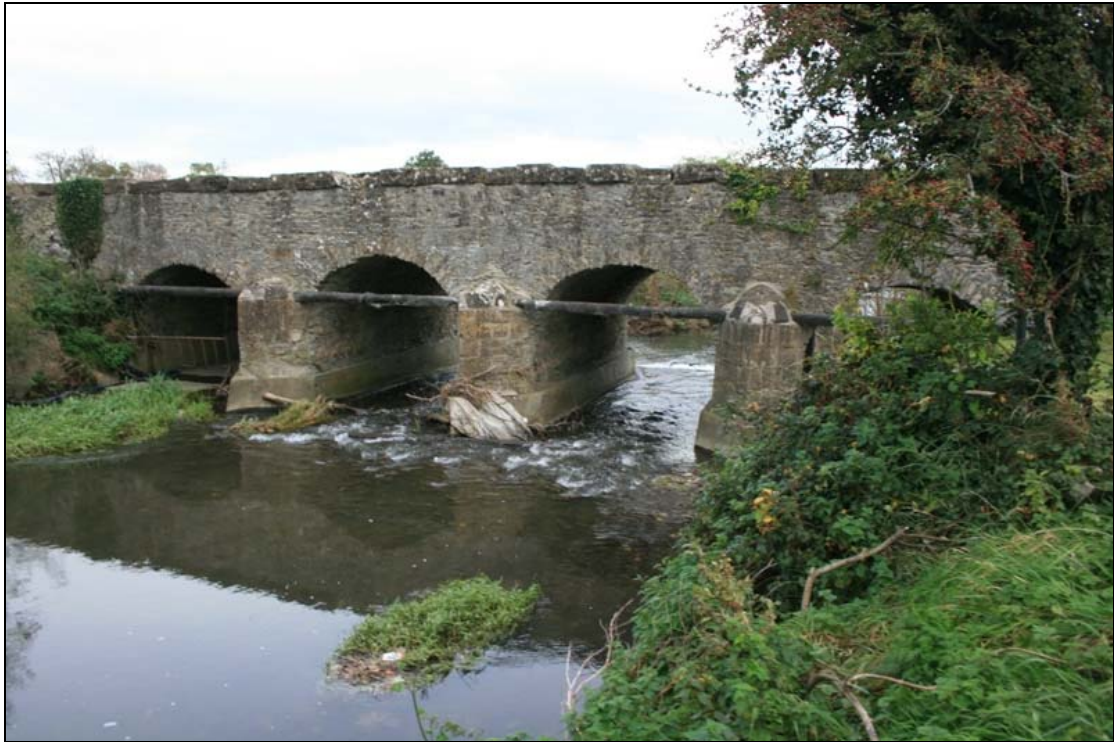
FHBS-08-BH-01 ~ West upstream elevation
