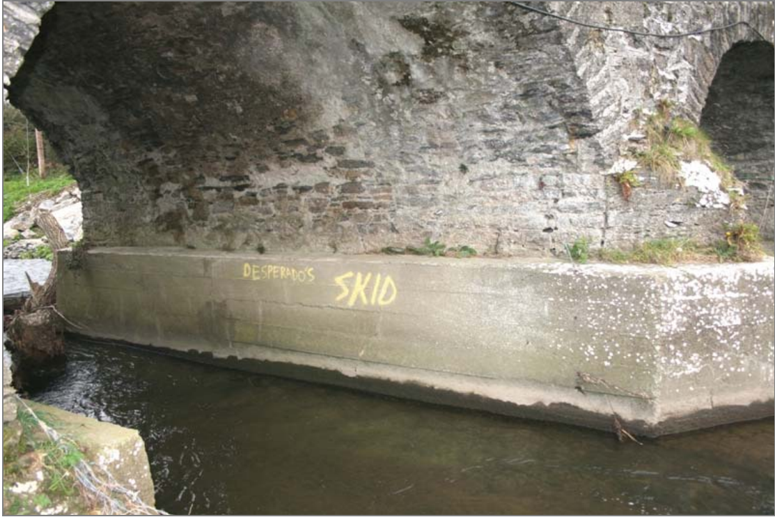
FHBS-07-BH-07 ~ Southern archway from east
