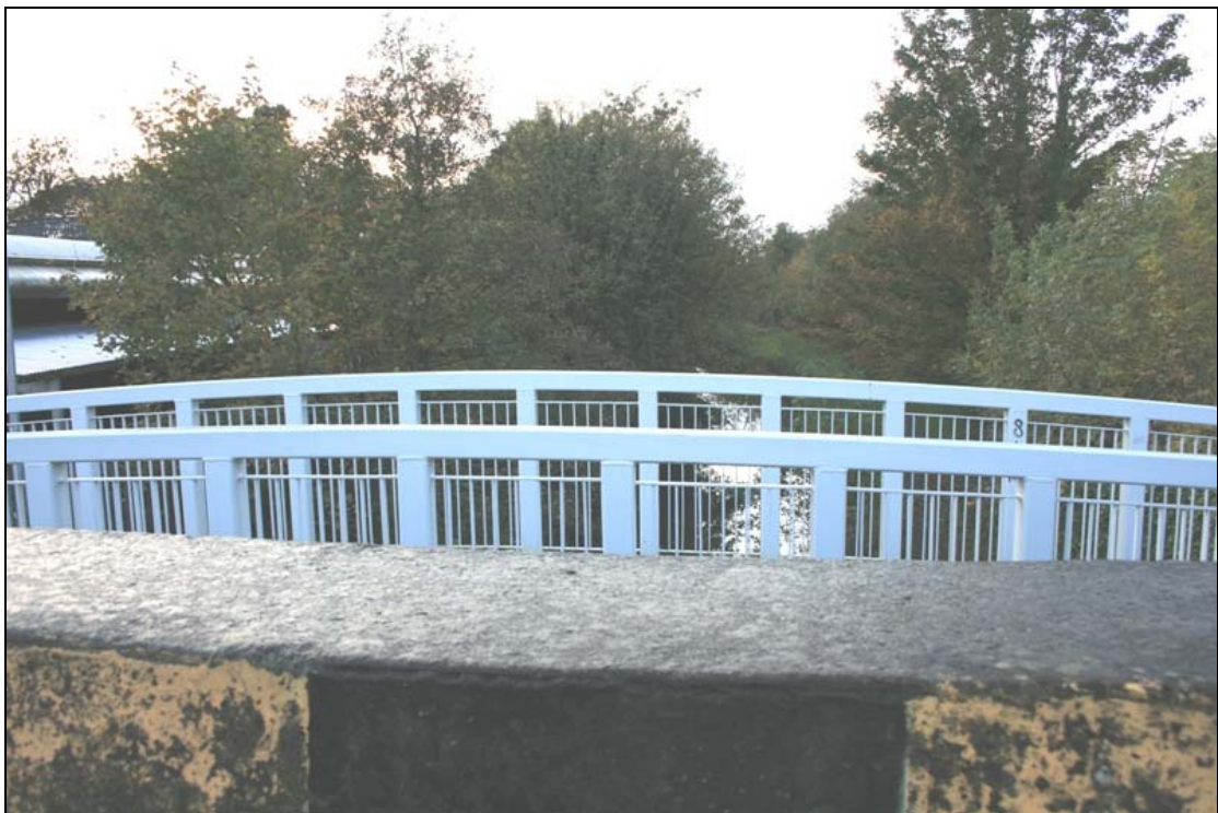
FHBS-14-BH-08 ~ View over road and foot-bridge parapets to west
