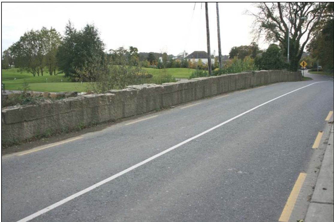
FHBS-08-BH-04 ~ East parapet from road
