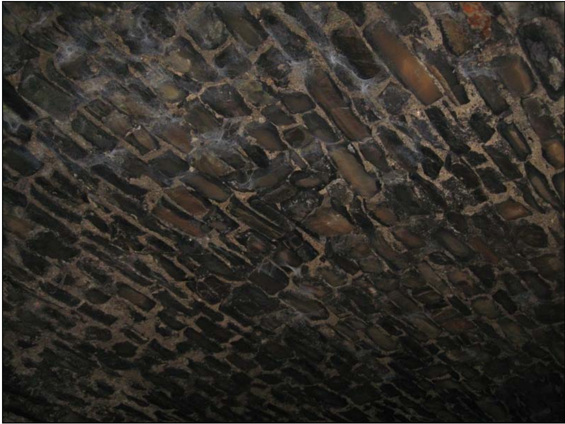
FHBS-14-NH-01 ~ Bridge underarch
