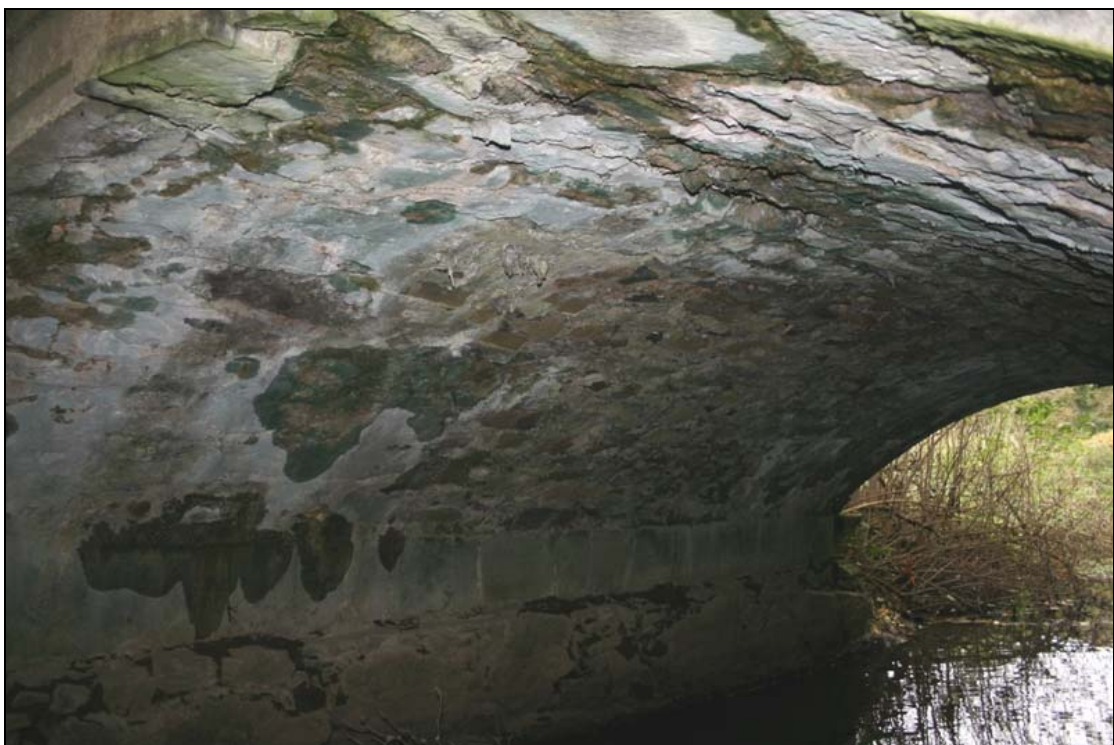
FHBS-09-BH-07 ~ Soffit of arch from west
