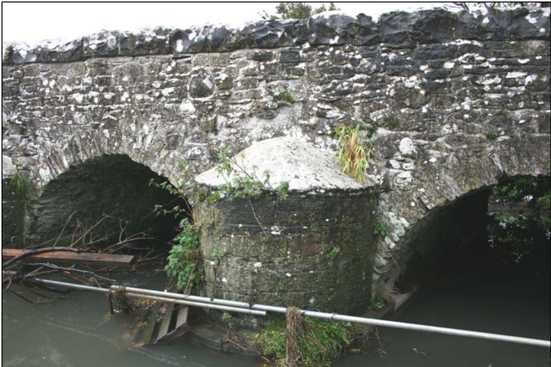
FHBS-12-BH-07 ~ Round cutwater between southern and central arch from west
