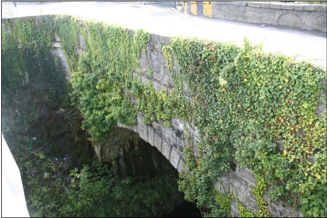
FHBS-13-NH-03 ~ Ivy coverage near bridge underarch
