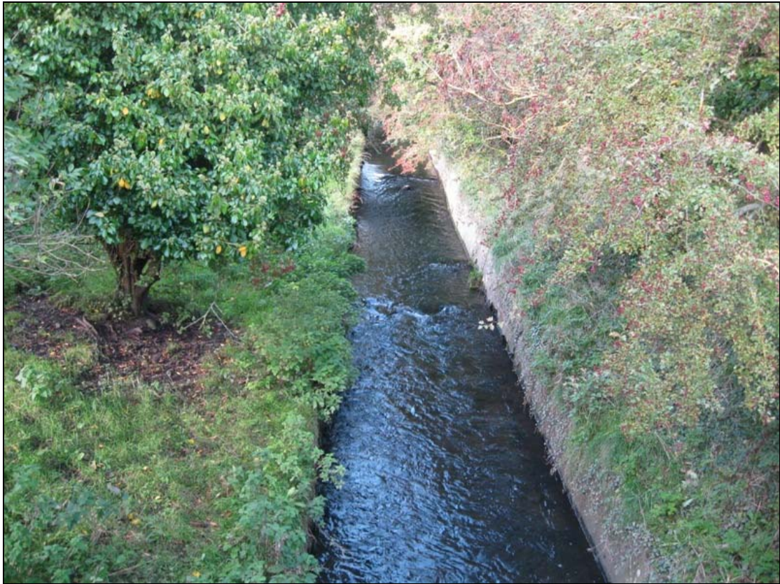
FHBS-04-NH-01 ~ Channelised stream flowing under bridge
