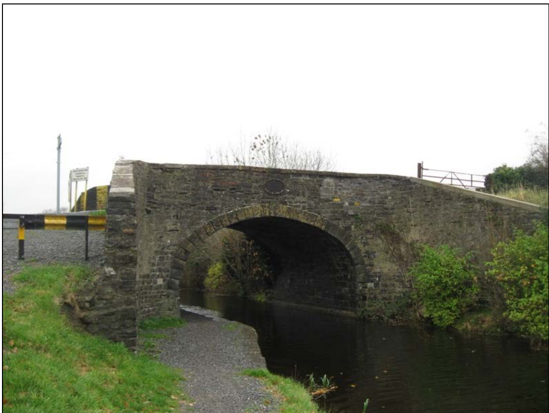
FHBS-15-NH-04 ~ Upstream side of bridge structure
