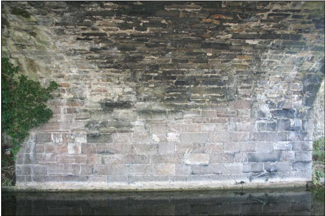
FHBS-15-BH-07 ~ South side of canal bridge arch soffit
