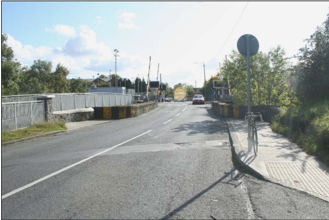
FHBS-13-BH-07 ~ View south over Kirkpatrick bridge and adjacent railway level crossing
