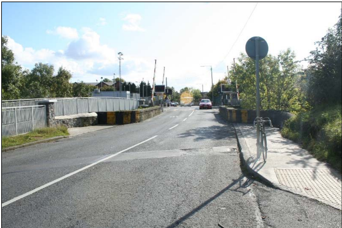
FHBS-13-NH-02 ~ Bridge walls - nearby railway crossing
