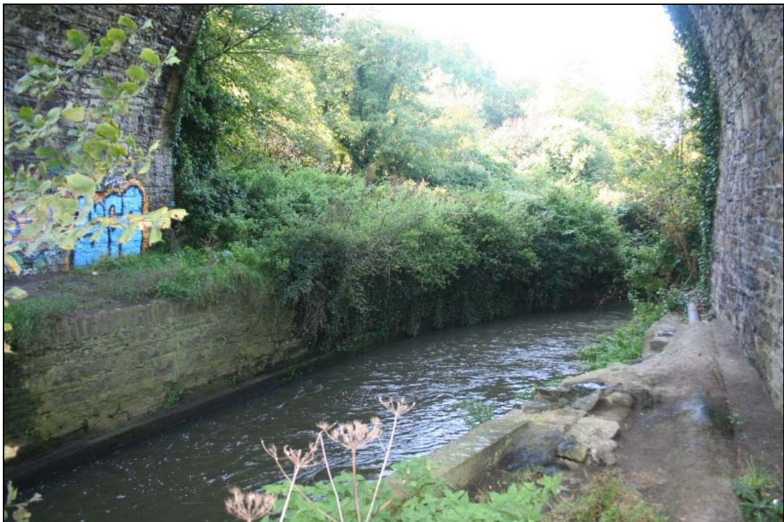
FHBS-11-BH-13 ~ View upstream through arch
