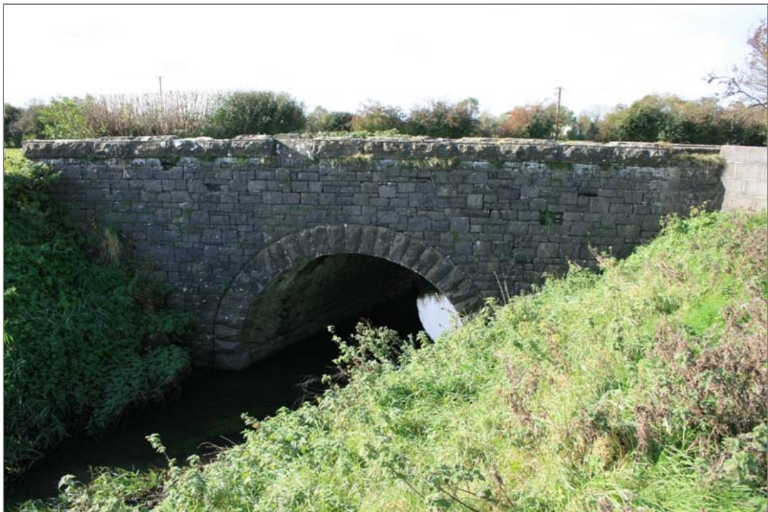
FHBS-03-BH-02 ~ East downstream elevation
