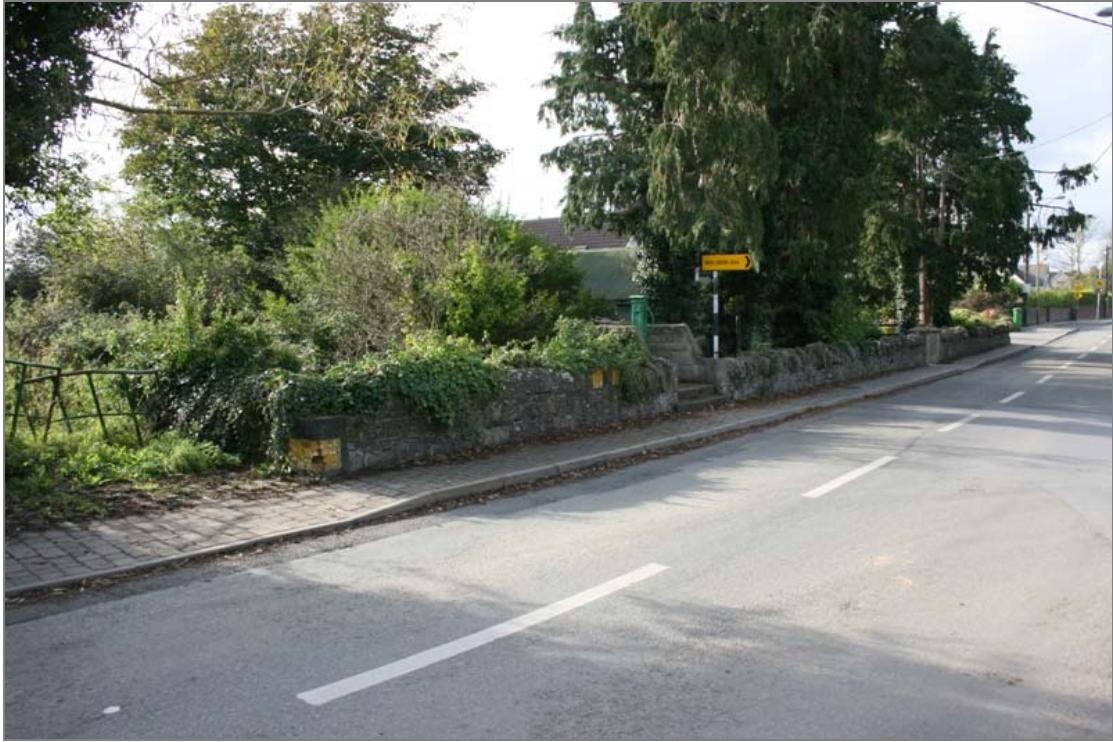
FHBS-05-BH-03 ~ South parapet from road
