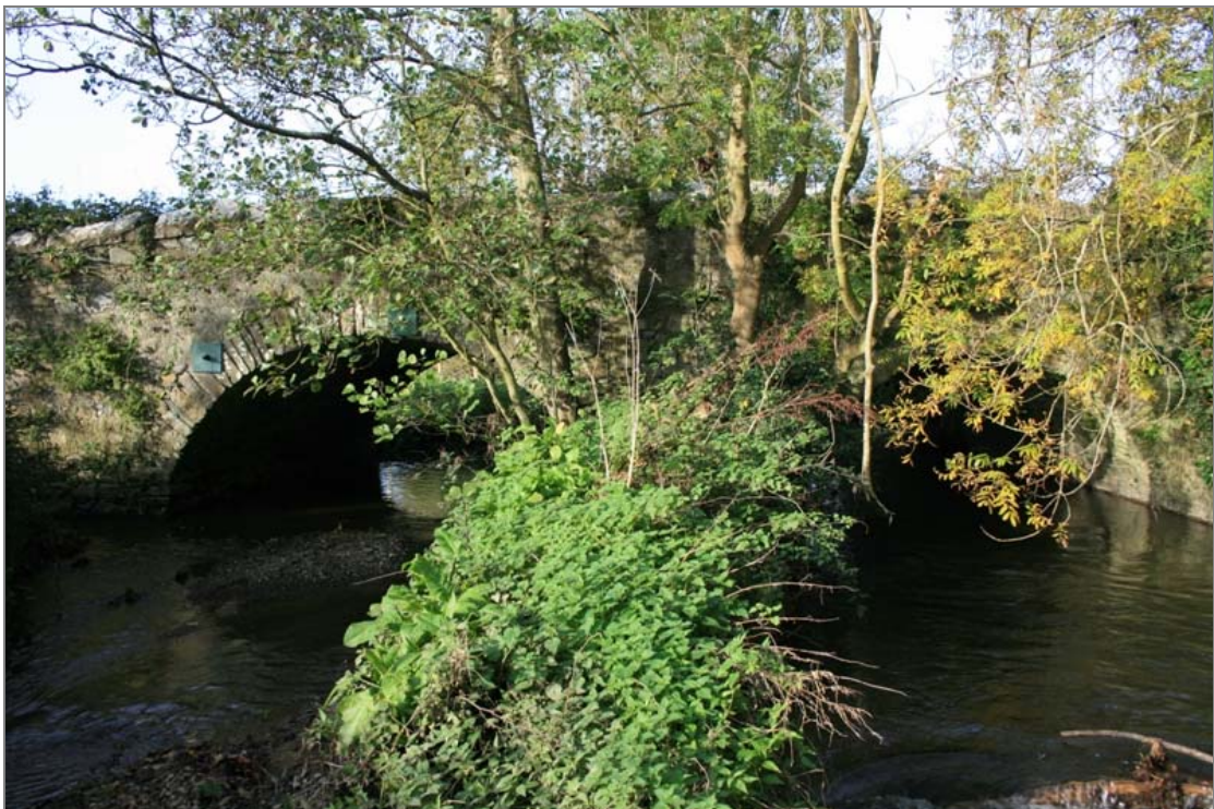
FHBS-01-BH-02 ~ East downstream elevation
