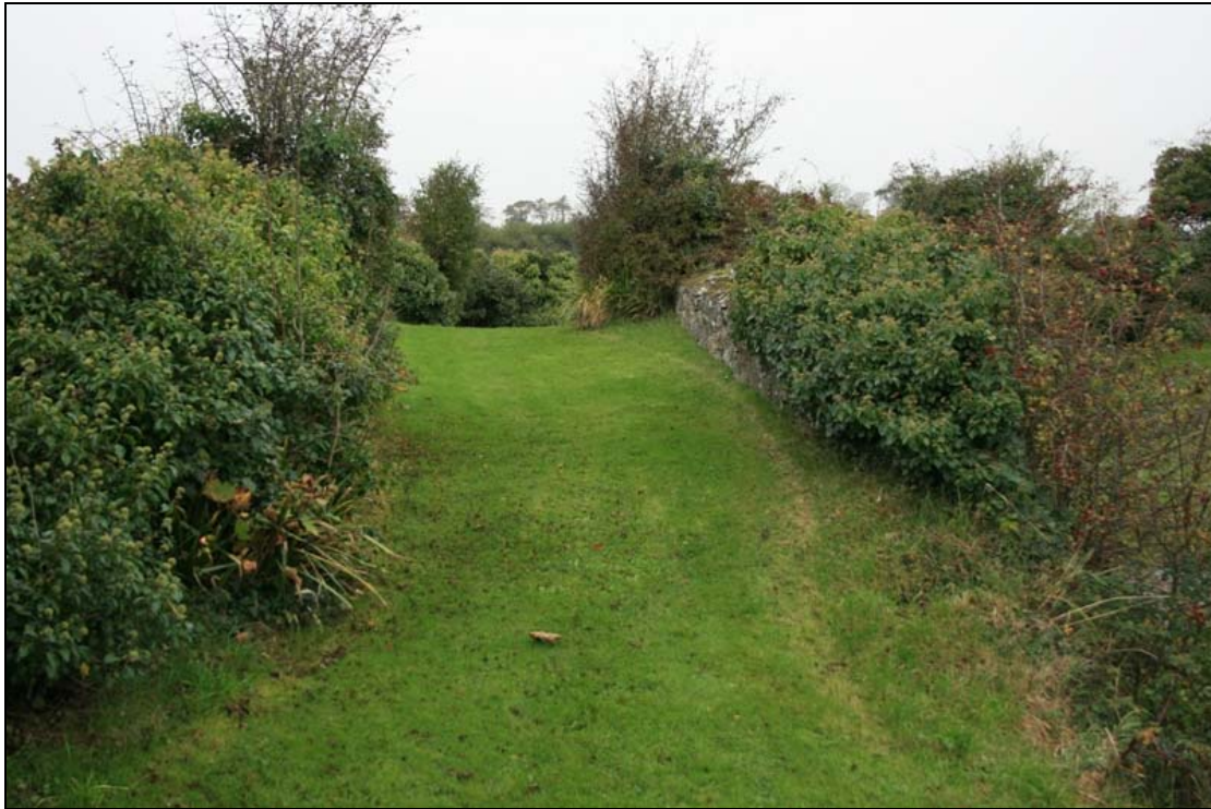
FHBS-10-BH-08 ~ View west over bridge
