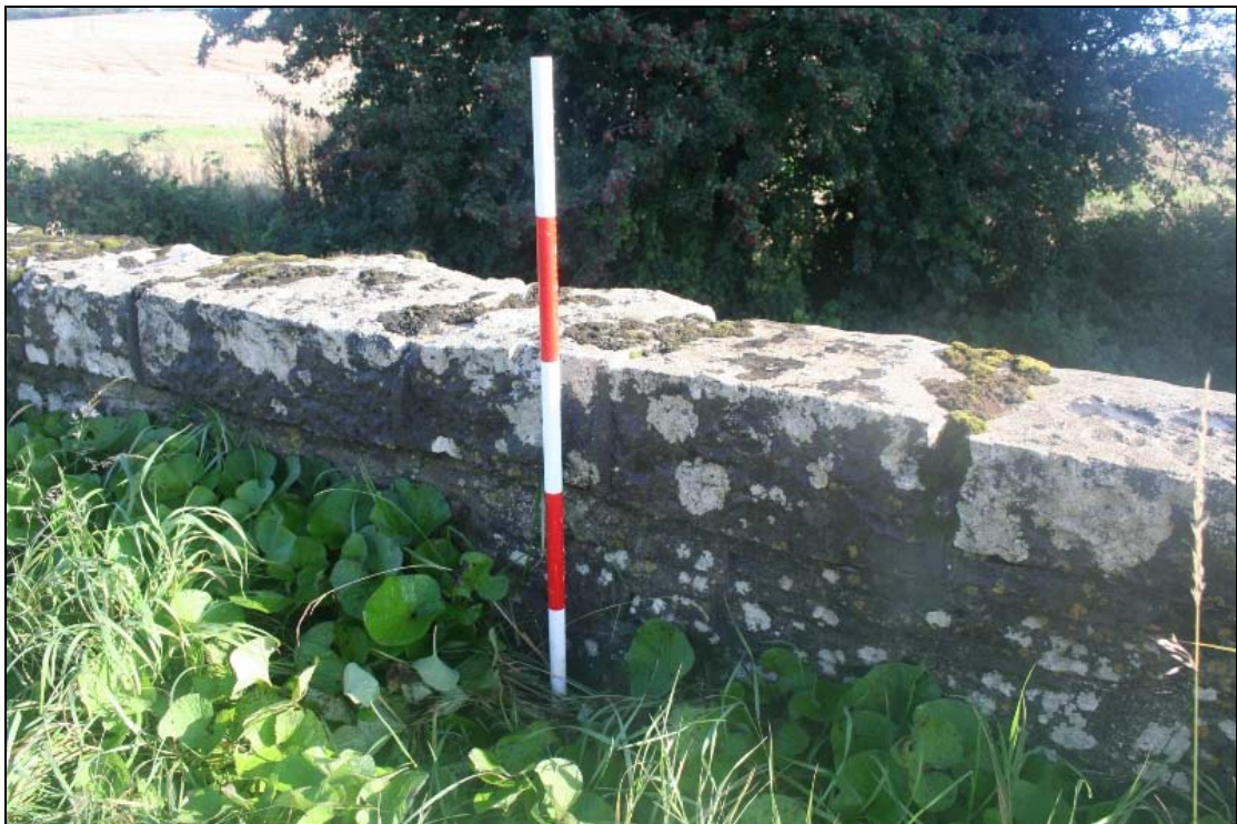
FHBS-12-BH-04 ~ East parapet from road
