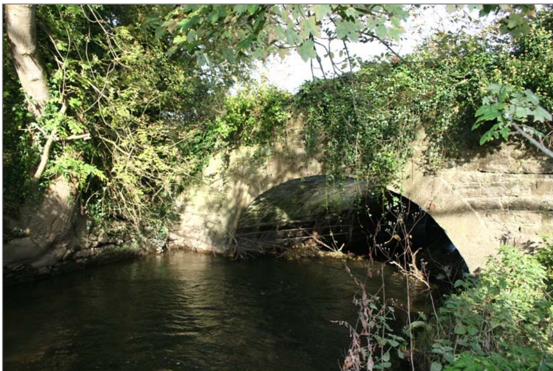
FHBS-02-BH-01 ~ South upstream elevation
