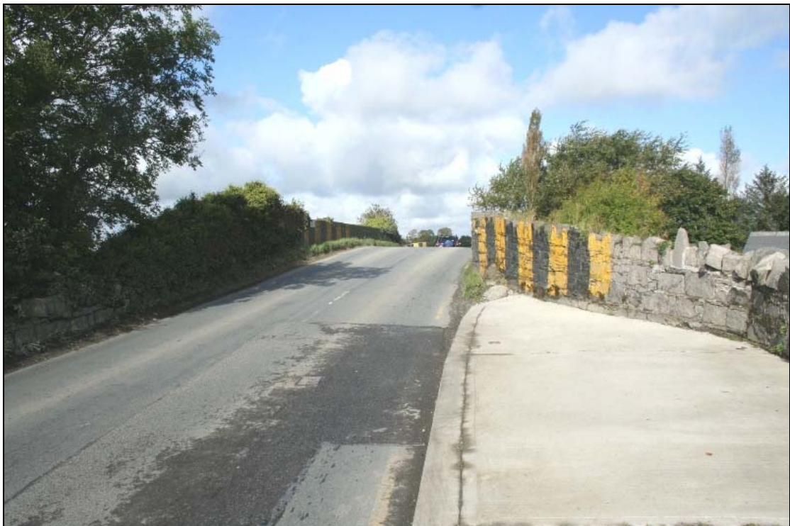
FHBS-15-BH-15 ~ View north over rail bridge)
