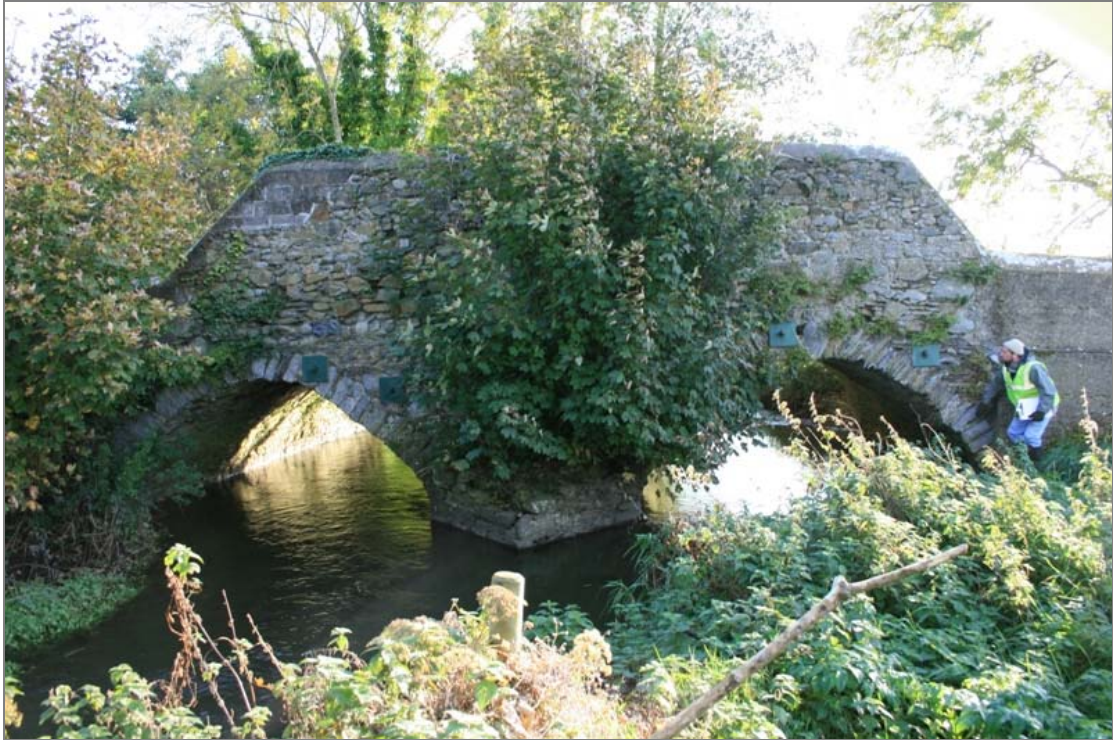
FHBS-01-BH-01 ~ West upstream elevation
