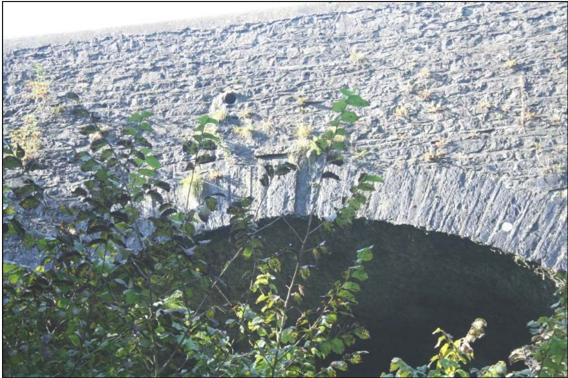
FHBS-11-BH-02 ~ East parapet from east showing road drainage pipe and keystone
