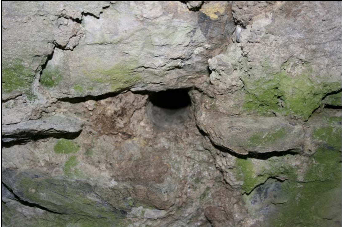
FHBS-08-NH-01 ~ Circular opening in bridge underarch
