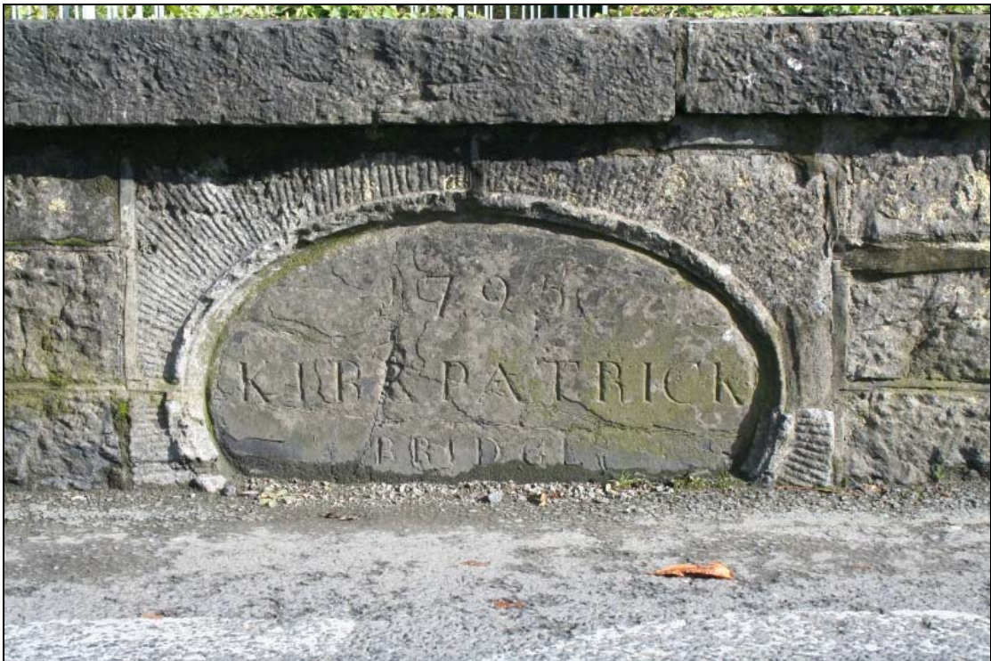
FHBS-13-BH-06 ~ Name plaque on road side of west parapet
