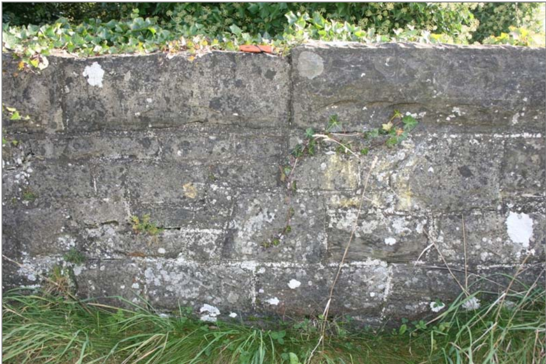
FHBS-04-BH-03 ~ West parapet from road
