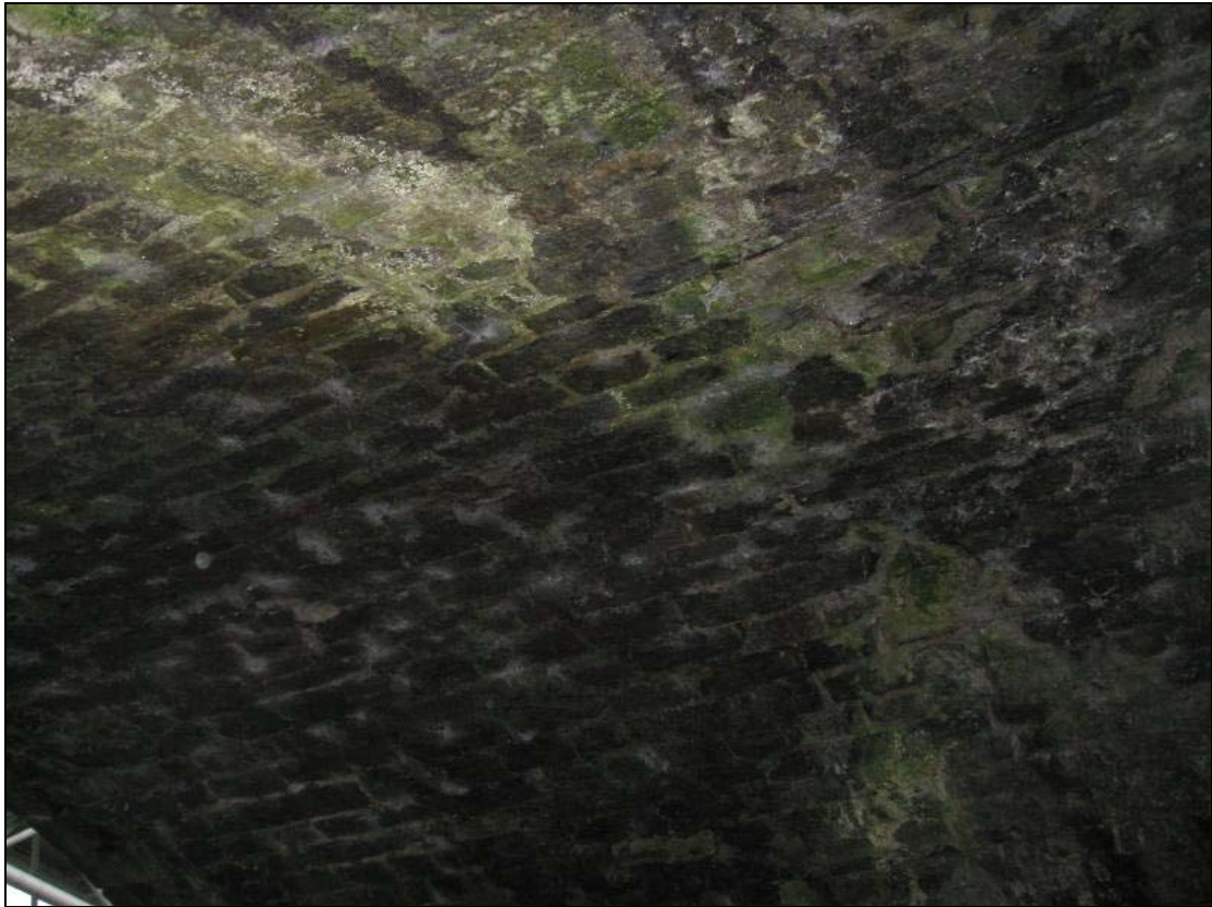
FHBS-13-NH-01 ~ Bridge underarch - lack of crevices
