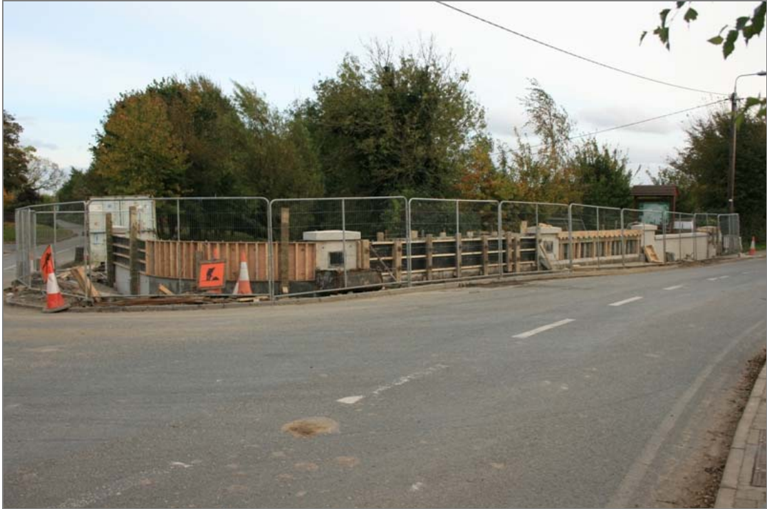
FHBS-06-BH-04 ~ East parapet from road
