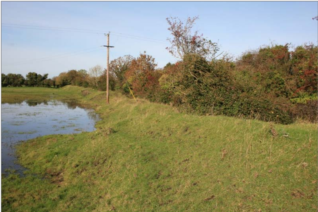
FHBS-04-BH-08 ~ View upstream to west
