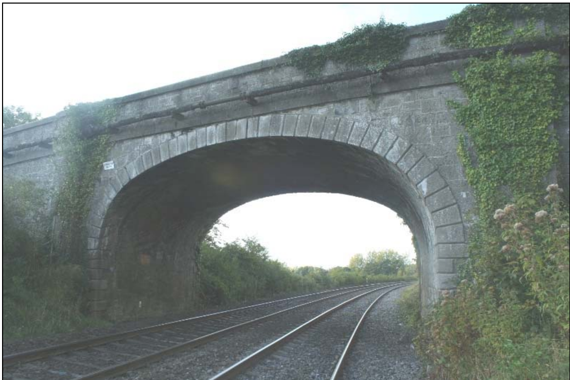
FHBS-15-BH-12 ~ East elevation of rail bridge
