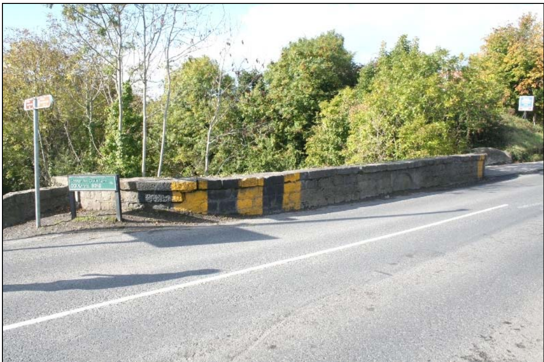
FHBS-13-BH-04 ~ West parapet from road looking north west
