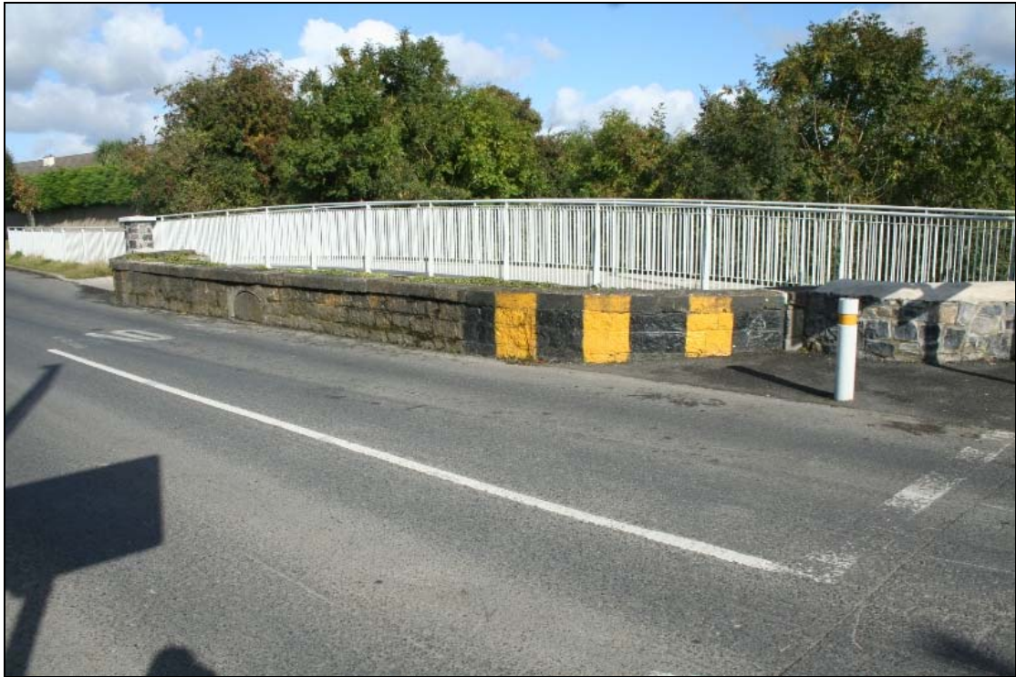
FHBS-13-BH-03 ~ East parapet from road looking north east
