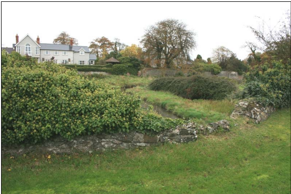
FHBS-10-BH-07 ~ View downstream to north from west abutment
