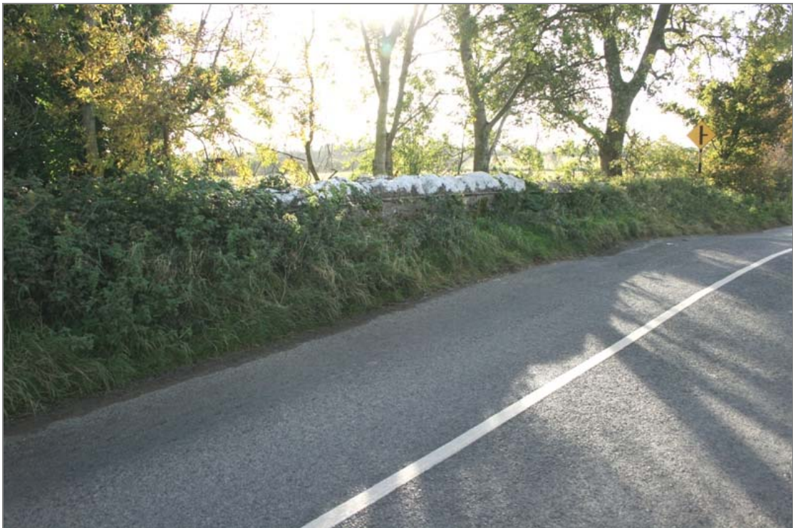
FHBS-01-BH-04 ~ East parapet from road
