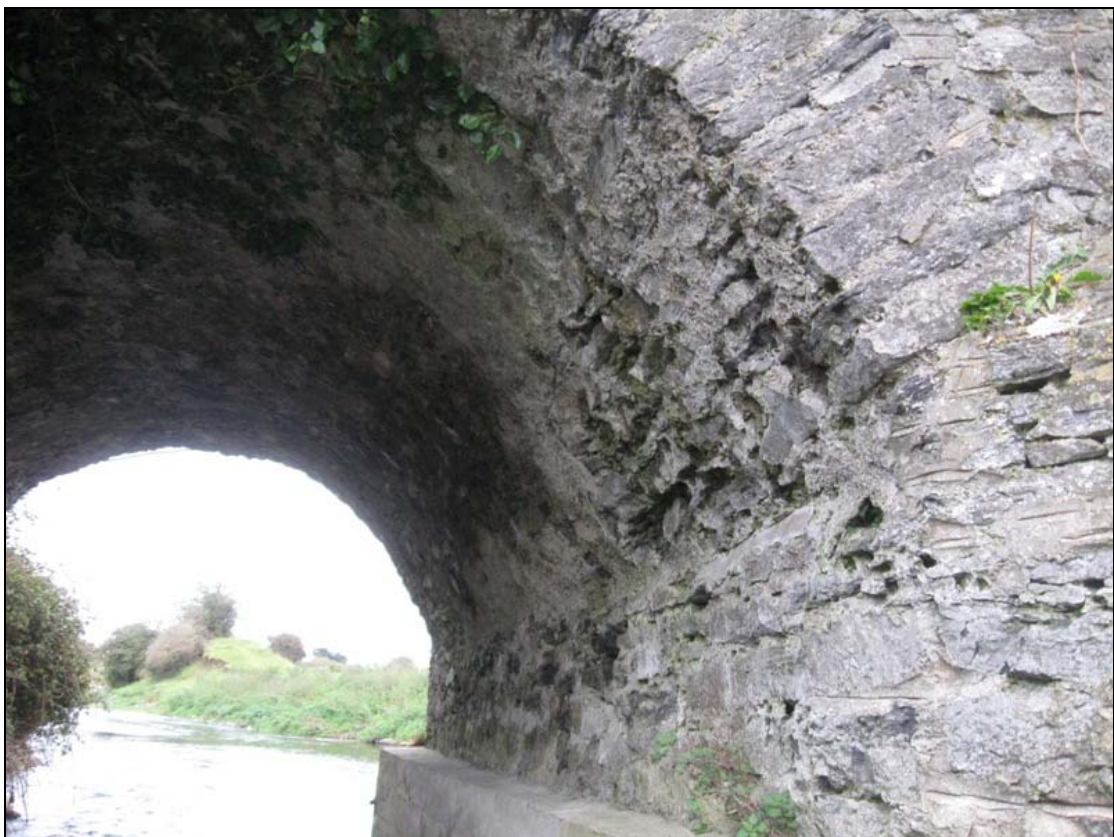
FHBS-07-NH-04 ~ Underarch of bridge
