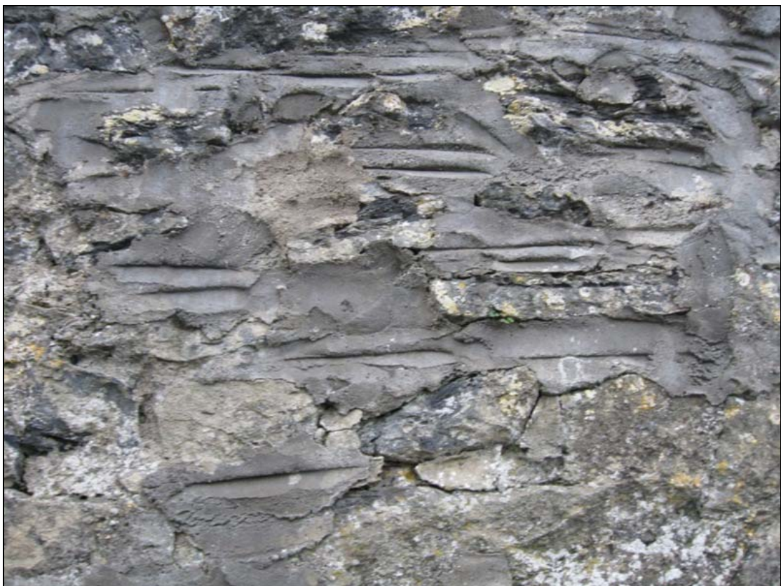
FHBS-08-NH-04 ~ Repointed parapet wall
