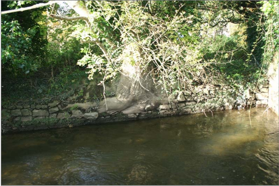
FHBS-02-BH-04 ~ Large Ash tree rooted on stone-built west bank just upstream of south elevation
