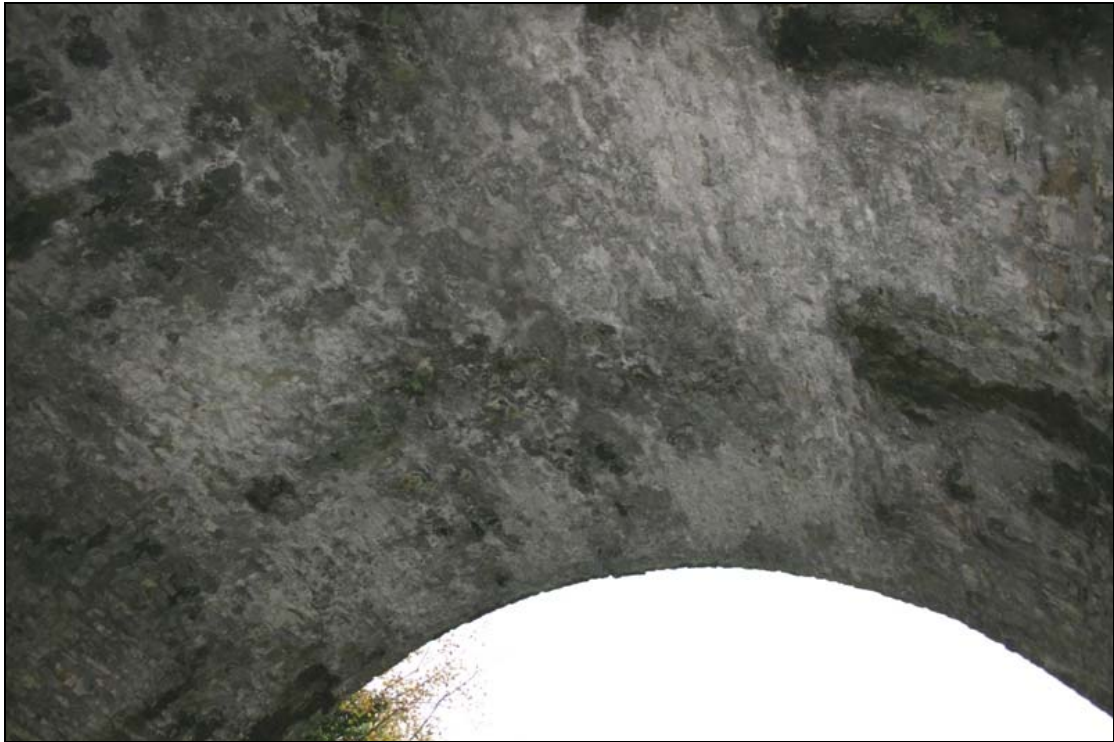
FHBS-11-BH-12 ~ Soffit of arch at western side
