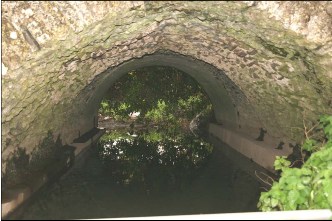
FHBS-12-BH-06 ~ Soffit of southern arch from west
