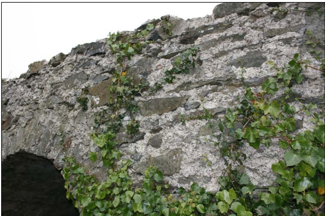
FHBS-10-NH-02 ~ Bridge Parapet - restricted bat potential
