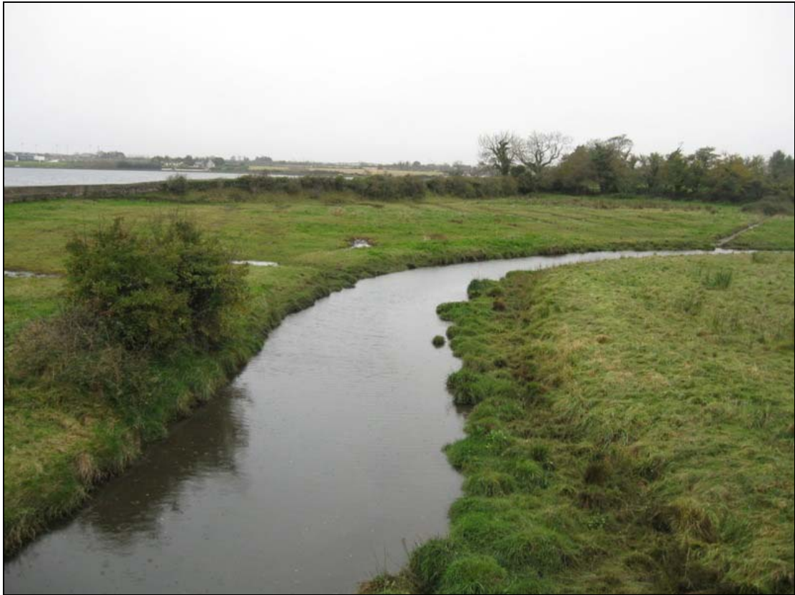
FHBS-10-NH-01 ~ Adjacent habitats upstream of the bridge structure
